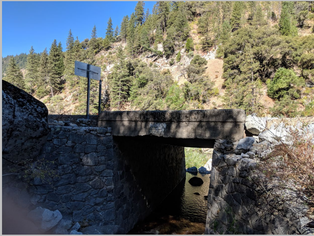
Appx. Figure 3. Existing Bear Creek Bridge
