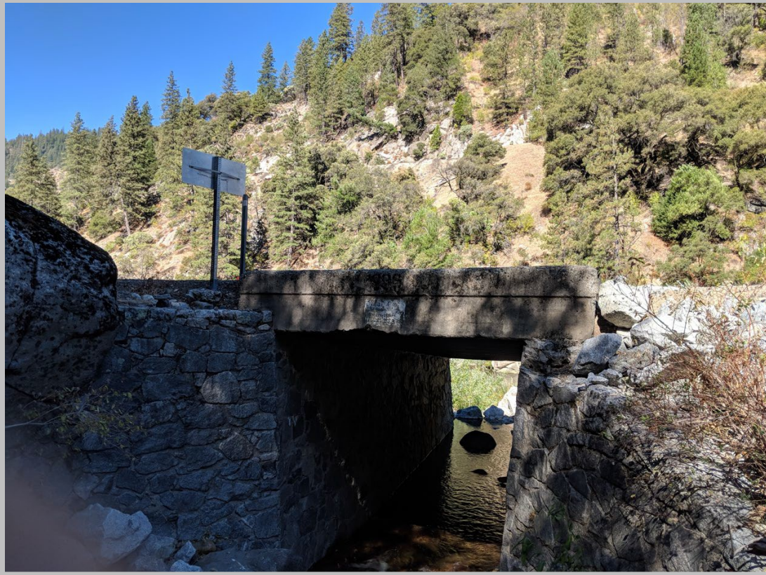
Appx. Figure 3. Existing Bear Creek Bridge
