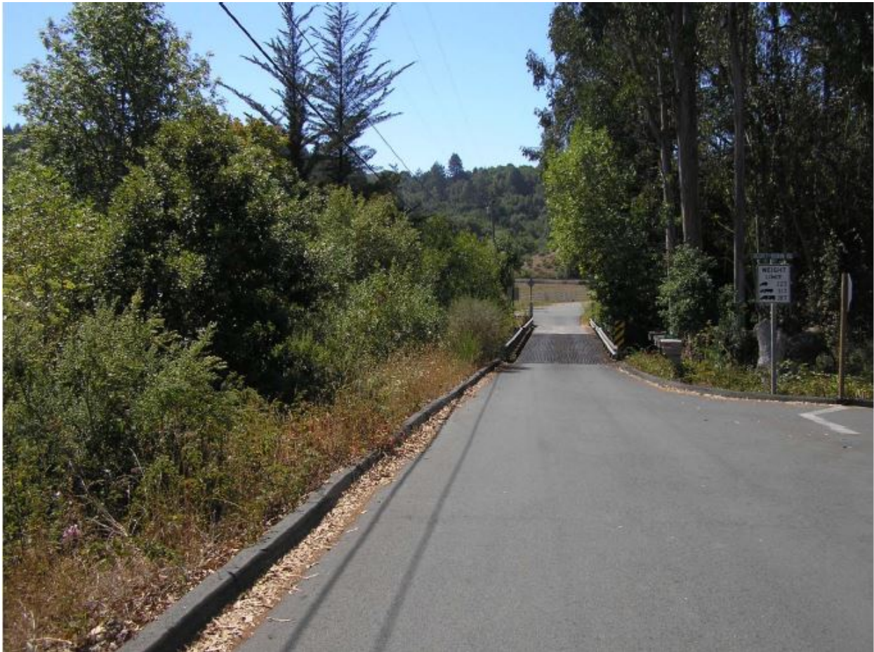
Figure 7 View of Freestone Flat Road at Scott Robin Road Looking Southwest
