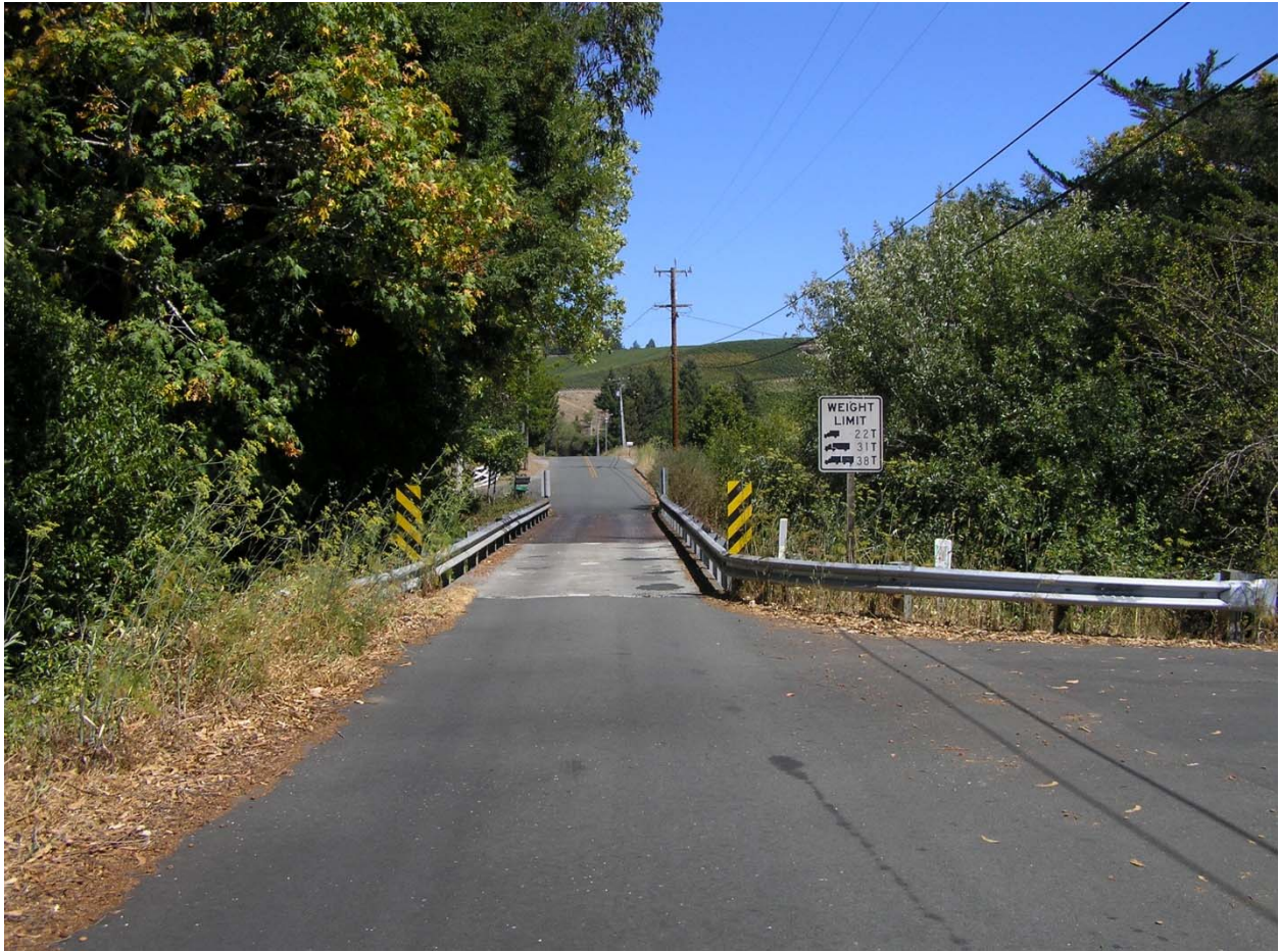
Figure 8 View of Freestone Flat Road Looking Northeast
