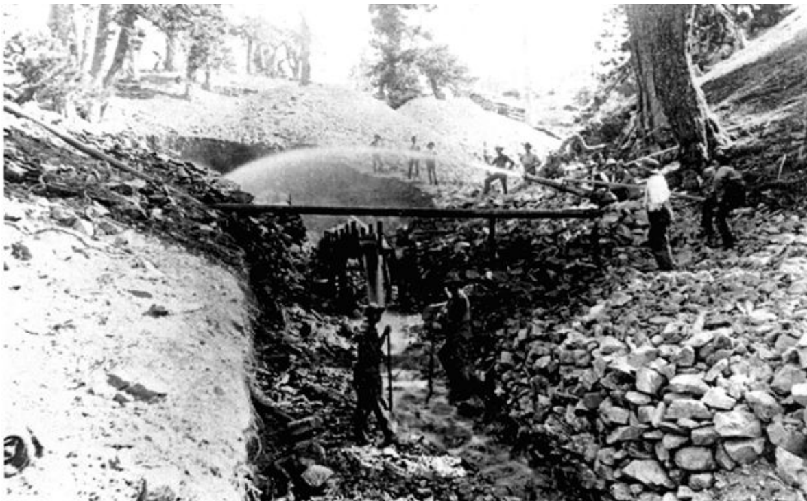
Figure 3.3-2. Hydraulic mining, n.d. Courtesy California Gold Mines, A Sesquicentennial Photograph Collection, California Department of Mines and Geology.
