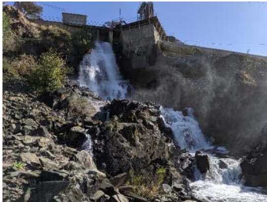
Eastern canyon walls looking up sluice channel. Shows steepness and limited line of sight.
