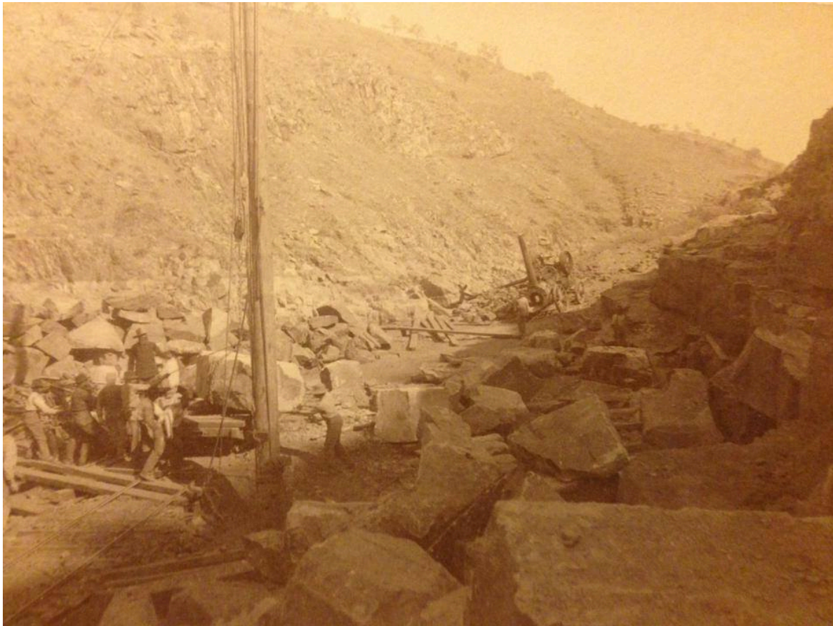
Figure 3.3-6. Early construction of La Grange Diversion Dam, n.d. Courtesy of La Grange Museum.
