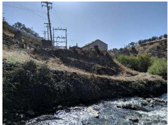
Existing dirt road which would be used to access channel and diversion structure installation area. All soils are previously compacted and/or very rocky. Few burrows/refugia observed.
