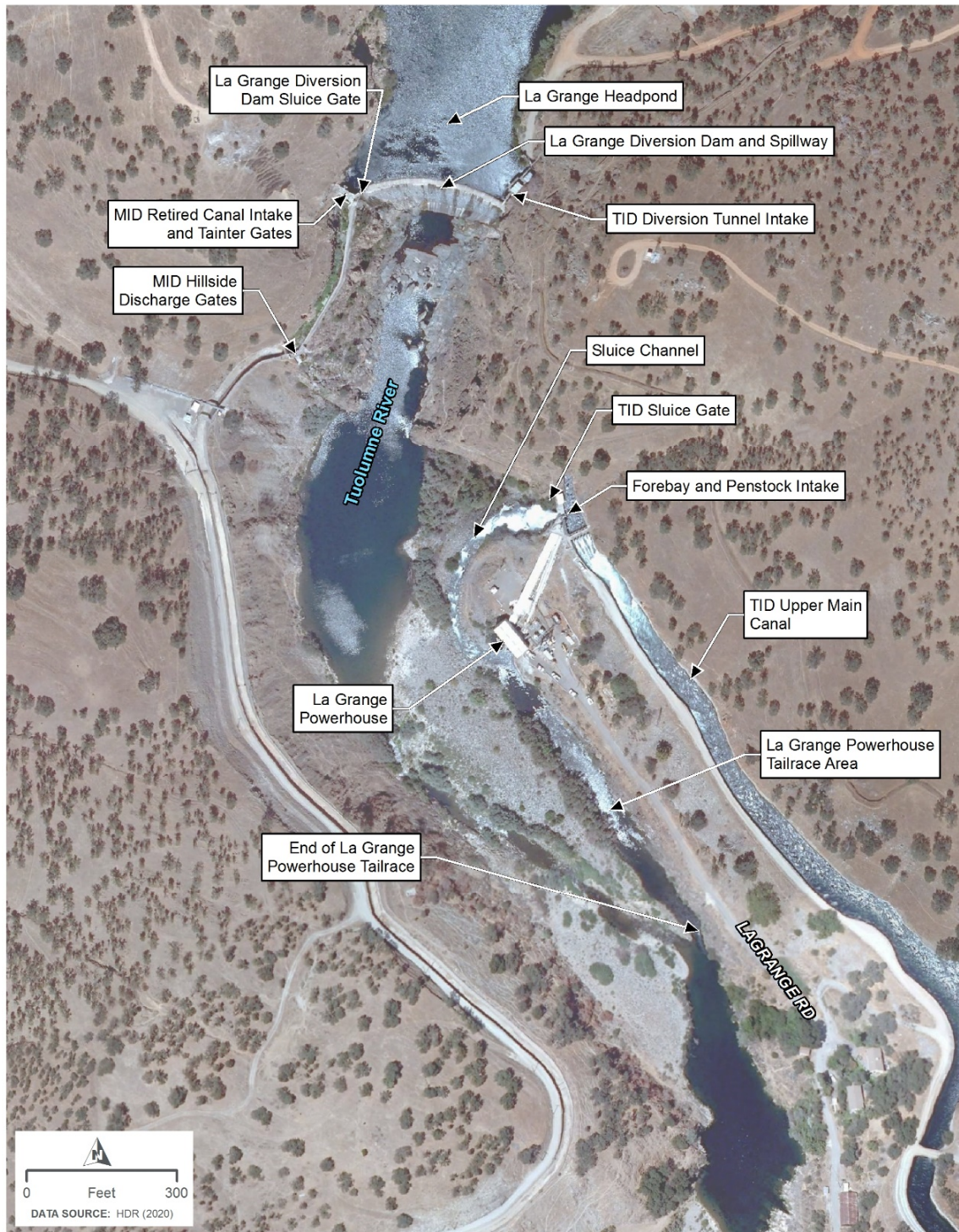
Figure 1. Infrastructure associated with the La Grange Diversion Dam
