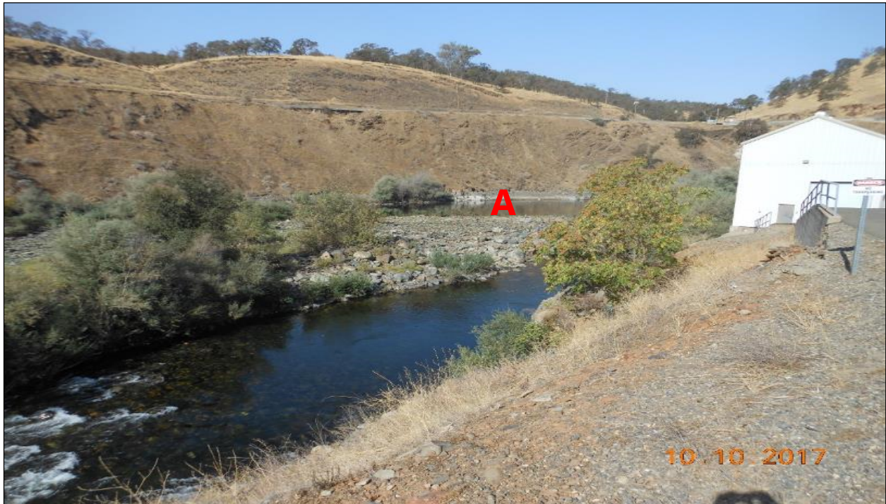
Figure 7. Upstream topographic high between river and tailrace channel
