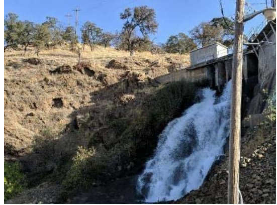
Steep cliff north of sluice channel. Another barrier to potential California tiger salamander movement.
