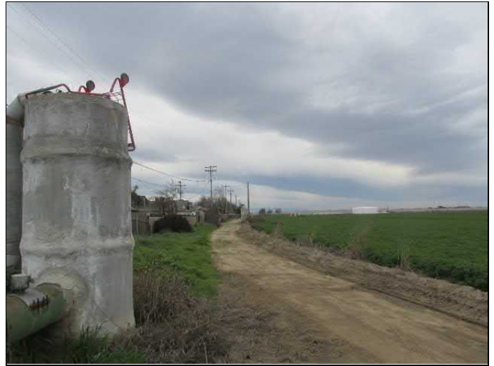
20. View of the concrete standpipe and the southern portion of the subject property.
