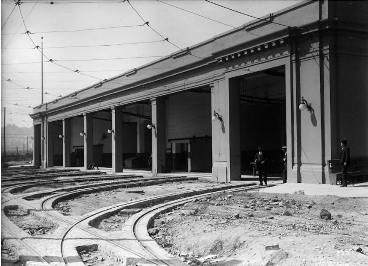
Figure 76. Potrero Car Barn under construction, 1915.
