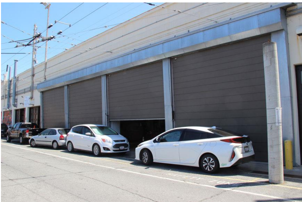
Figure 51. Contemporary overhead doors on west façade, looking northeast from bus yard.
