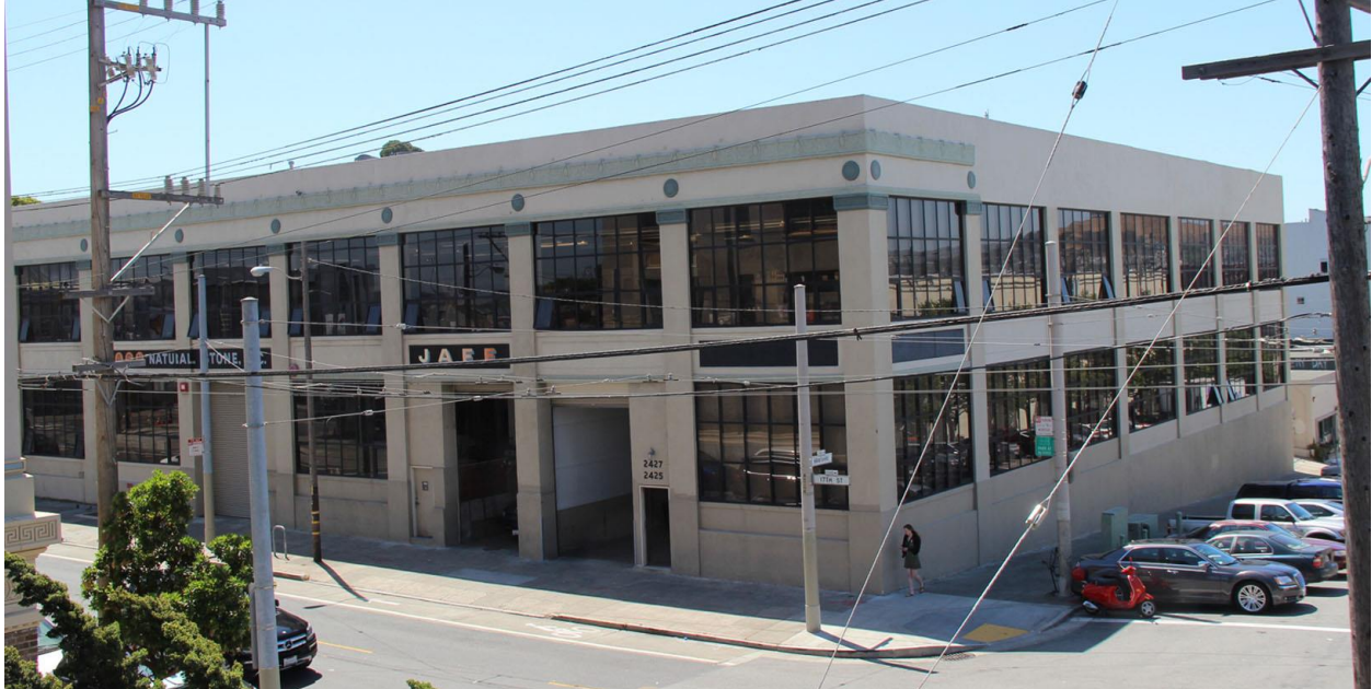
Figure 20. Leyser-Green Co. Building at 2401-25 17 th Street, looking southeast from 17 th Street.
