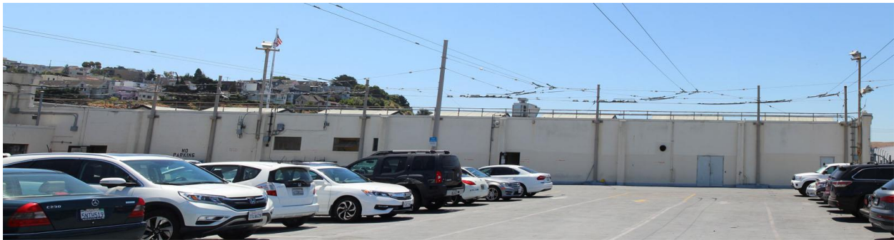
Figure 46. North façade of second floor office wing, looking south from parking deck.
