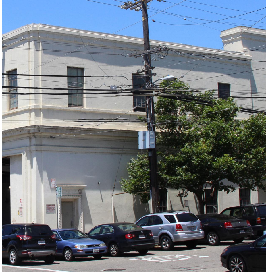
Figure 41. Southernmost section of secondary façade facing Hampshire Street, looking northwest.
