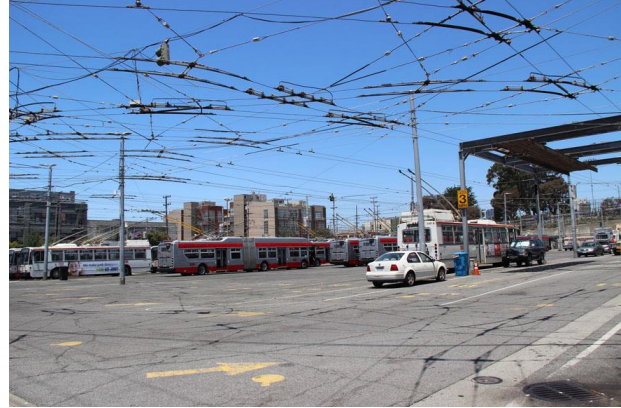
Figure 25. Entrance to bus yard, looking northwest.
