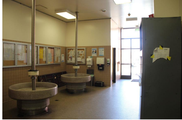
Figure 58. Hand wash station near toilet rooms on west side of first floor level, looking west.
