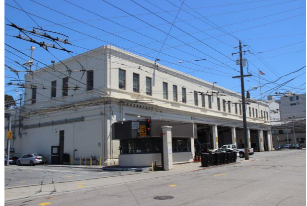
Figure 29. Paved setback and control tower in front of maintenance/operations building, looking northeast.
