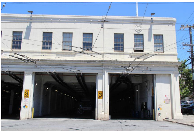
Figure 37. Easternmost bays of primary façade, looking north.
