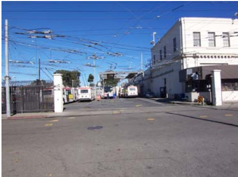
100_5702.JPG, 11/20/2007, view to N
