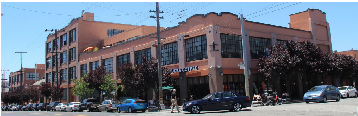
Figure 8. Former Best Foods plant at 1900 Bryant Street, looking southwest.
