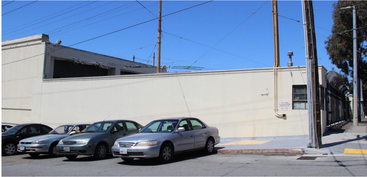
Figure 43. Northern section of secondary façade, looking southwest from Hampshire and 17 th Streets.
