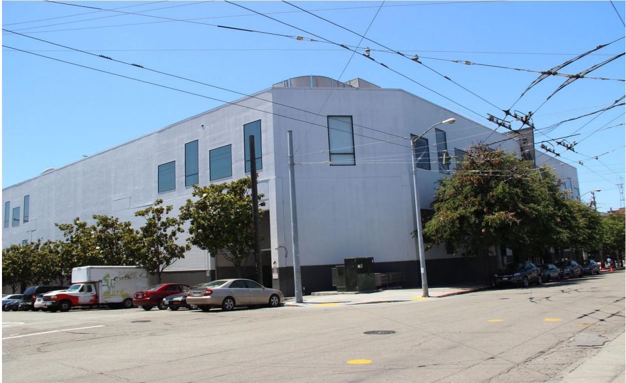
Figure 7. KQED studios at 1901 Bryant Street, looking southwest.
