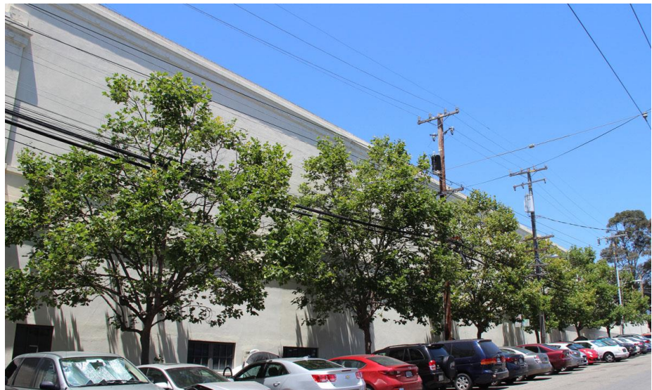
Figure 42. Middle section of secondary façade, looking northwest.
