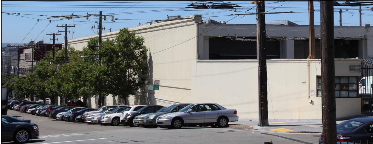
Figure 3: SFMTA Potrero Trolley Coach Division Facility, view northwest of east elevation facing Hampshire Street, (photo courtesy of HRE Part 1). The end of the shops wing is visible here along Hampshire Street at the intersection of Hampshire and 17 th Street.
