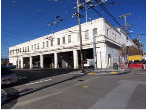
100_5706.JPG, 11/20/2007, view to SW
