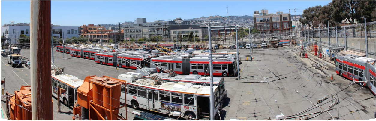
Figure 22. Mariposa Bus Yard, looking southwest.
