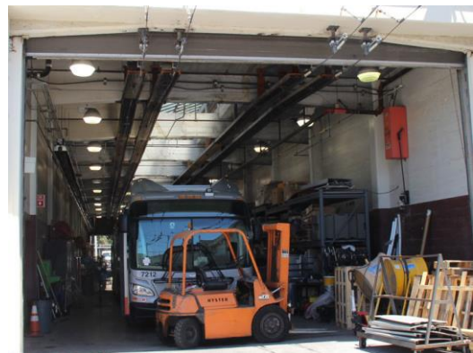
Figure 61. Second floor maintenance shop, looking north.
