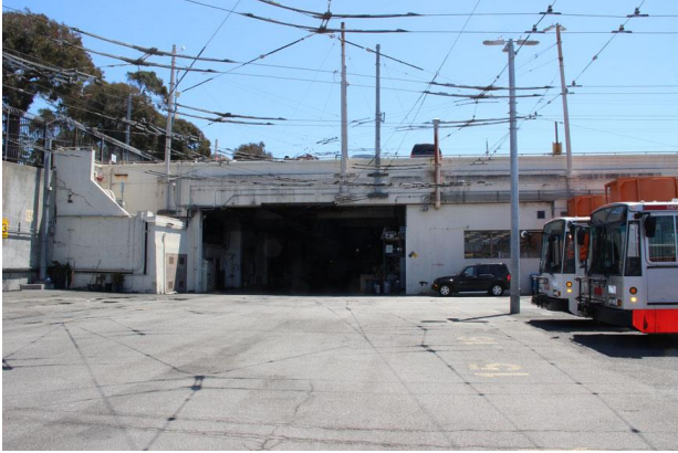
Figure 49. Vehicular entrance at north end of west façade, looking east from bus yard.
