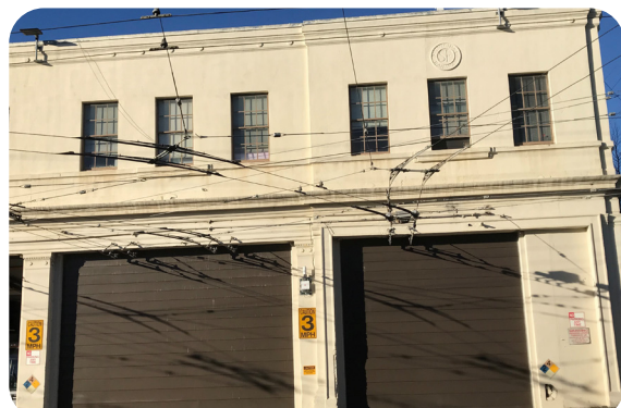
Image 9: Detail view of office wing primary façade. Note character-defining features include large vehicular openings, double-hung windows, and medallion featuring original Muni logo.
