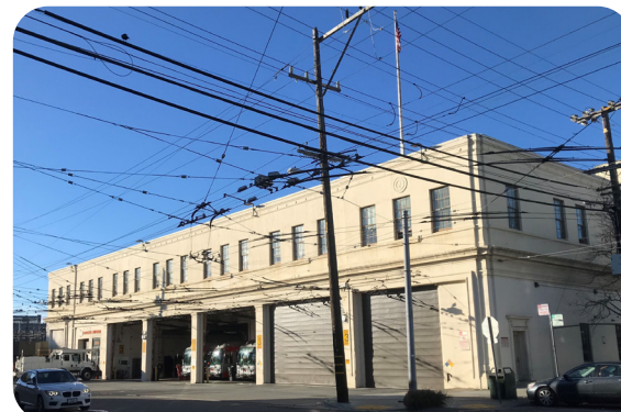
Image 10: Detail view of office wing's primary (Mariposa Street) and secondary façades (Hampshire Street). Note character-defining features include the fenestration pattern of groups of three double-hung metal windows at the second floor level with a continuous lug sill, large vehicular openings at the first floor, reentrant corner detailing, and the flagpole.
