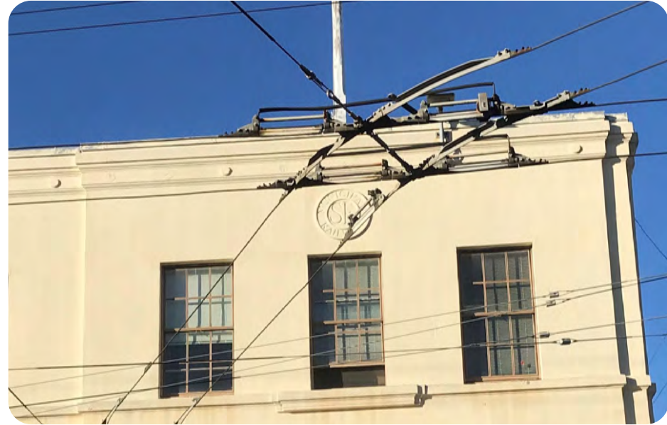
Image 6: Detail view of office wing primary façade. Note character defining features including molded concrete and cement plaster ornament, fenestration pattern of groups of three double-hung metal windows, medallion featuring original Muni logo, and flagpole
