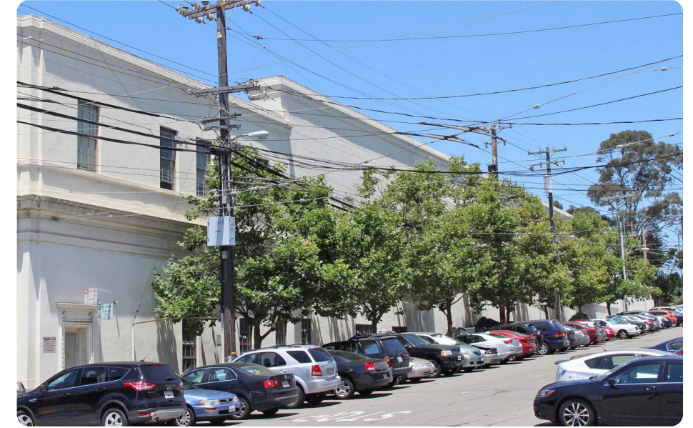
Image 3: View northwest of secondary façade along Hampshire Street. Note the change in parapet height where the office wing (left) meets the shops wing (right).
