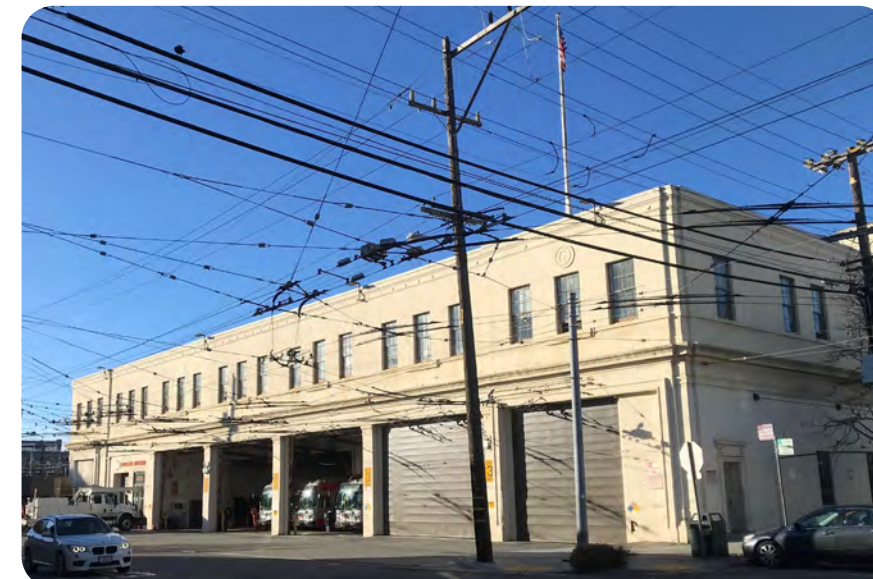
Image 10: Detail view of office wing's primary (Mariposa Street) and secondary (Hampshire Street) façades. Note character-defining features include the fenestration pattern of groups of three double-hung metal windows at the second floor level with a continuous lug sill, large vehicular openings at the first floor, reentrant corner detailing, and the flagpole.
