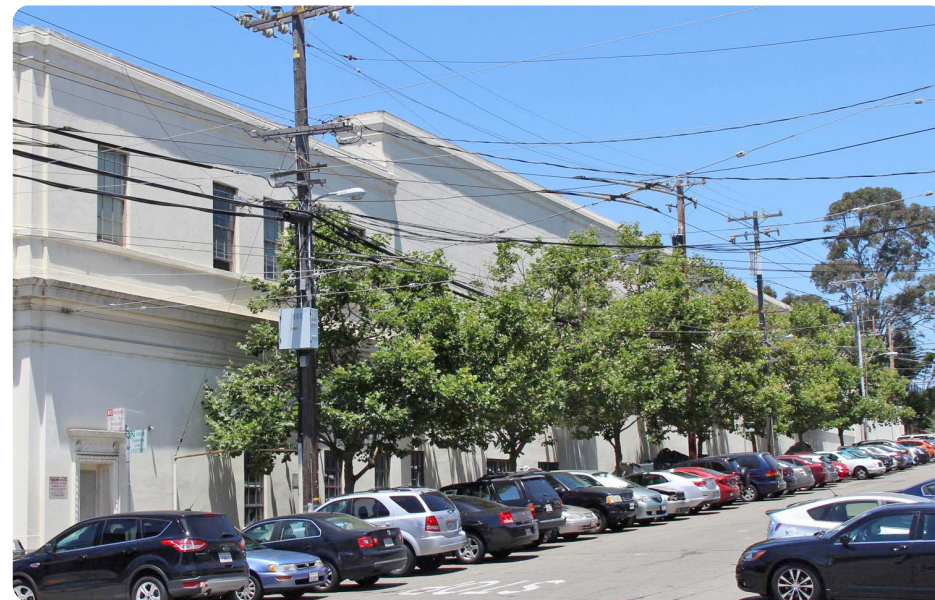
View B: Hampshire Street Looking North, Existing
