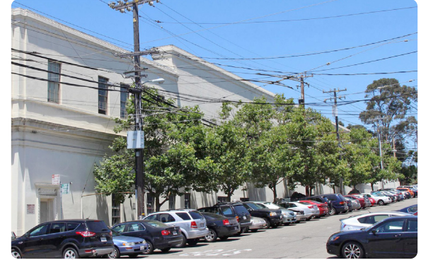
Image 3: View northwest of secondary façade along Hampshire Street. Note the change in parapet height where the office wing (left) meets the shops wing (right).
