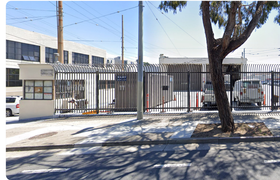
Image 5: View south of shops wing tertiary façade along 17th Street.
