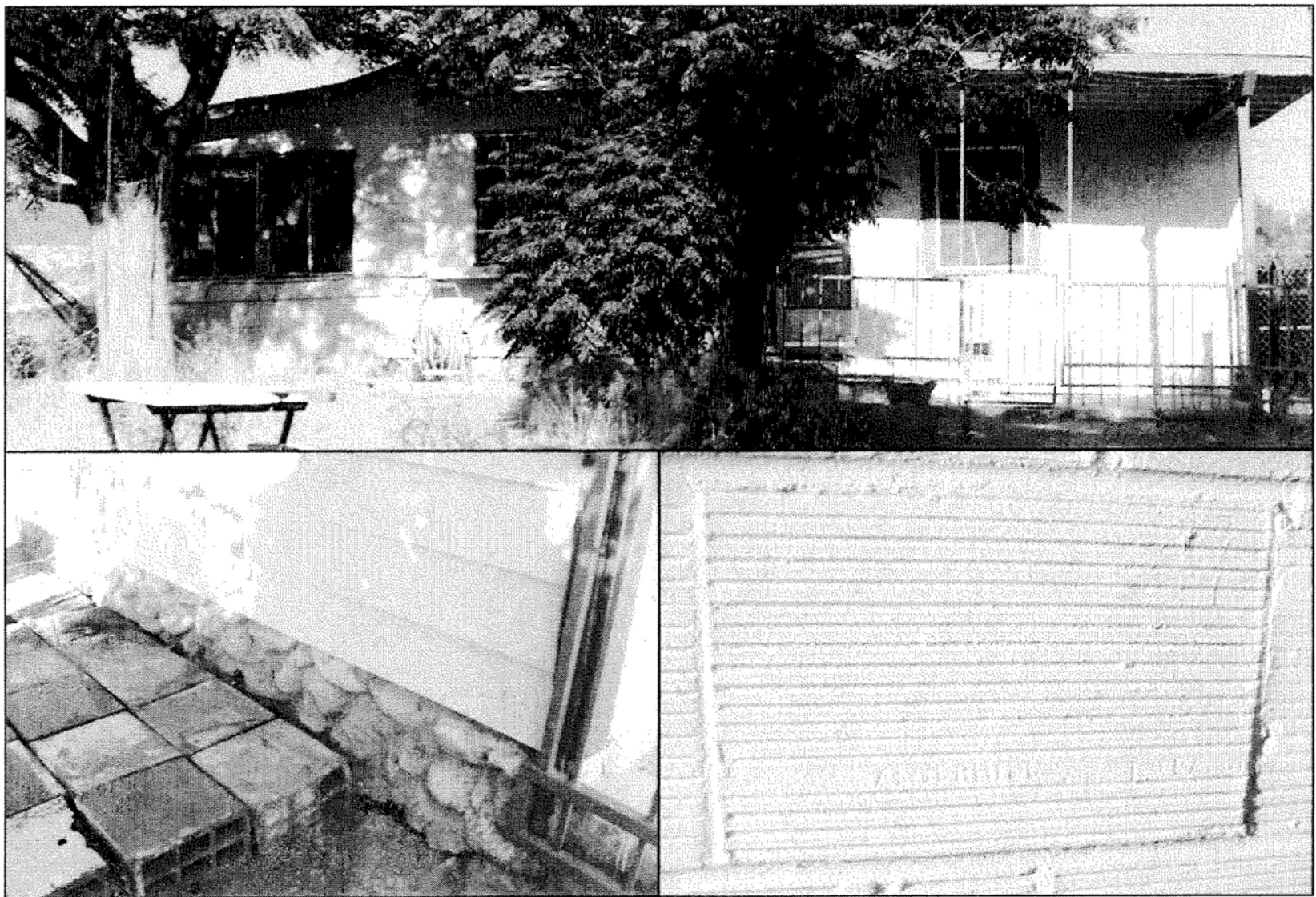
Figure 9. Historic-period residence at 28915 Lake Street. Clockwise from top: primary façade, view to the west; detail of "Alberhill LABCP Co" blocks; stone footing at the middle of the primary façade.
