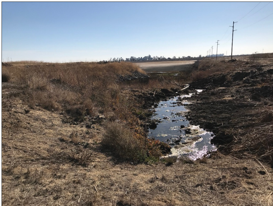
Photograph 7: Looking south is a view of the eastern detention basin proposed for the Wastewater Storage Reservoir and Floating Solar area. Note the wastewater currently draining into the detention basin.
