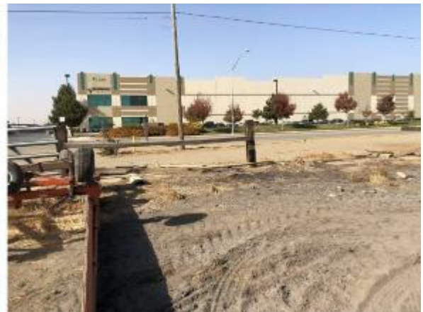
Photo #78 View of the UST tank location after cleanup and removal. Refer to Photo #54.
