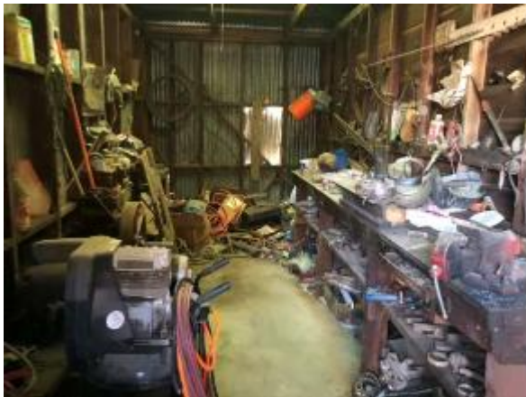
Photo #75 View of the air compressor room after cleanup. Refer to Photo #25.
