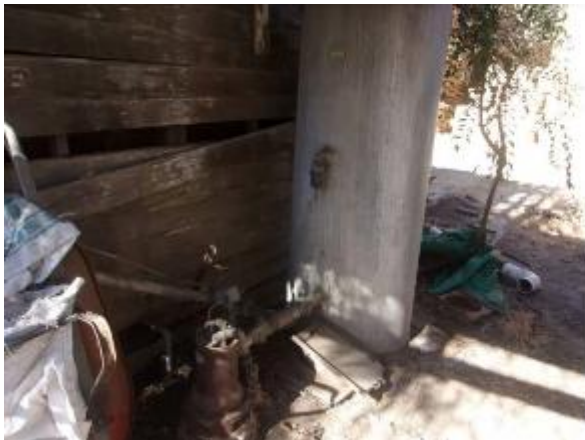
Photo #33 View of a non-functioning groundwater well located west of the calf barn.
