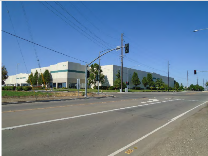
View toward Southwest adjoining properties
