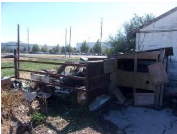
Photo #17 View of trash and debris located on the northern portion of the milk barn exterior.
