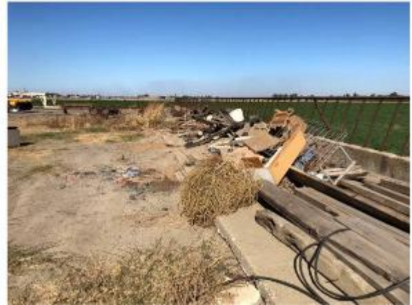
Photo #50 View of debris piles along the east side of the equipment storage area.
