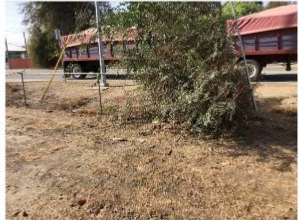
Photo #74 View of the location of the gasoline and diesel ASTs after removal. Refer to Photo # 22.
