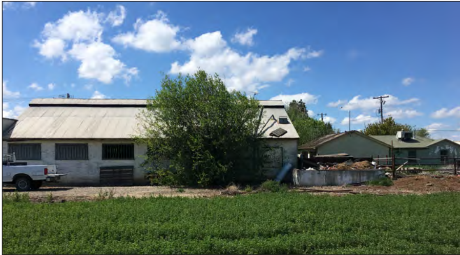
Photograph 19: View of the residences at the southwest corner of the project site; facing west.
