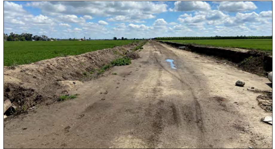
Photograph 4: View of dirt road entering the project site at the intersection of Paradise Road and West Pescadero Avenue; facing east.
