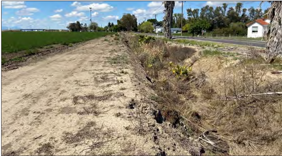
Photograph 13: View of northern boundary of project site along California Ave; facing northwest.
