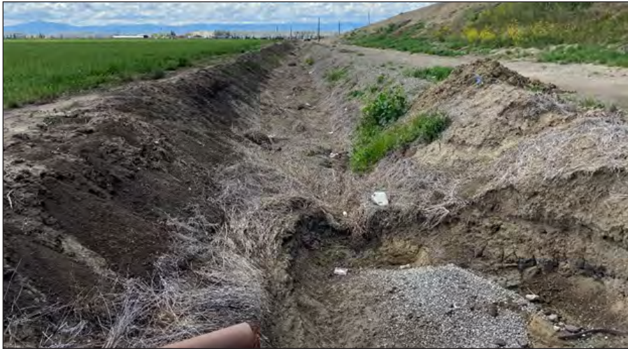
Photograph 3: View of drainage ditch running along the western side of the future interchange area; facing south.
