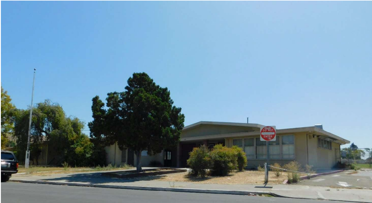
Figure 2. Western half of the north (main) elevation, looking SE (DSCN3867)
