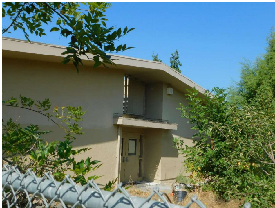
Figure 18. East elevation showing slatted screen and cantilevered overhang above the double entry door, looking NW (DSCN3837)
