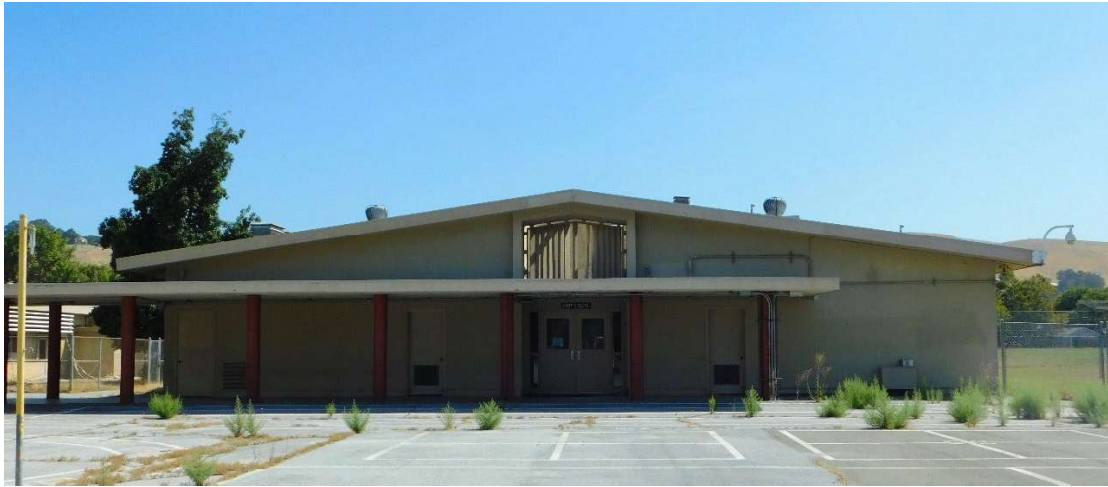
Figure 9. Western elevation showing covered walkway connection, looking E (DSCN3822)
