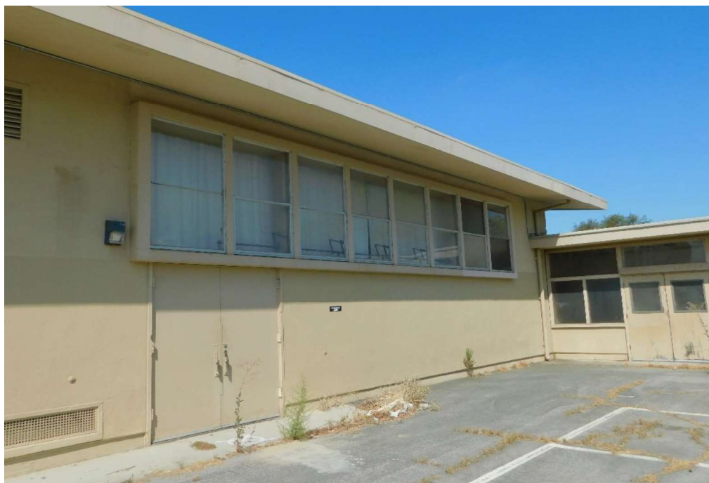
Figure 11. Protruding windows on east-facing section of rear elevation, looking NW (DSCN3793)
