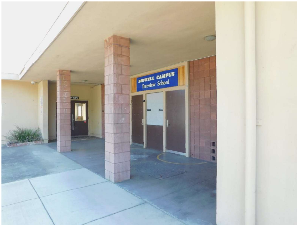
Figure 10. Recessed entry on the north (main) elevation showing sienna CMU details, looking SE (DSCN3750)
