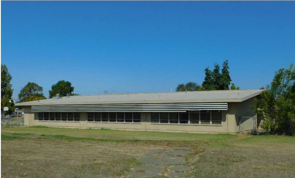
Figure 11. South elevation view showing brise soleils, view looking NW (DSCN3790)
