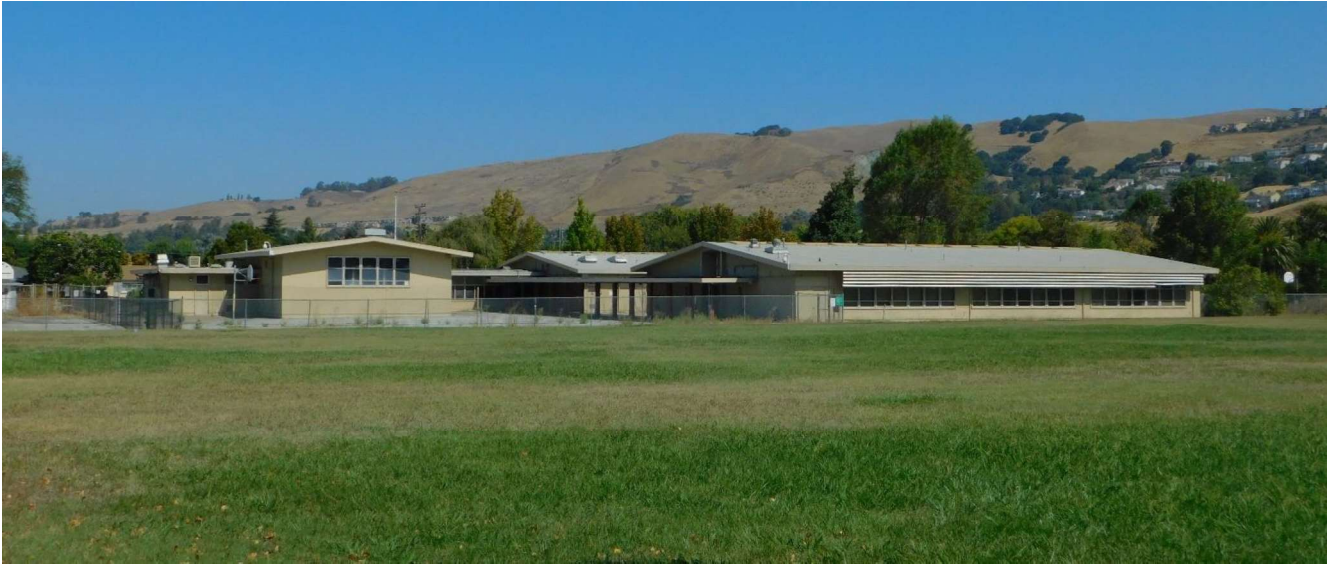
Figure 7. Rear view of Buildings A (at left and background) and B (right foreground), view looking north (DCSN3830)
