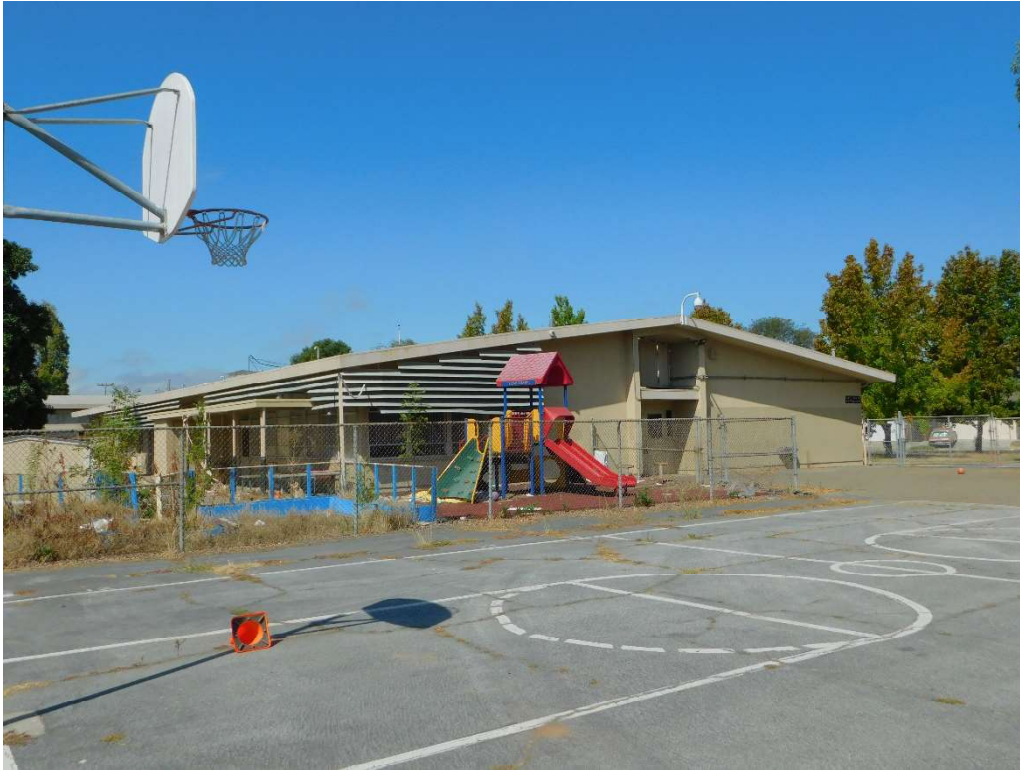
Figure 6. Brise soleils on south and east elevations, looking NW (DSCN3801)
