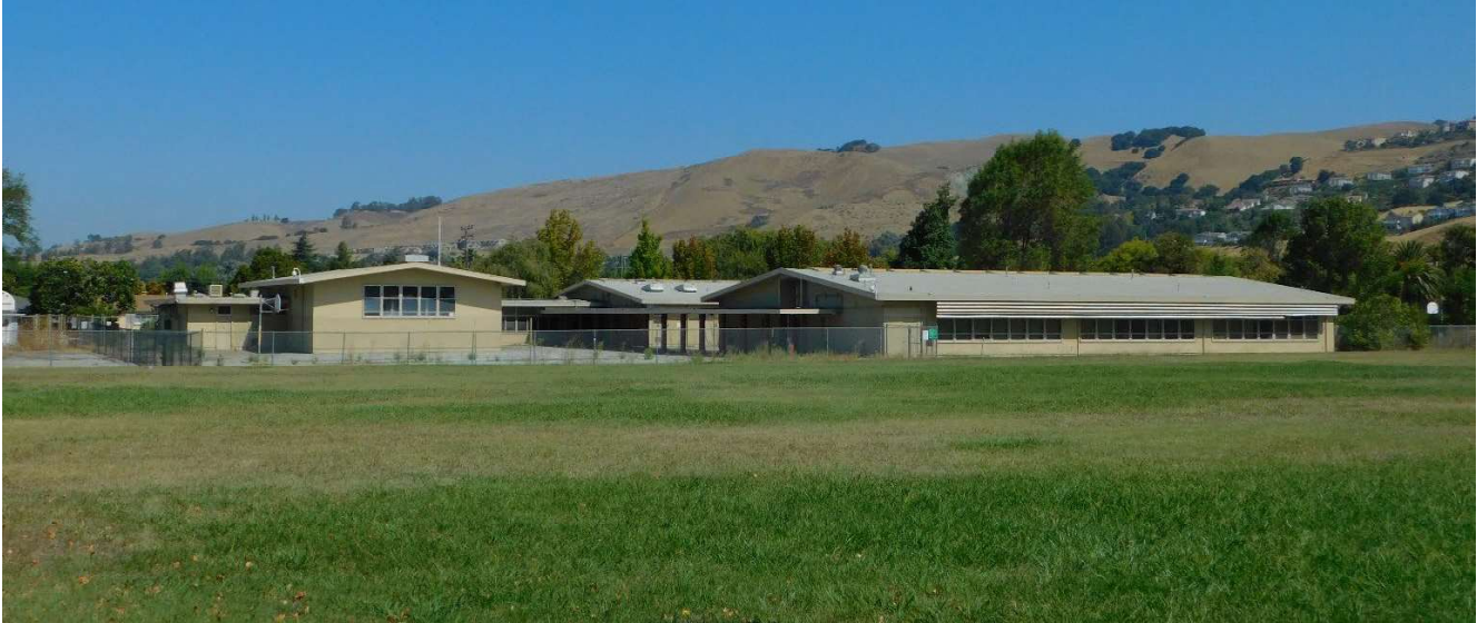
Figure 1. Rear view of Buildings A (at left and background) and B (right foreground), view looking north (DCSN3830)
