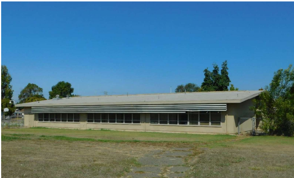
Figure 17. South elevation view showing brise soleils, view looking NW (DSCN3790)
