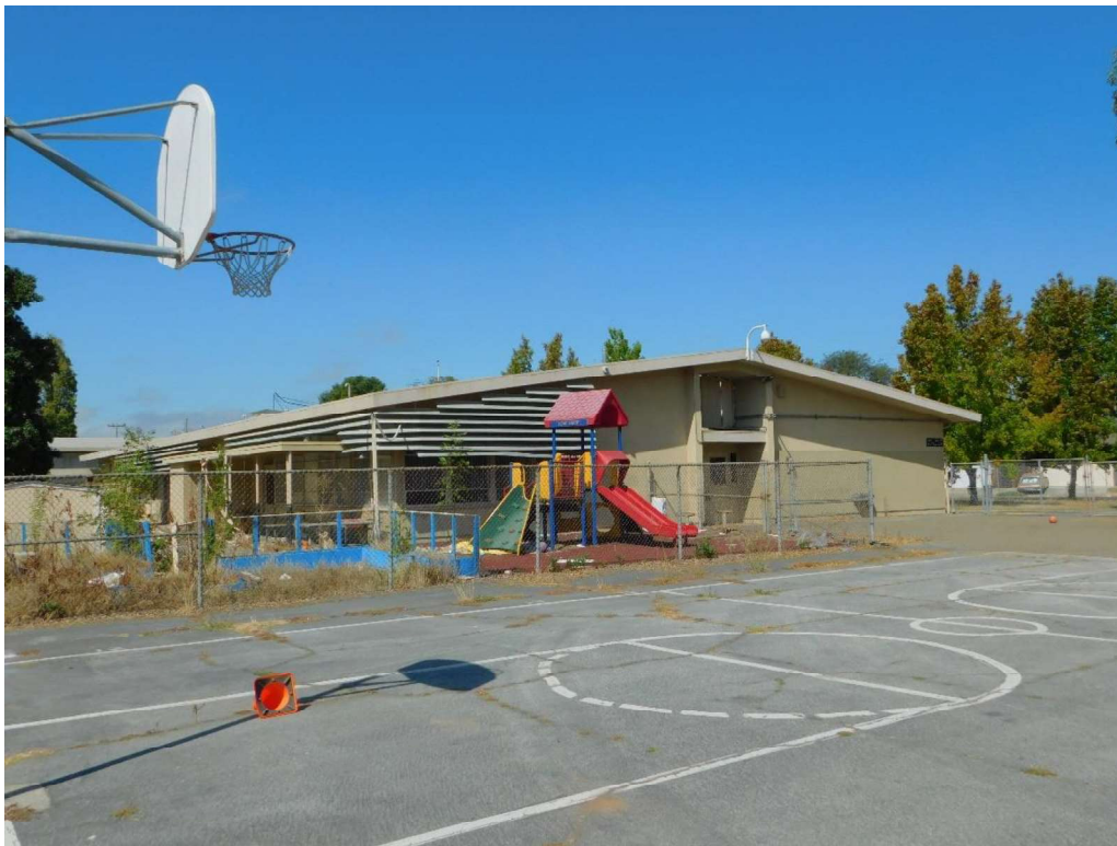
Figure 12. Brise soleils on south and east elevations, looking NW (DSCN3801)
