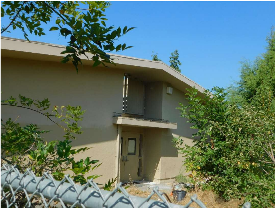
Figure 12. East elevation showing slatted screen and cantilevered overhang above the double entry door, looking NW (DSCN3837)
