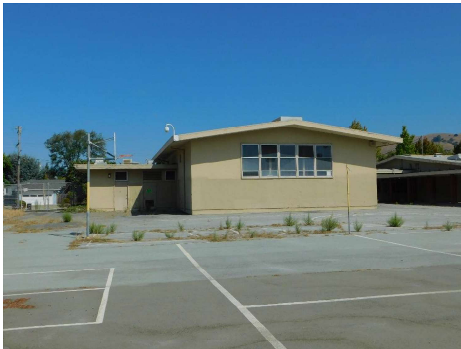
Figure 9. South (rear) elevations of Building A showing roof heights and types, looking NE (DSCN3785)
