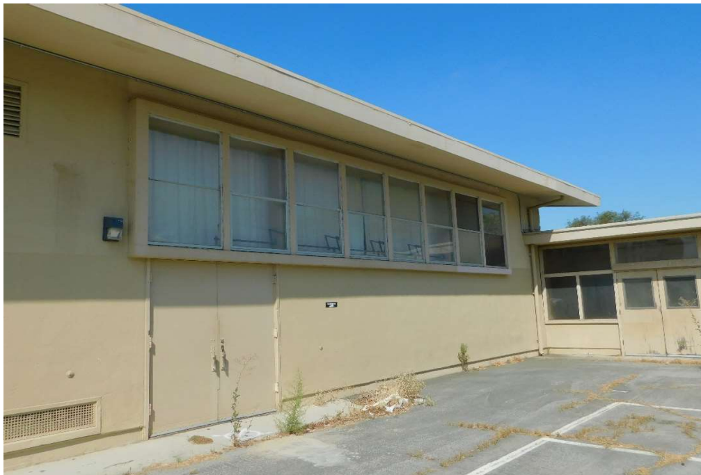
Figure 5. Protruding windows on east-facing section of rear elevation, looking NW (DSCN3793)
