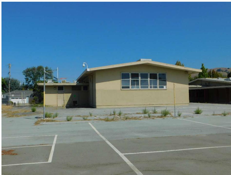
Figure 3. South (rear) elevations of Building A showing roof heights and types, looking NE (DSCN3785)
