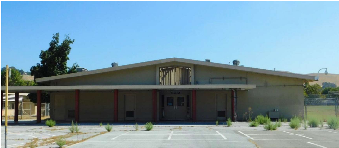
Figure 15. Western elevation showing covered walkway connection, looking E (DSCN3822)
