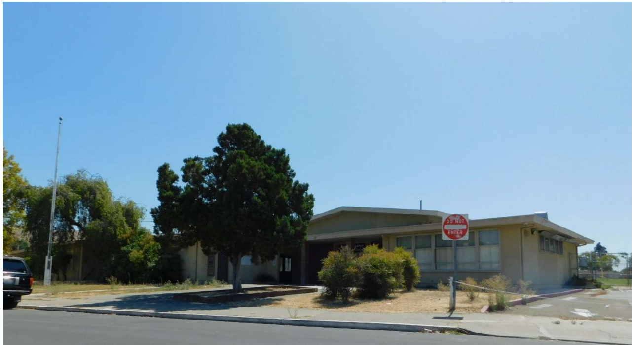
Figure 8. Western half of the north (main) elevation, looking SE (DSCN3867)
