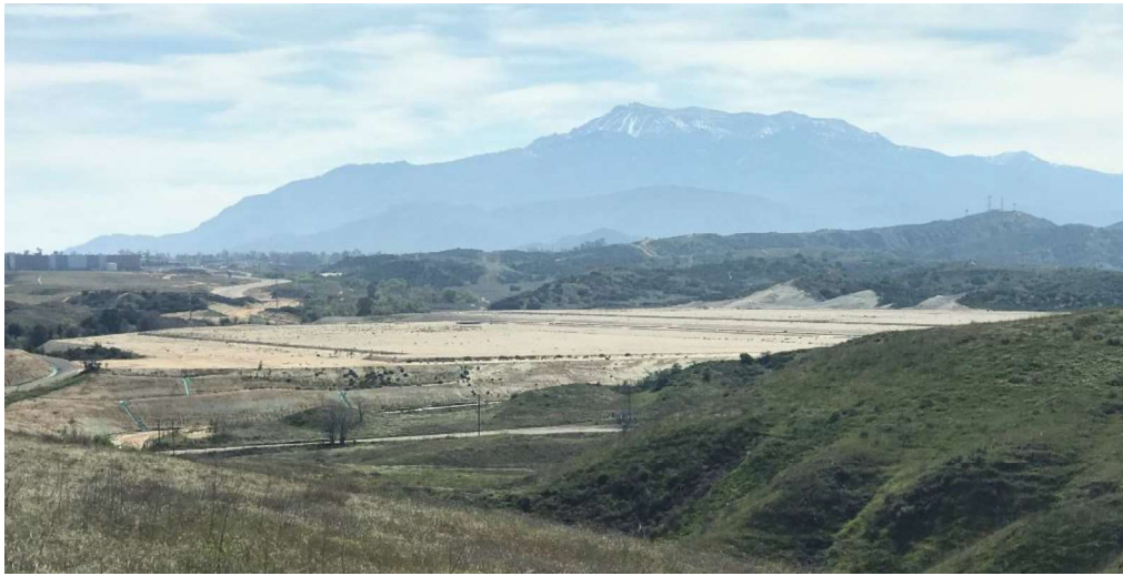
Photograph 12. View of the Hidden Canyon development currently in the grading phase east of the Project site.
