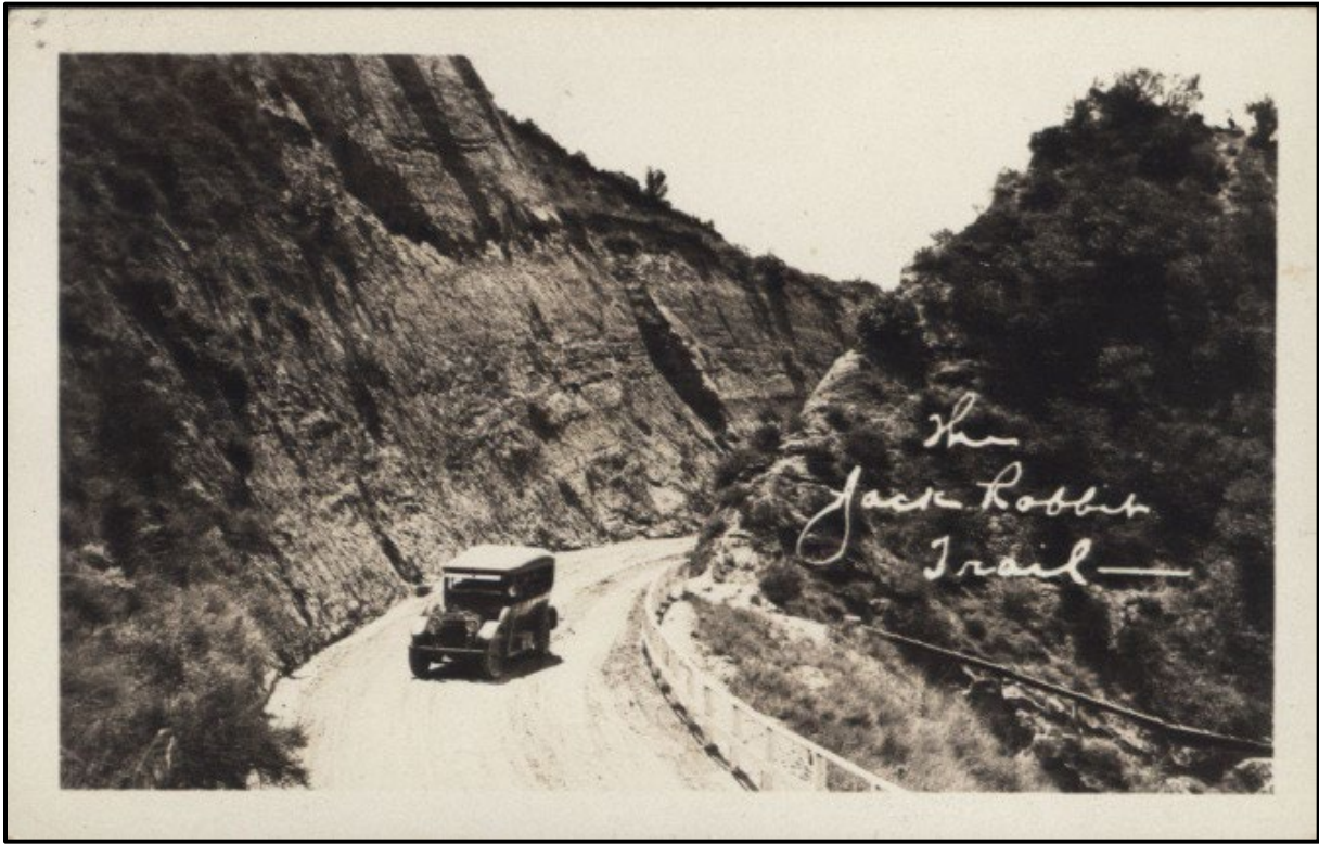
Plate 4.1–1: Jack Rabbit Trail with wooden guardrails (circa 1920s). (Photograph courtesy of Press Enterprise)
