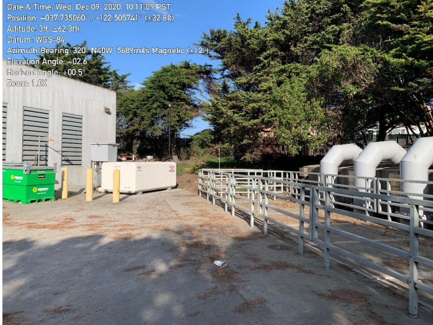
Photograph 1 (P1) Photo of developed/landscaped areas.
