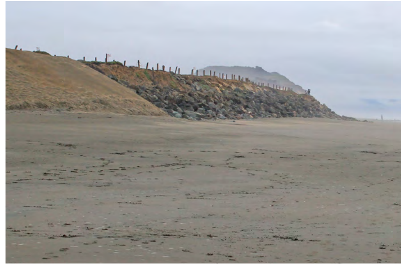
Photo 2. View from South Ocean Beach nearing the rubble revetments, facing south.
