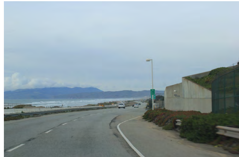
Photo 4. View from a vehicle driving along the Great Highway, adjacent to the Oceanside Treatment Plant, as it bends away from the Pacific Ocean.
