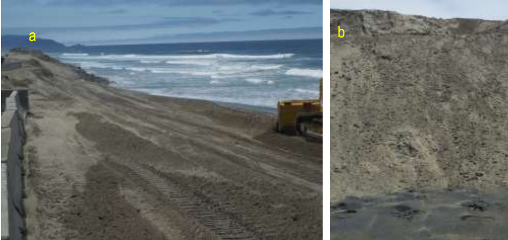
Figure 1. Artificial sand fill, South Ocean Beach, June 2013. Sand sources include beach and dune sand mechanically harvested from North Ocean Beach, and deposited below the erosional scarp south of Sloat Blvd. Deposition by grading (a) and avalanche slope (b) processes eliminates internal bedding structure and can increase the range of grain sizes deposited.
