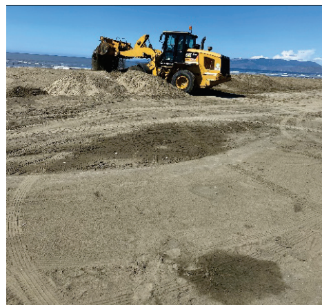
Mechanical Placement Observed
