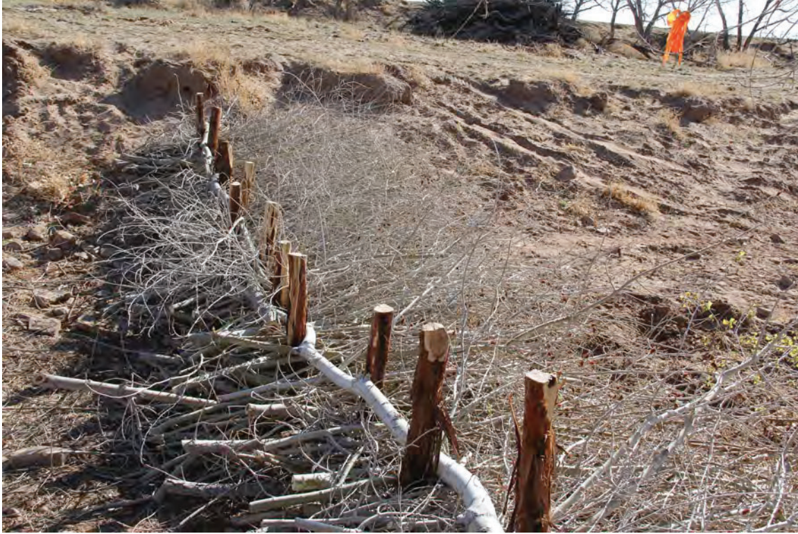
Figure 82: BDA interwoven with cottonwood branches parallel and perpendicular to the stream flow. The perpendicular, downstream (left to right) branches are placed to limit the development of a downstream scour pool during high-flow events, which could compromise the integrity of the structure. Photo courtesy of Seventh-Generation Institute.
