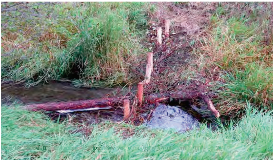
Figure 73: BDA – Two pilings extending onto the bank with LWD placed through the structure
