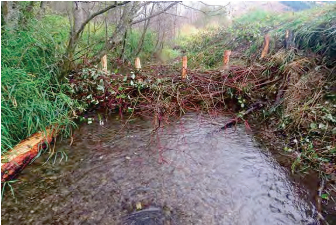
Figure 75: Pilings woven with live red oyster dogwood, some of which was planted directly into the exposed bank to facilitate resprouting
