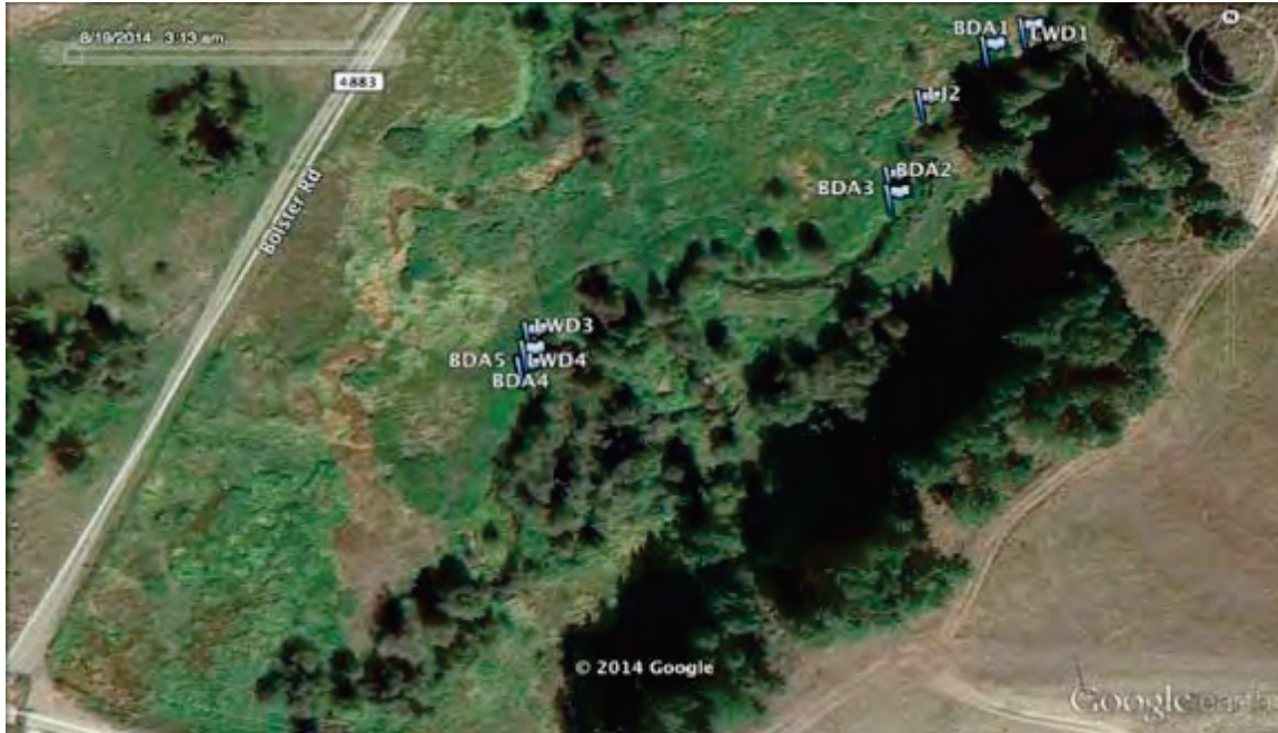
Figure 72: Myers Creek restoration site showing locations of LWD and BDA placement
