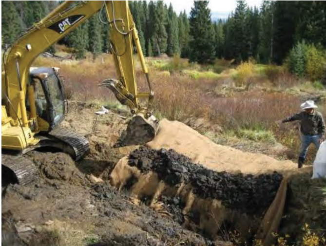
Figure 62: Breached dams were “plugged” with soil lifts wrapped in coir fabric and sod interwoven with live willow stems
