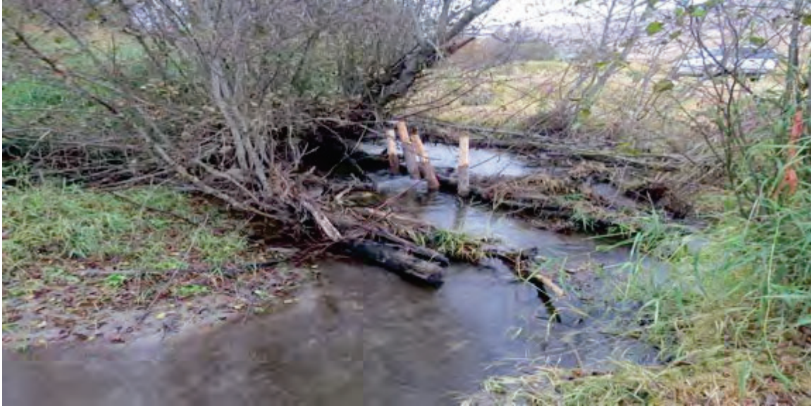
Figure 74: Partially channel spanning BDAs and LWD additions to a naturally occurring log and debris jam
