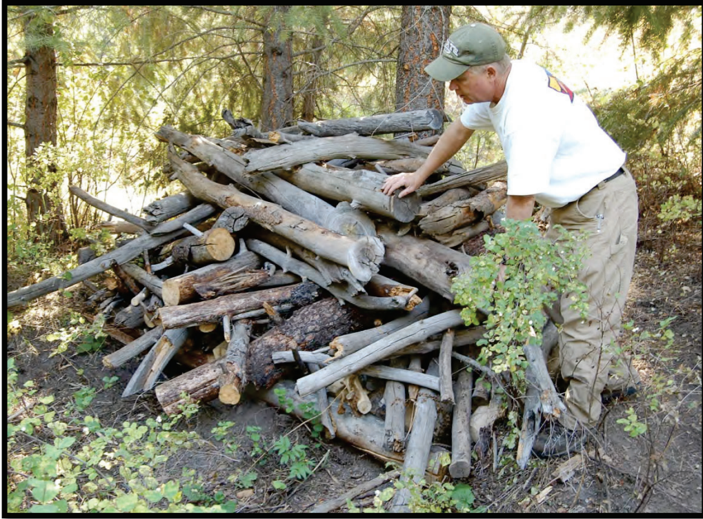
Figure 22: Construction of an artificial beaver lodge in the Methow Valley, Washington. The lodge opening faces the water and is about 10 feet away from the water’s edge.
