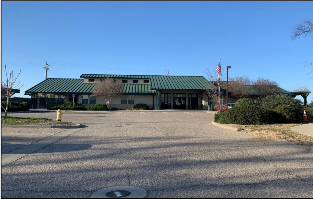
Figure ES-5. Existing County Sheriff building on the parcel.
