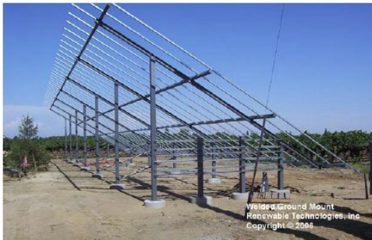
Typical Fixed-Tilt Mounting Structure
