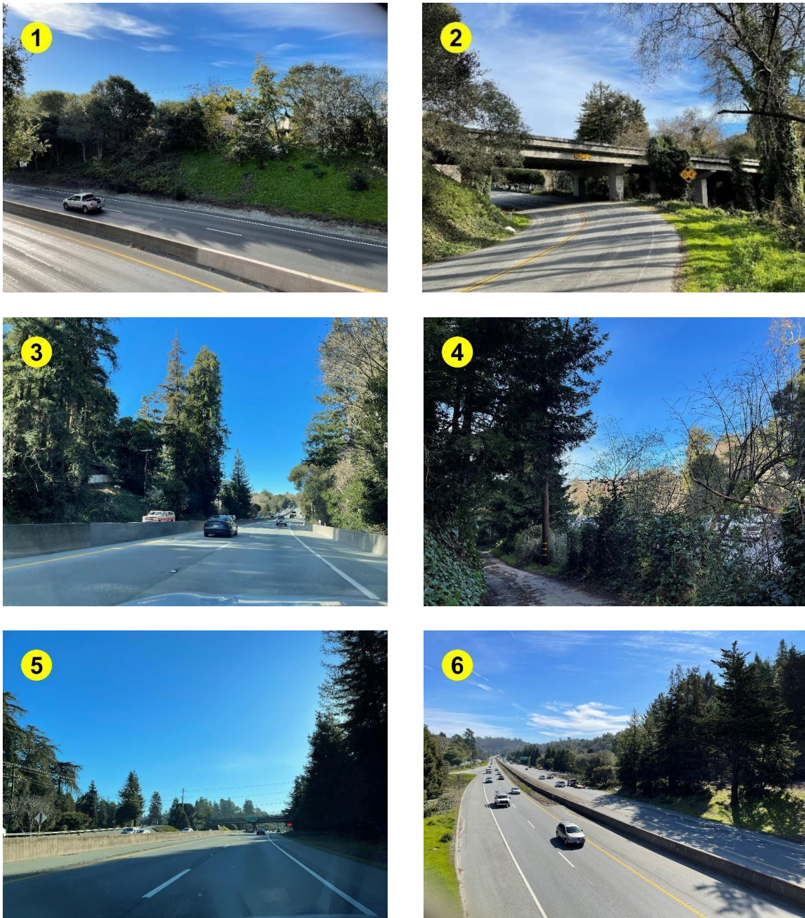
Figure 2-8. State Route 1 Visual Assessment Unit Typical Views
