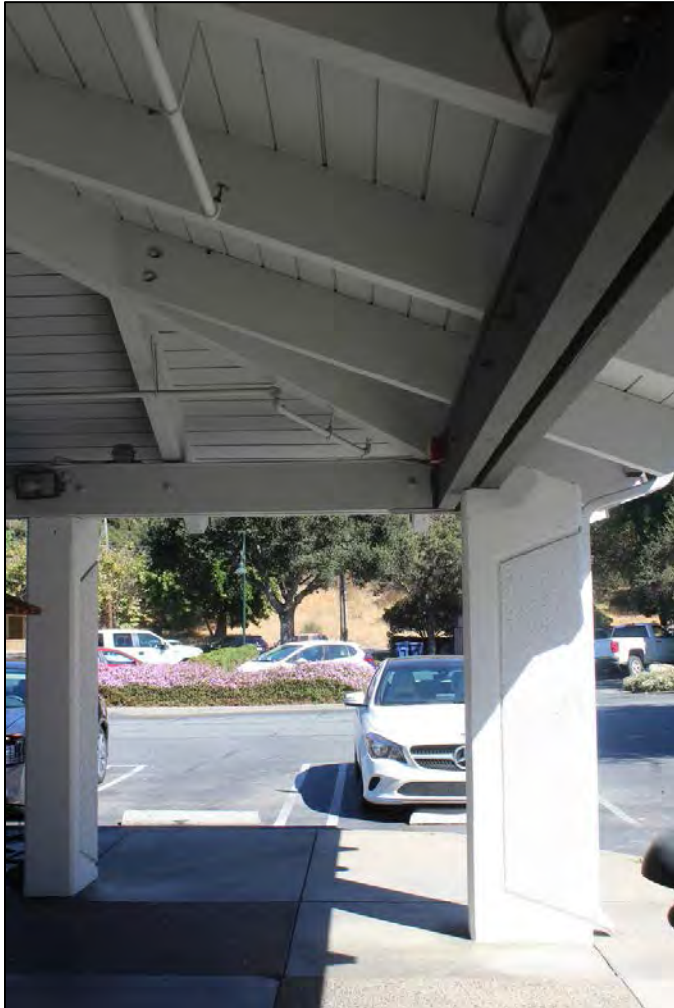
Building C walkway detail, northeast corner, typical
