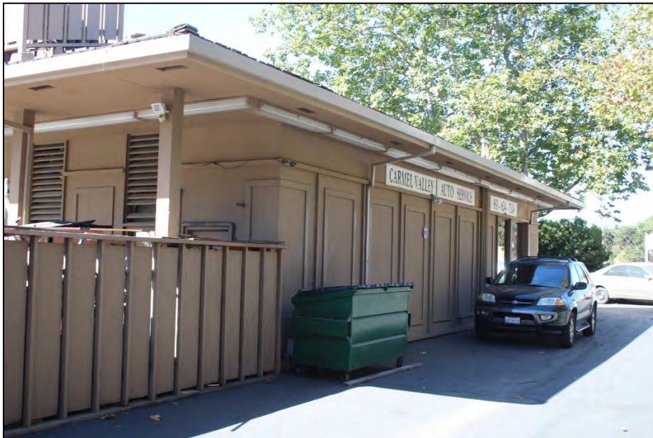
Rear east façade, looking north
