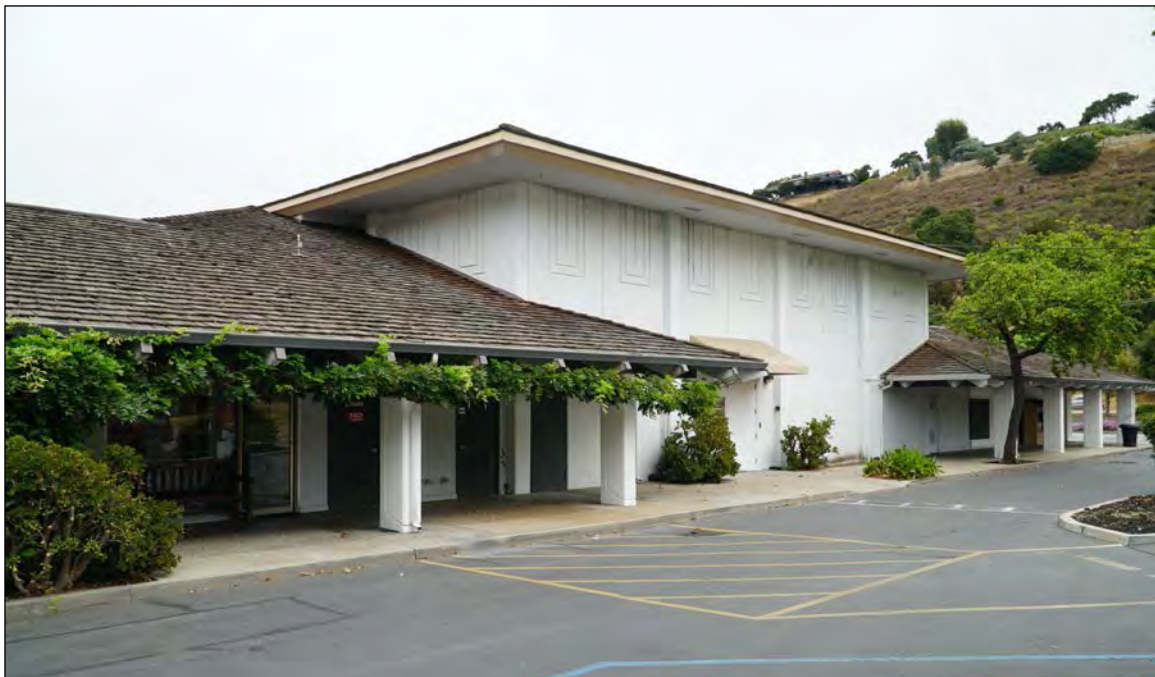
Figure 9. Looking northwest at east side of Building B-2, 19 August 2019.
