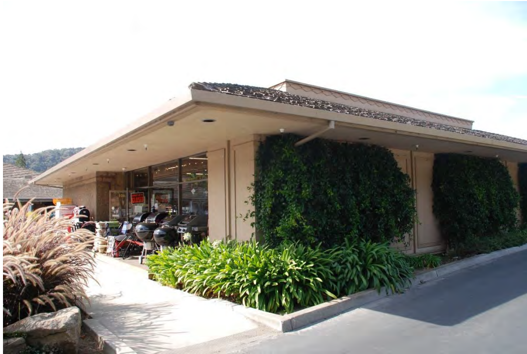
Figure 21. Building D, southeast and northeast façades, view southwest.
