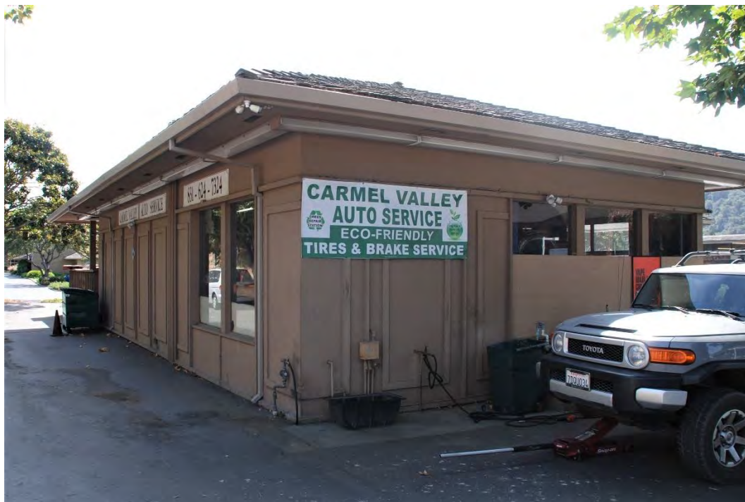
Figure 27. Building E, northwest and northeast façades, view southeast.
