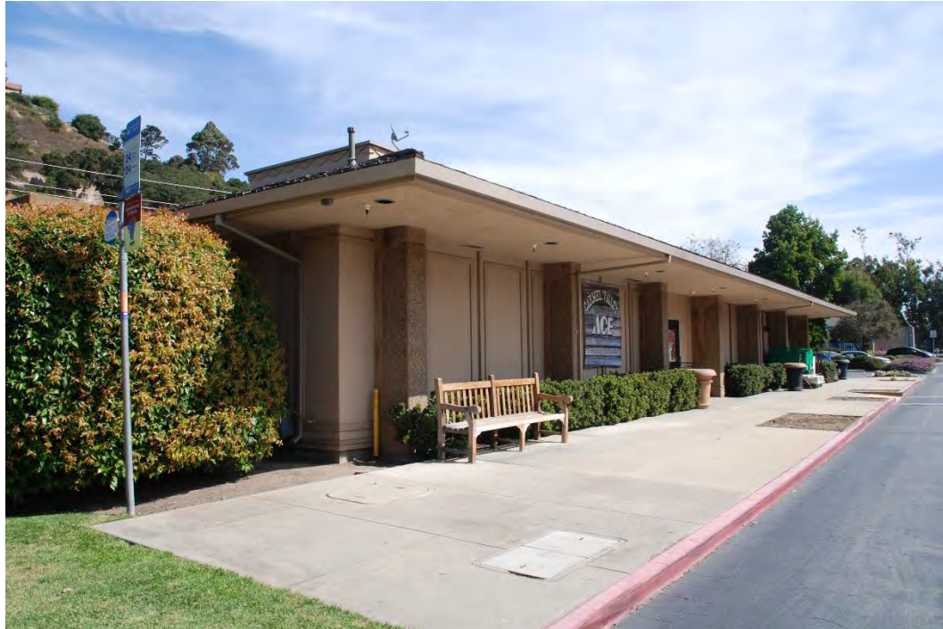
Figure 24. Building D, southwest façade, view east.
