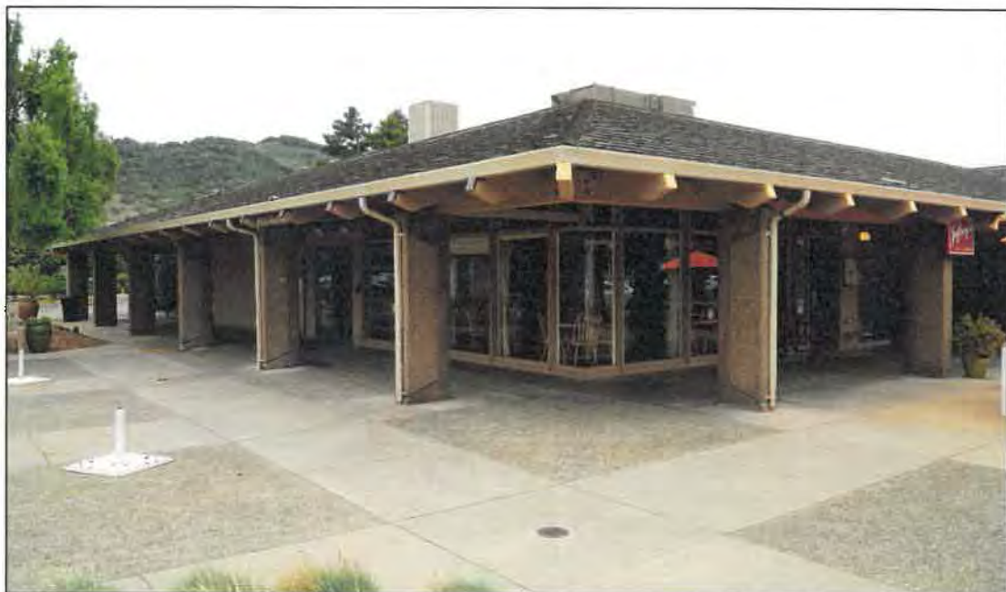
Figure 2. Looking southwest at east and north sides of Block 1, 19 August 2019.
