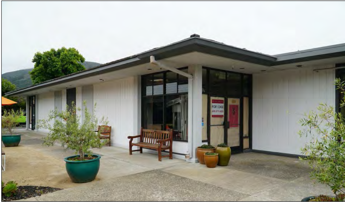
Figure 6. Looking southeast at north side of 1981 section of Building C, 19 August 2019.
