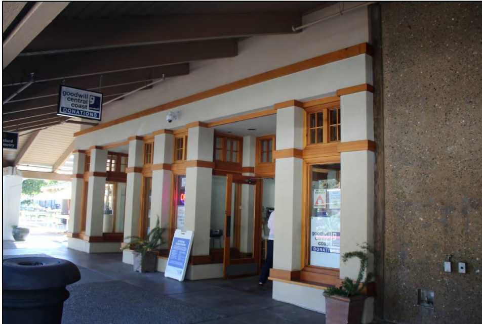
Former Steinmetz Pharmacy, west façade, looking southwest
