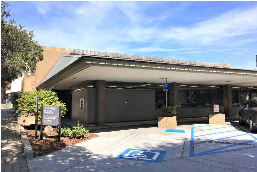
Figure 54. Wells Fargo building, Carmel-by-the-Sea, view northeast.
