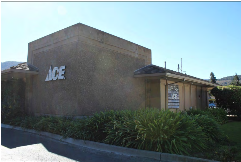
Pylon detail at northeast corner
