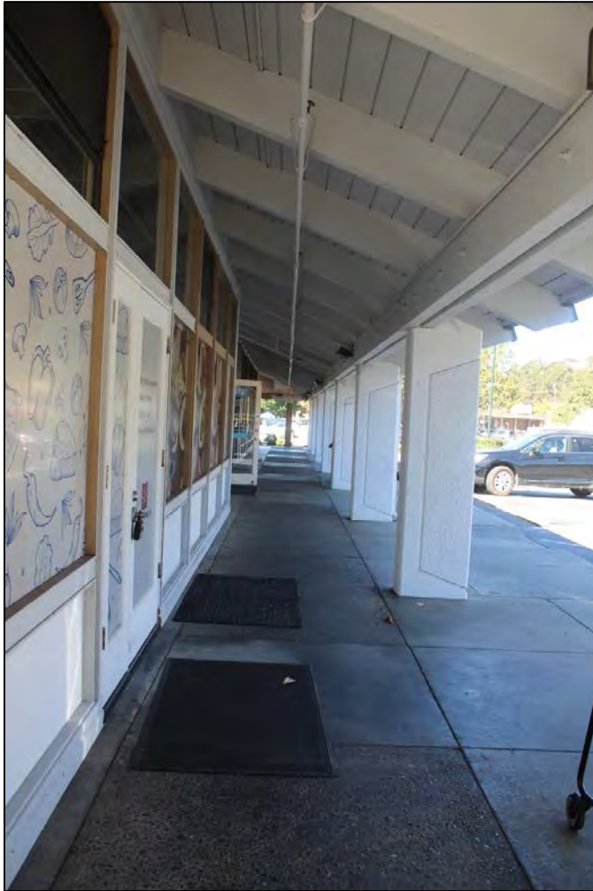
East façade, exterior walkway, looking north
