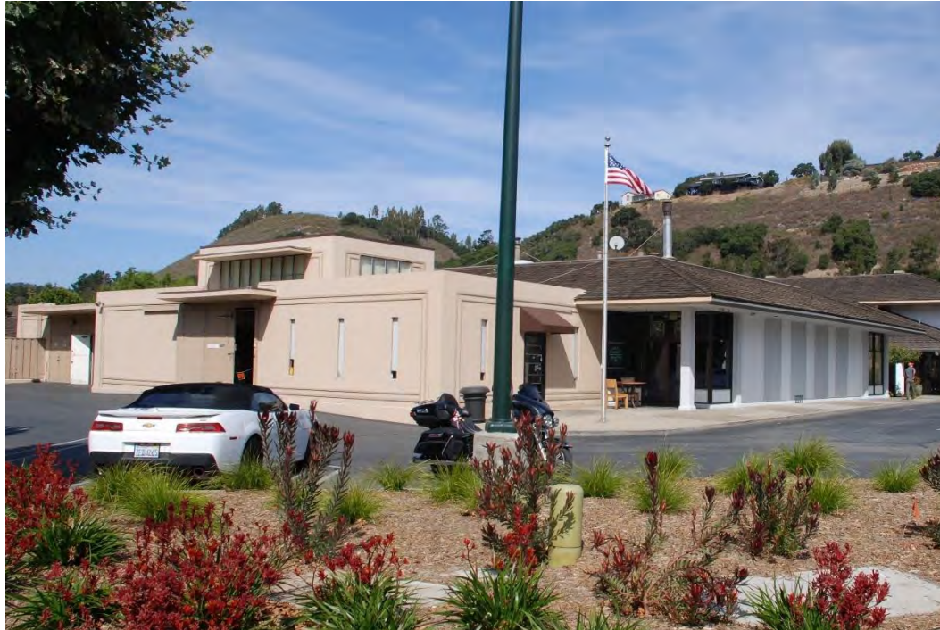
Figure 12. Building B, east portion of southwest façade and southeast façade, view north.
