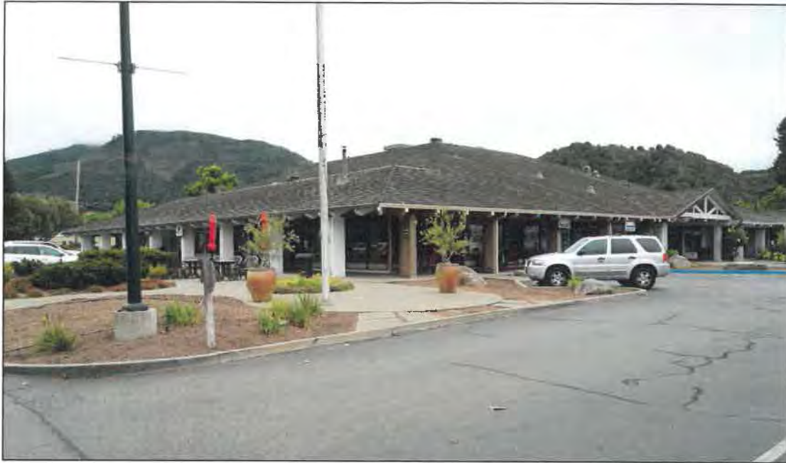
Figure 7. Looking southeast at north and west sides of Block 3, 19 August 2019.
