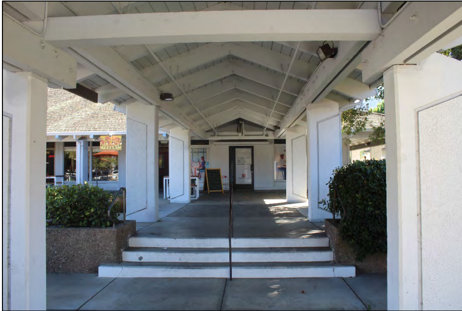
Covered walkway from Safeway to Building C, looking south
