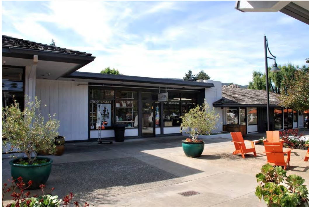
Figure 9. Building B, western portion of northeast façade, overlooking courtyard, view southwest.
