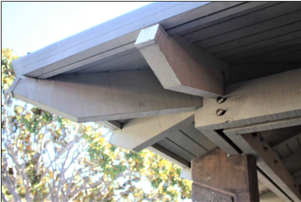
Framing of walkway and column detail, typical
