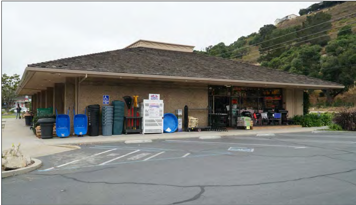
Figure 10. Looking northwest at south and east sides of Building D, 19 August 2019.
