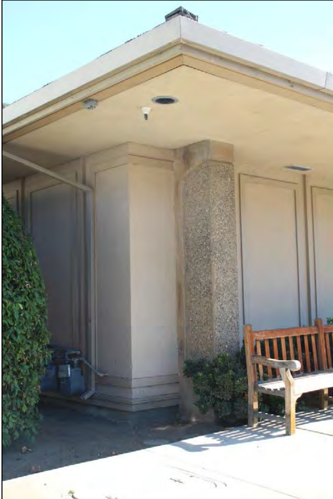
Pilaster detail, northwest corner
