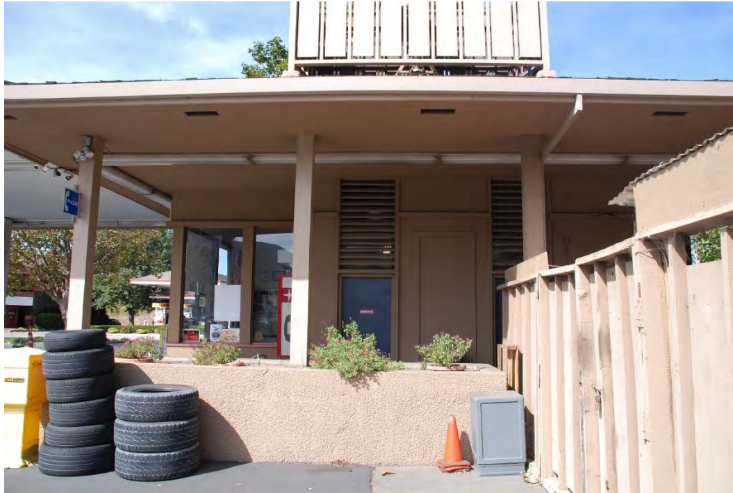
Figure 28. Building E, southeast façade, view northwest.
