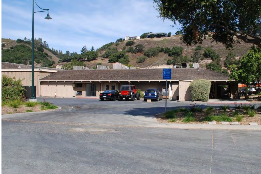
Figure 7. Building A, southeast portion of southwest façade, rear of stores to southeast of Safeway, view northeast.
