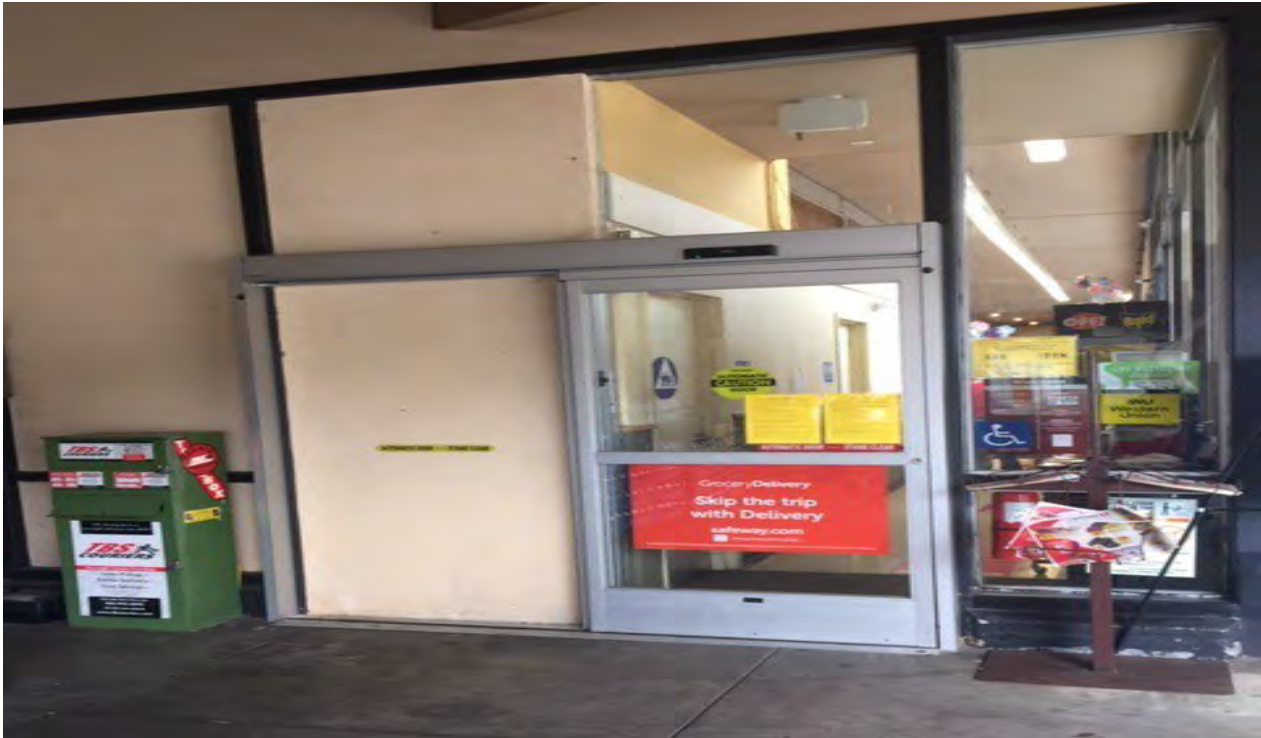
Figure 6. Infill of glass wall at east entry to store
