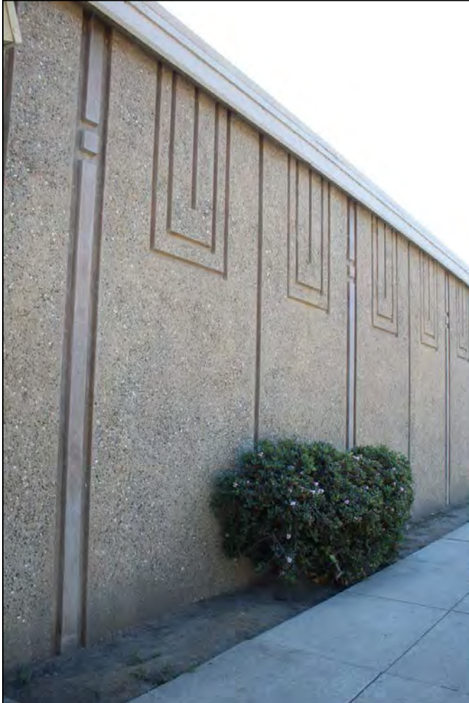
North side façade, looking west
