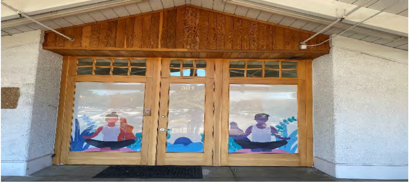
Figure 16. Building entry in October 2020
