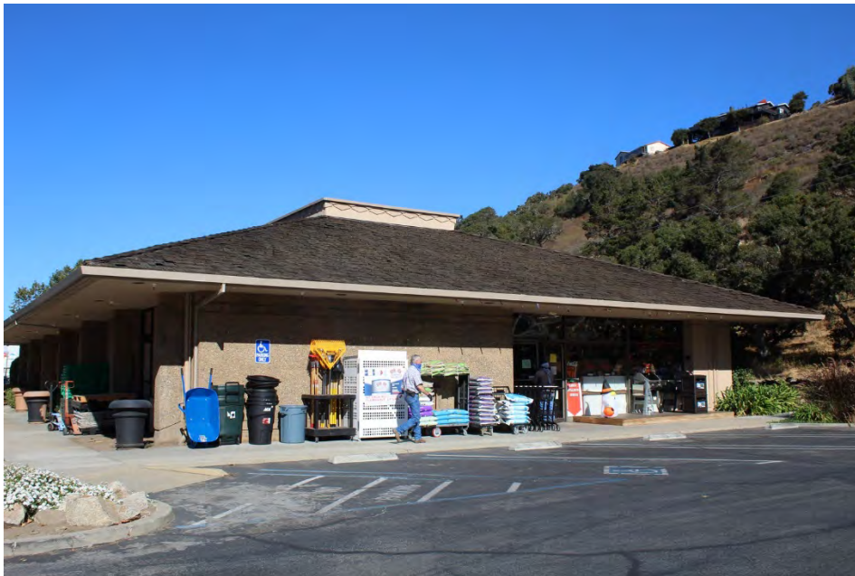
South entry façade, looking north
