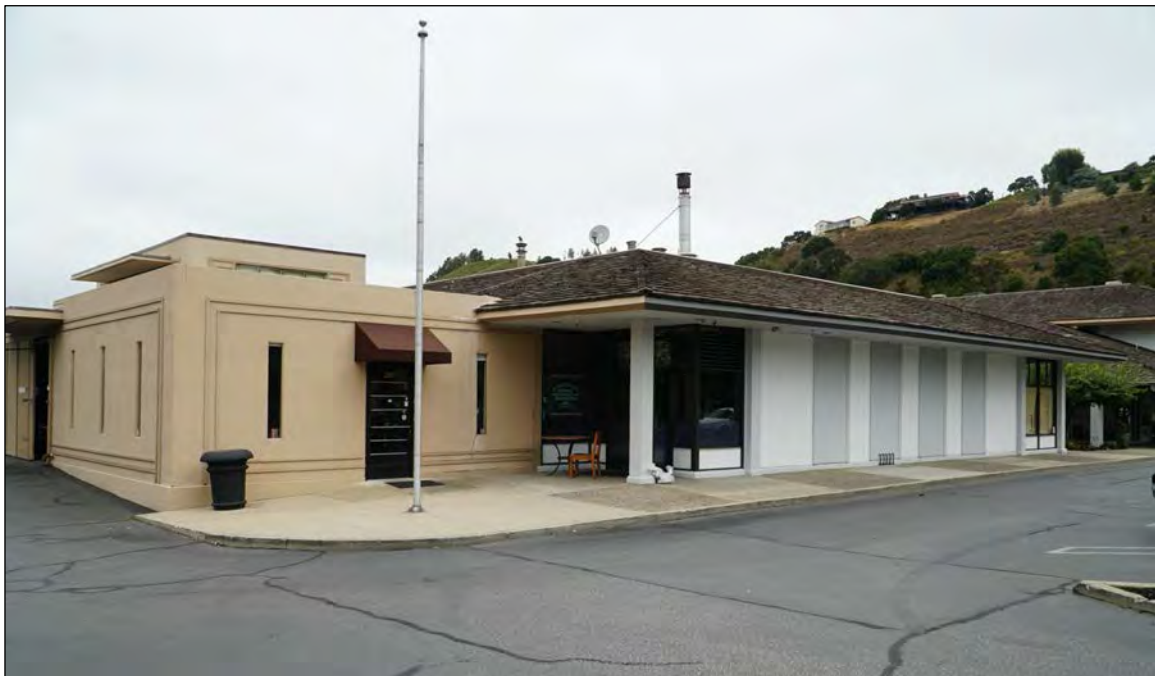
Figure 7. Looking northwest at south and east sides of 1981 and 1982 sections of Building C, 19 August 2019.
