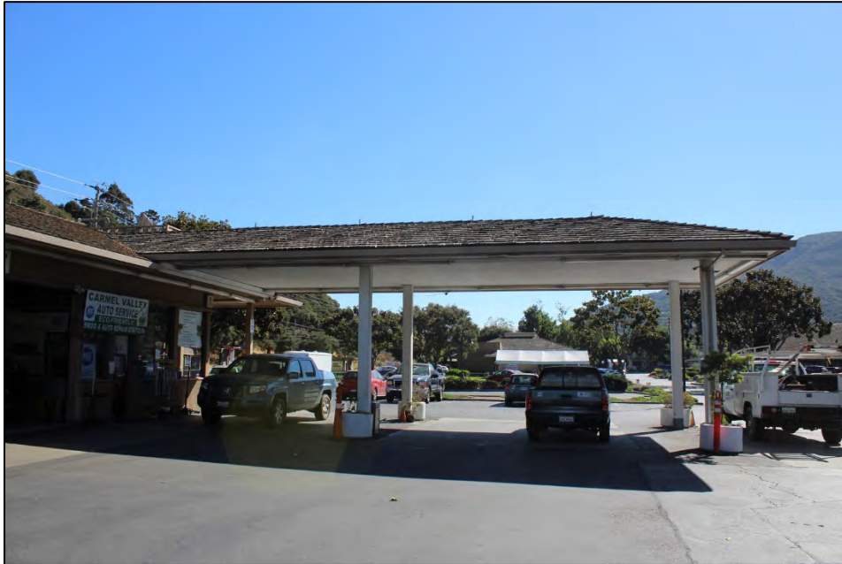
North side of canopy, looking south
