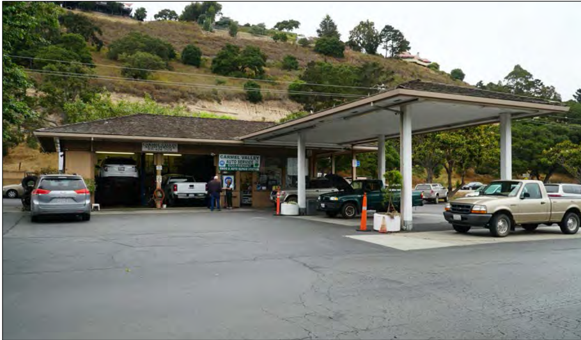
Figure 12. Looking northeast at south side of Building E, 19 August 2019.
