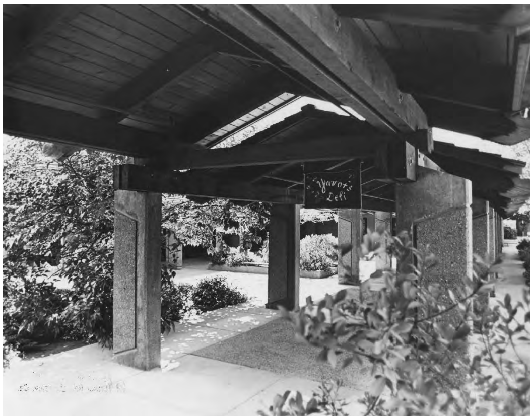
Figure 40. Covered walkway between Buildings A and C, ca. 1974, view northwest.
