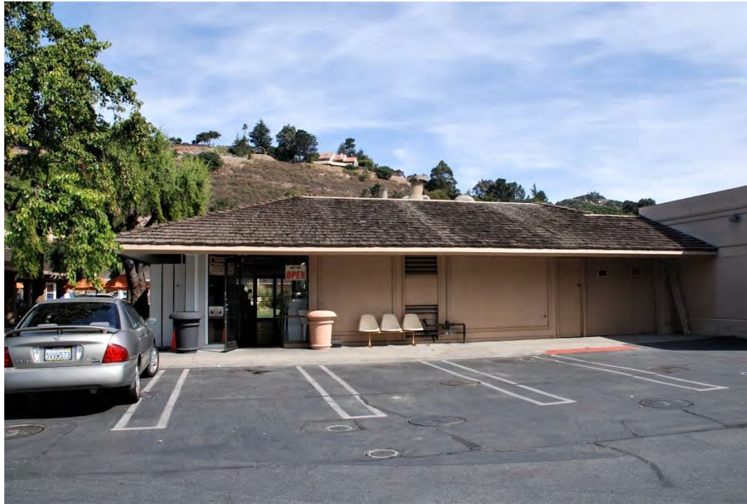
Figure 11. Building B, west portion of southwest façade, view northeast.
