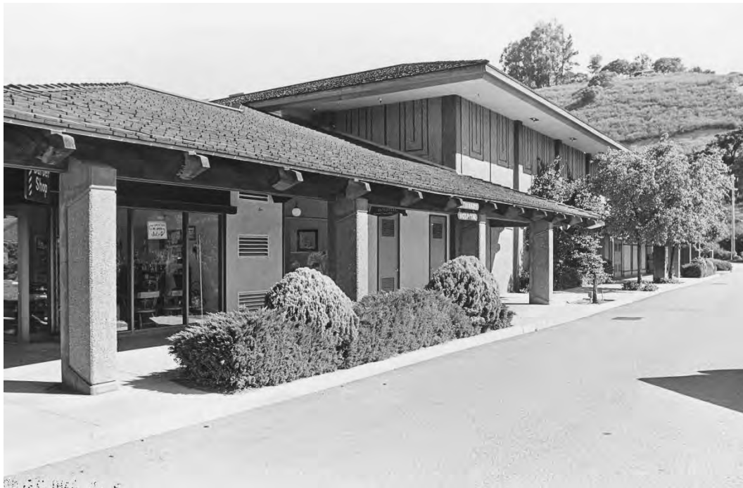
Figure 38. Building C, ca. 1974, view north.
