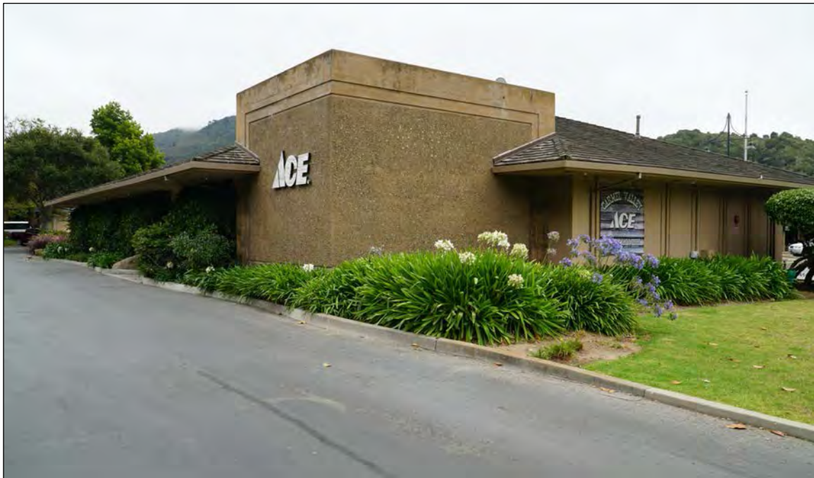
Figure 11. Looking southeast at north and west sides of Building D, 19 August 2019.
