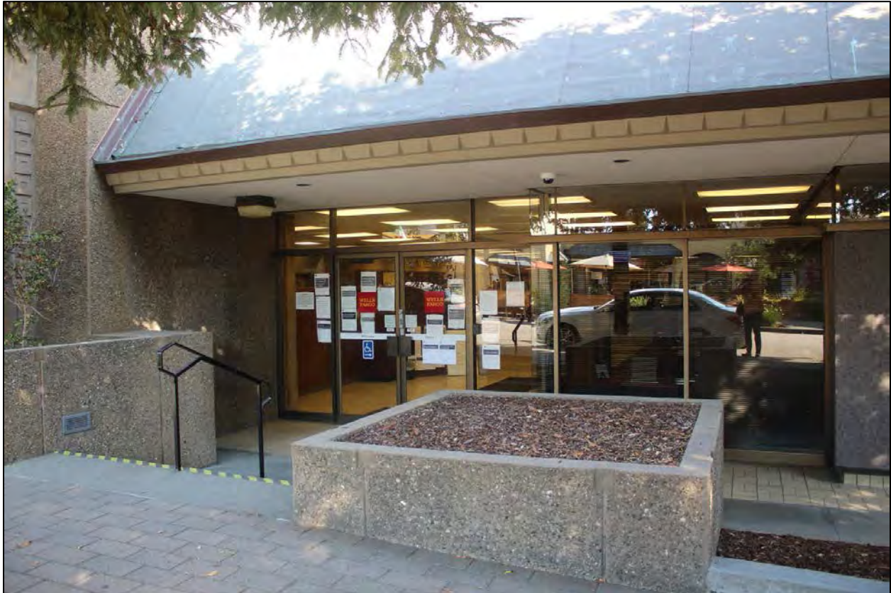
Wells Fargo Bank, design by Olof Dahlstrand, Carmel-by-the-Sea, 1965 Photo by Diana Painter
