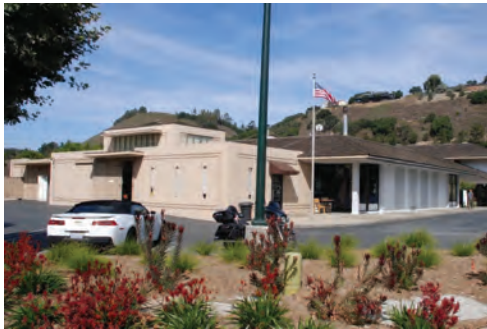
② Building B
