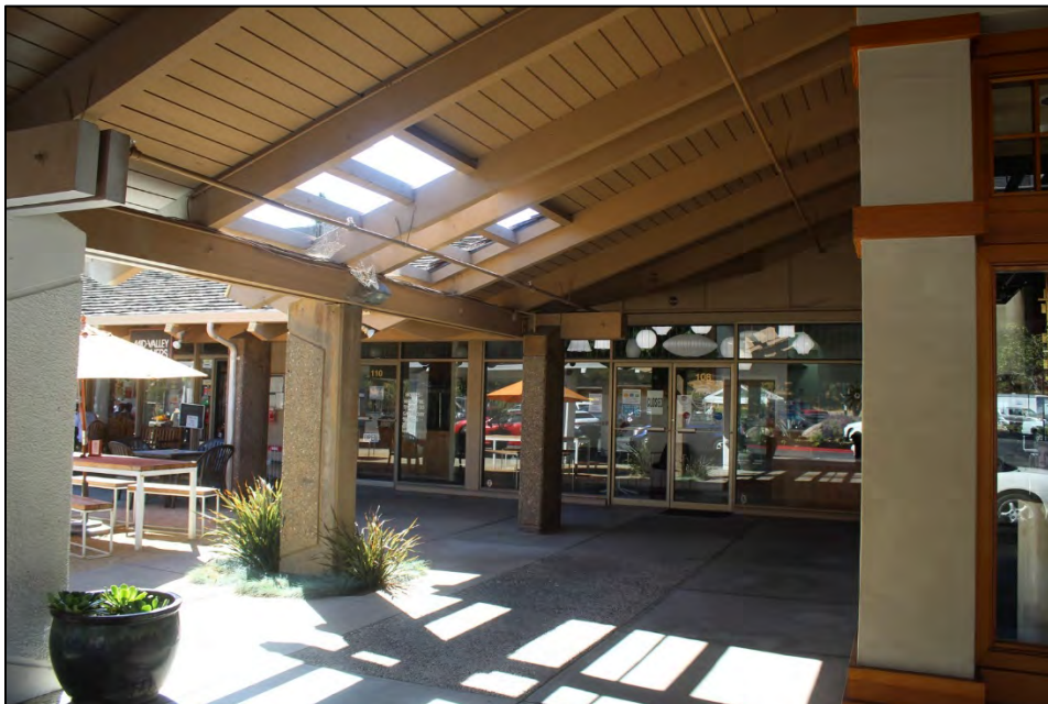
Covered outdoor space, south end of complex, looking west
