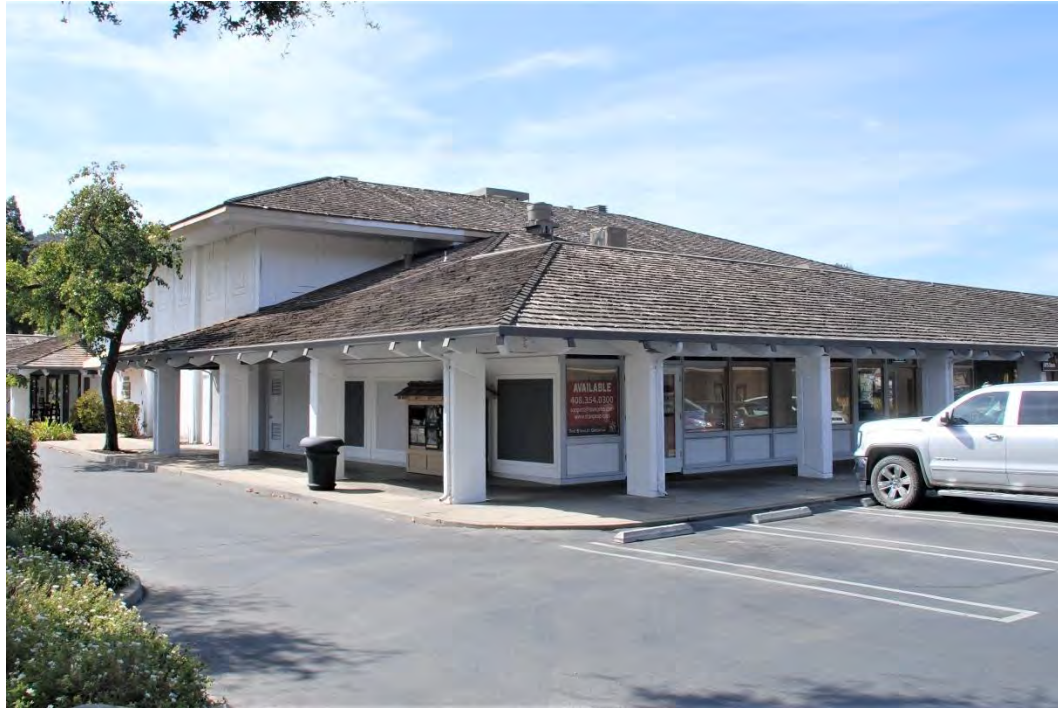
Figure 19. Building C, southeast and northeast façades, view southwest.
