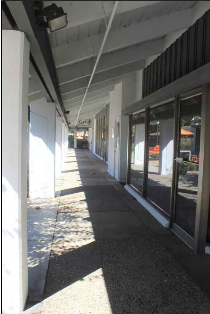
East façade, exterior walkway, looking south
