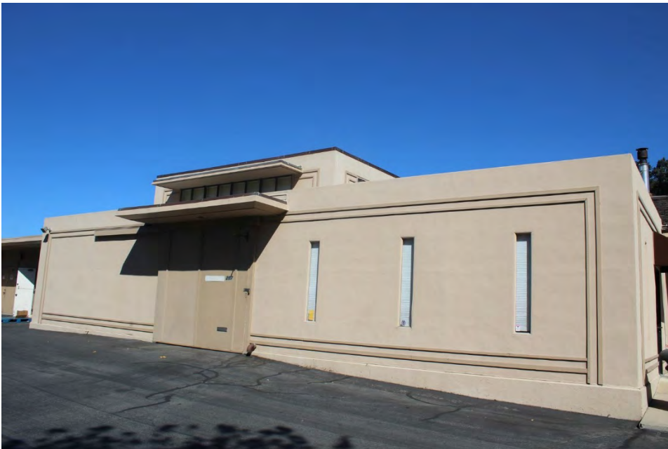
South façade, looking east
