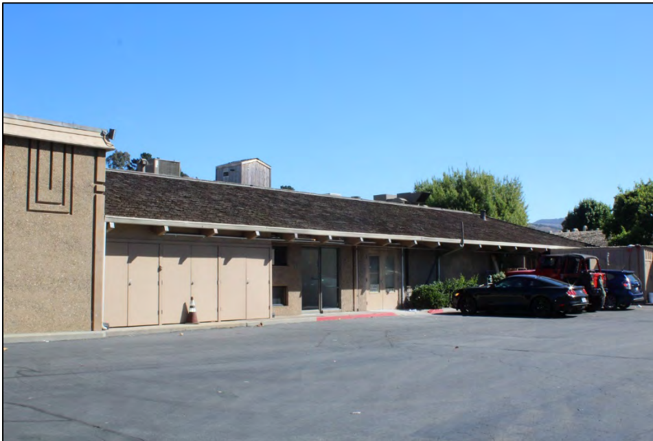
Rear west façade, south end, looking east
