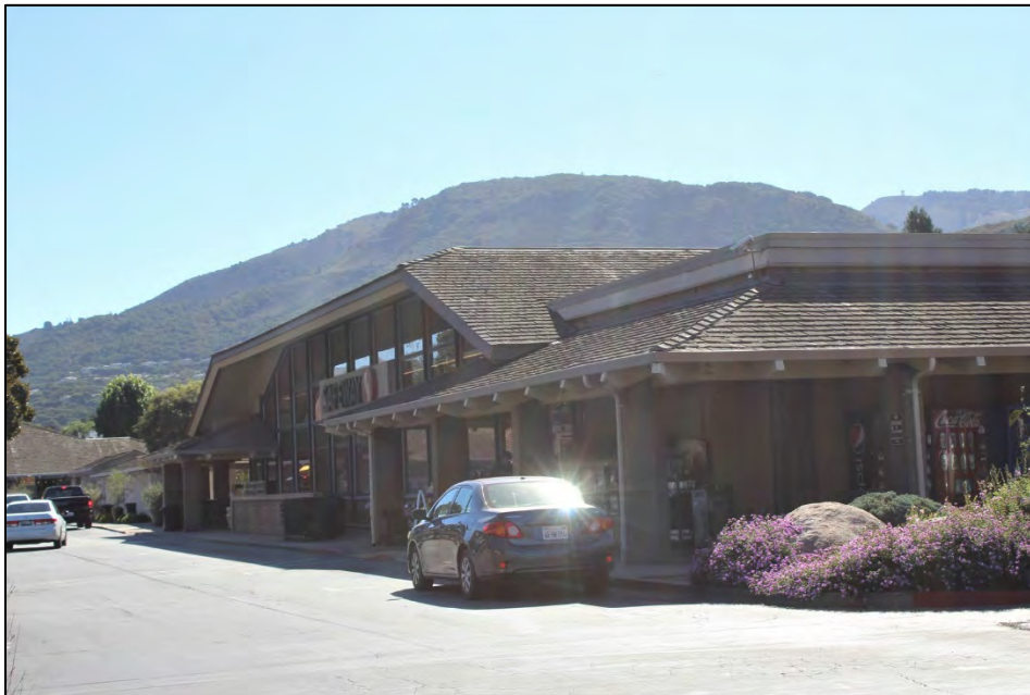
Front east façade and north side façade, looking southwest
