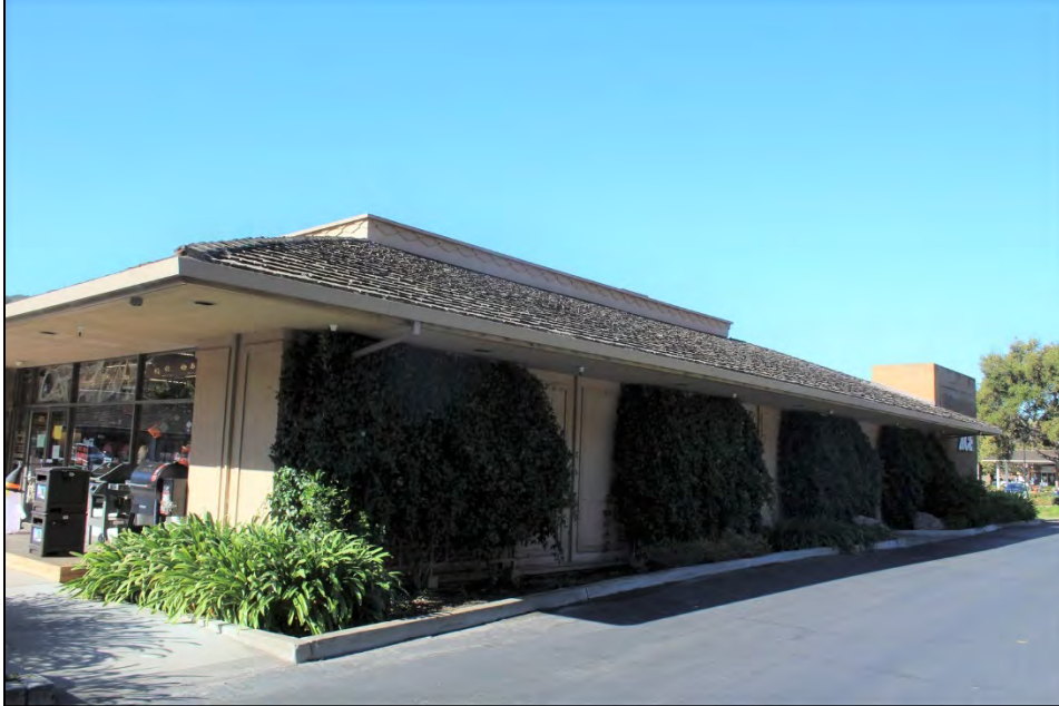
East side façade, looking northwest
