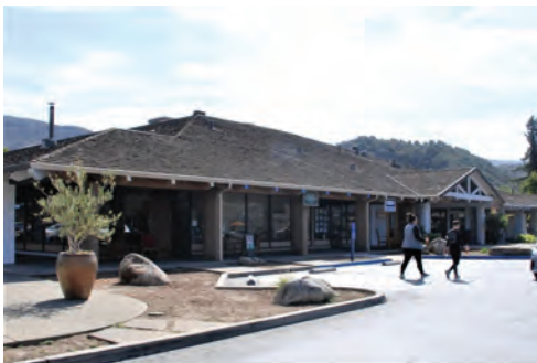
③ Building C
