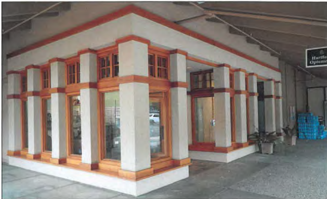
Figure 14. Looking southwest at two shops in Block 1, 19 August 2019. Their original appearance may be seen in Figure 13. The exteriors were radically altered about 1994.
