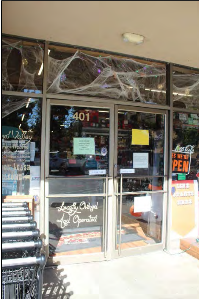
Entry detail, south facade
