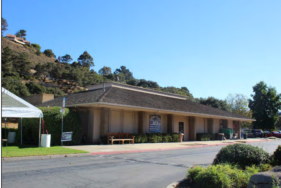
West side façade looking southeast
