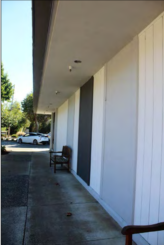
East façade, north end, looking south
