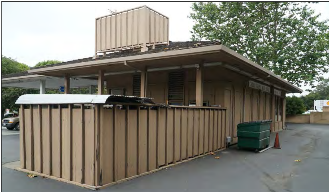
Figure 13. Looking southwest at east and north sides of Building E, 19 August 2019.
