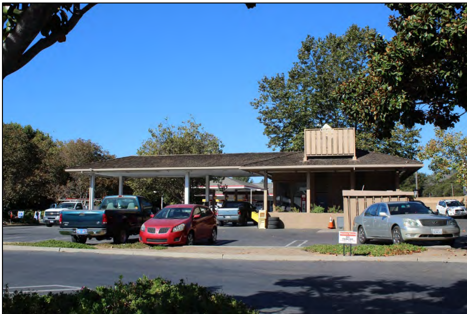
South side façade, looking north
