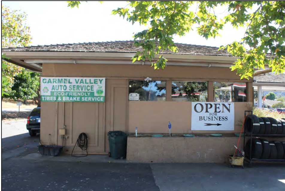
North side façade, looking south
