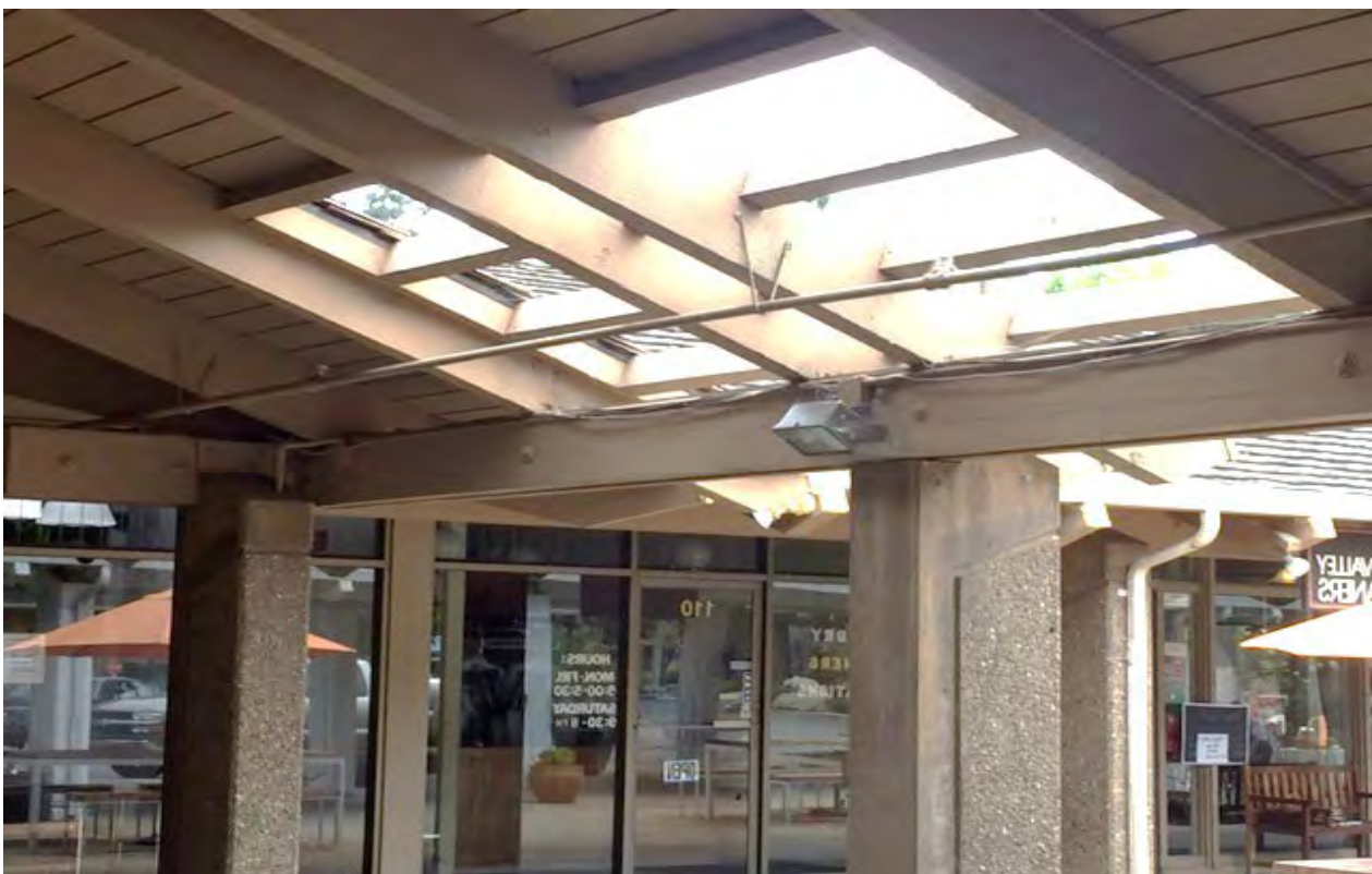
Figure 7. Removal of portion of arcade roof; painted-over stained wood surfaces
