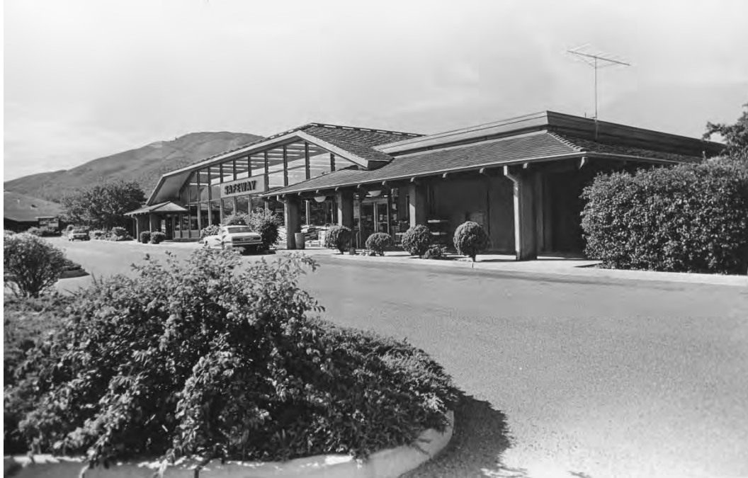
Figure 37. Building A, ca. 1974, view southeast.
