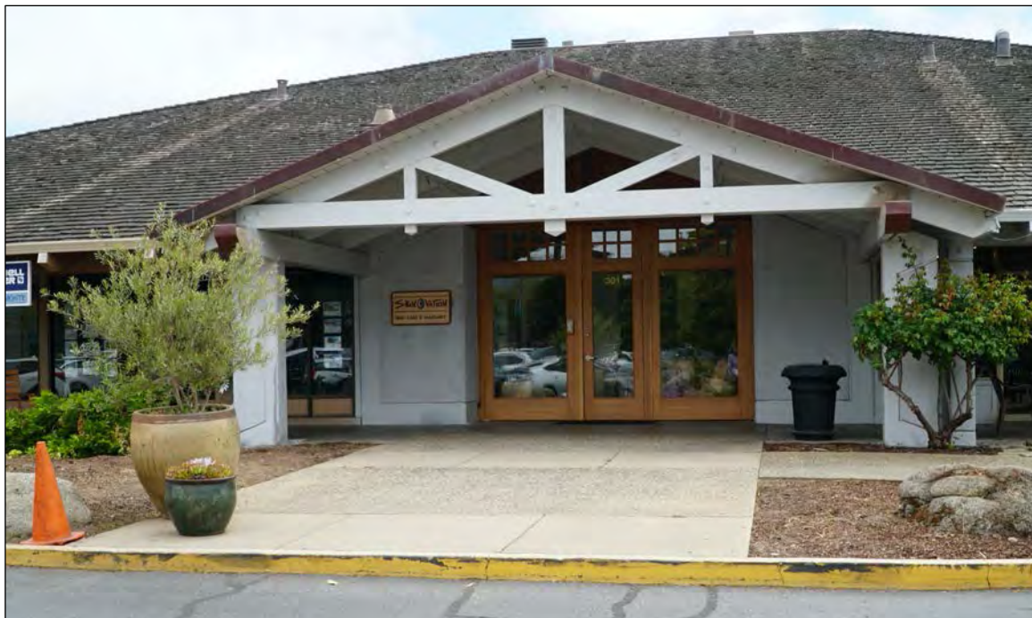
Figure 18. Looking north at section of south side of Building 3, formerly the location of Valley Cinema, 19 August 2019
