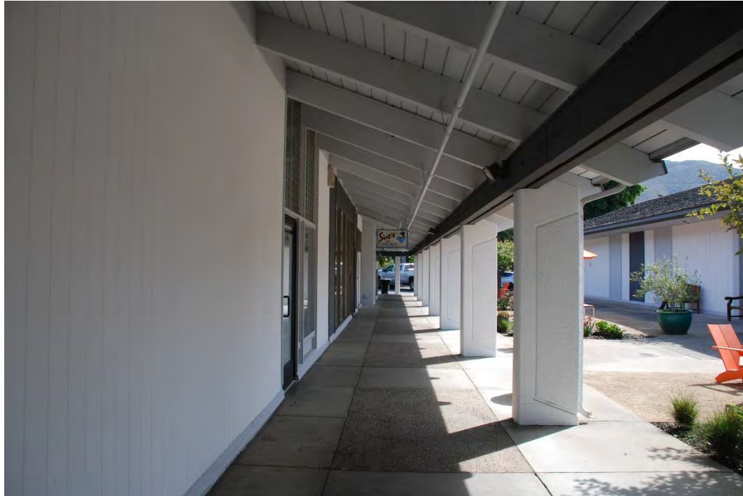
Figure 17. Building C southwest façade, view southeast.
