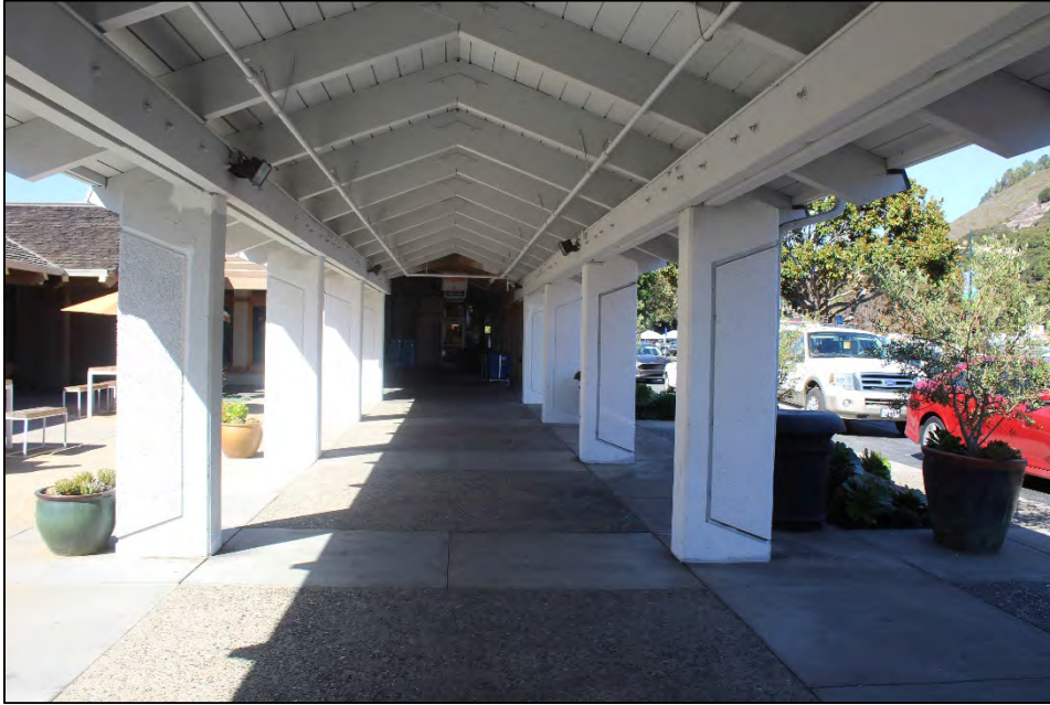
Walkway from Building C to Safeway, looking north
