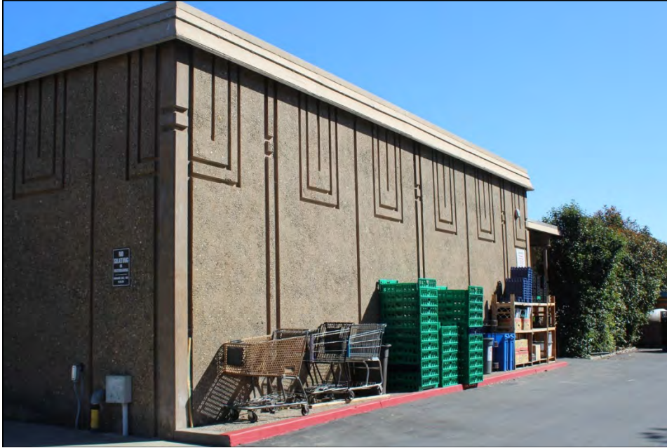
Rear west façade, north end, looking south
