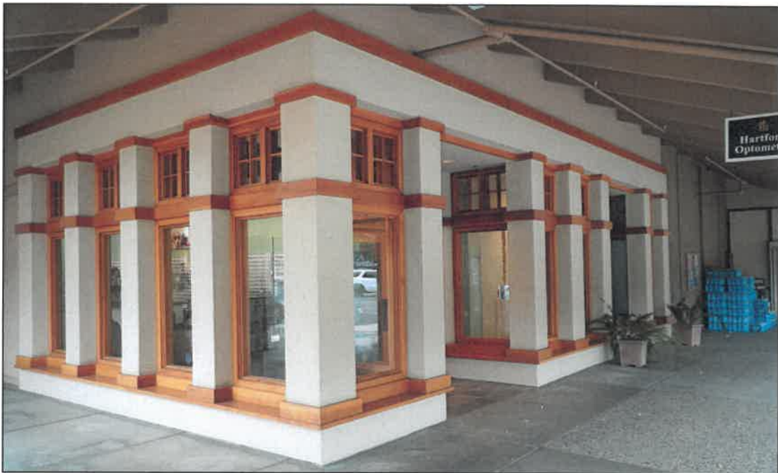
Figure 14. Looking southwest at two shops in Block 1, 19 August 2019. Their original appearance may be seen in Figure 13. The exteriors were radically altered about 1994.
