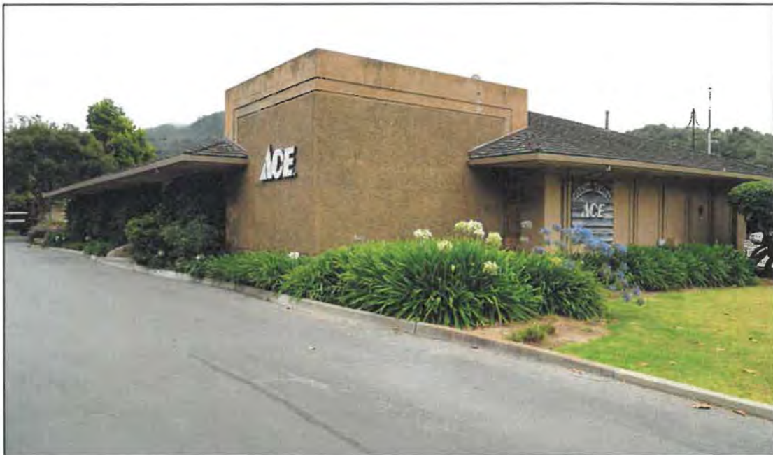
Figure 10. Looking southeast at north and west sides of Block 4, 19 August 2019.
