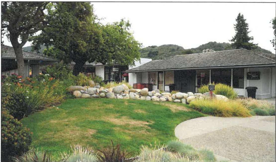
Figure 4. Looking southeast at north side of the 1967 section of Block 2, 19 August 2019.
