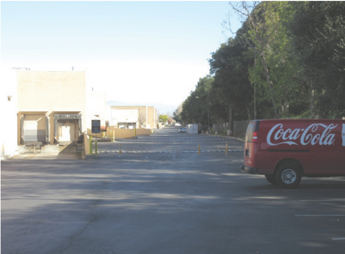
Photo 3: View of access road/alley behind El Paseo building, and screen trees/berm along southern project boundary, facing east.
