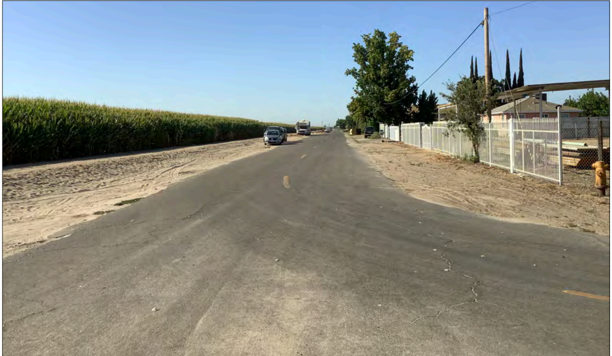
Figure 7. Photograph showing a paved street, disturbed road shoulder, fenced homes, and agricultural land cover.
