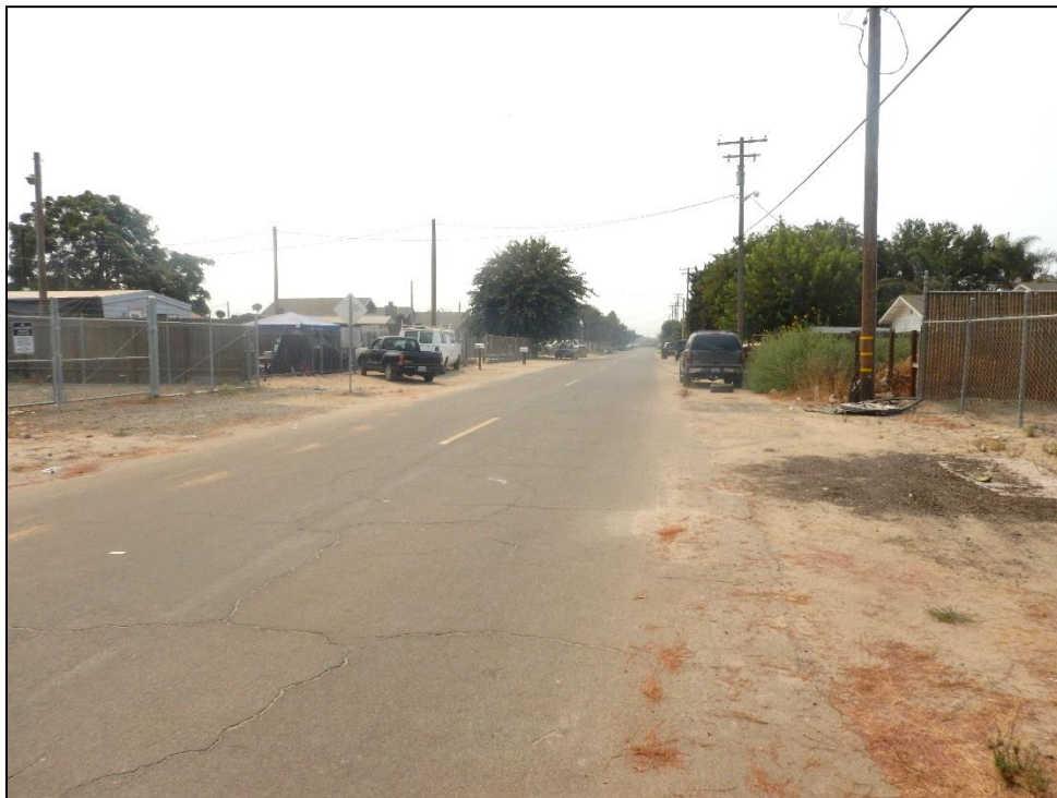
Figure 10. Overview of APE on Monterey Avenue. View west.
