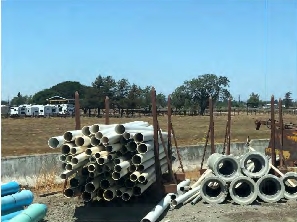
Concrete k-rail prevents CTS from dispersing into stockpile and staging areas on the site.
