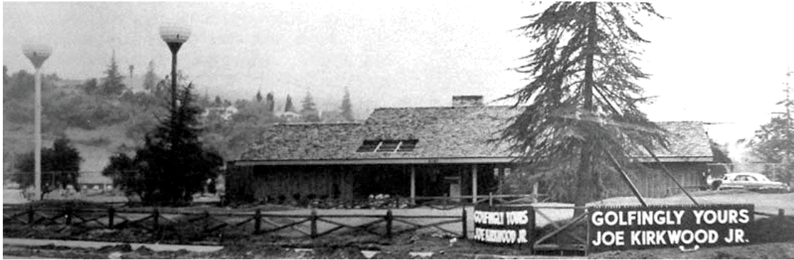
Historic Image 1. East façade of clubhouse, view facing southwest, c. 1956. Source: John Jones, “The Joe Kirkwood Jr Golf Center,” Golf Historical Society, http://golfhistoricalsociety.com/kirkwood/index.html (accessed July 2020).
