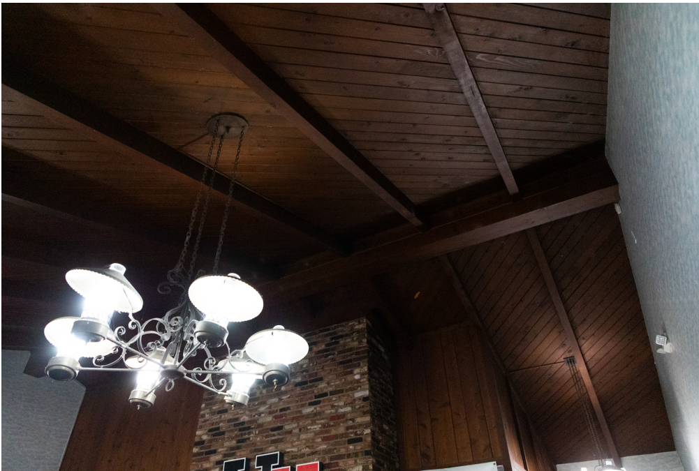
Photo 12. Lobby ceiling and chandelier, view facing southwest.
