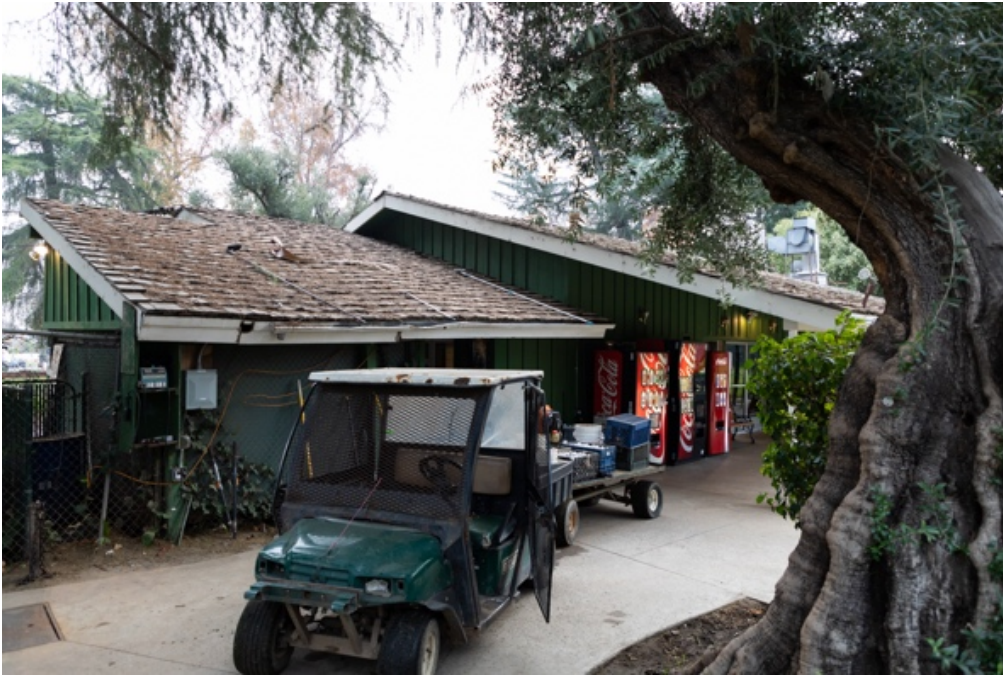
Photo 7. Clubhouse, north and west façades, view facing southeast.
