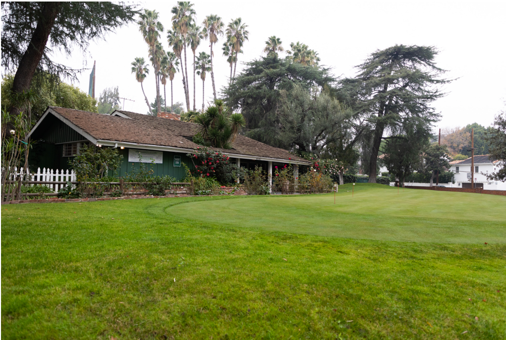
Photo 6. Clubhouse, east (primary) and south façades, view facing northwest.
