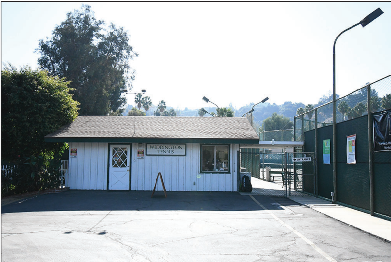
PHOTOGRAPH 3: Existing tennis check-in building. Tennis court fencing is visible in the right of the photograph.
