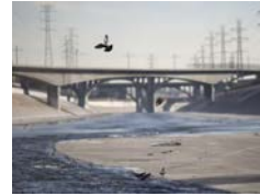
9 views of the LA River before and after it was paved in 1938
