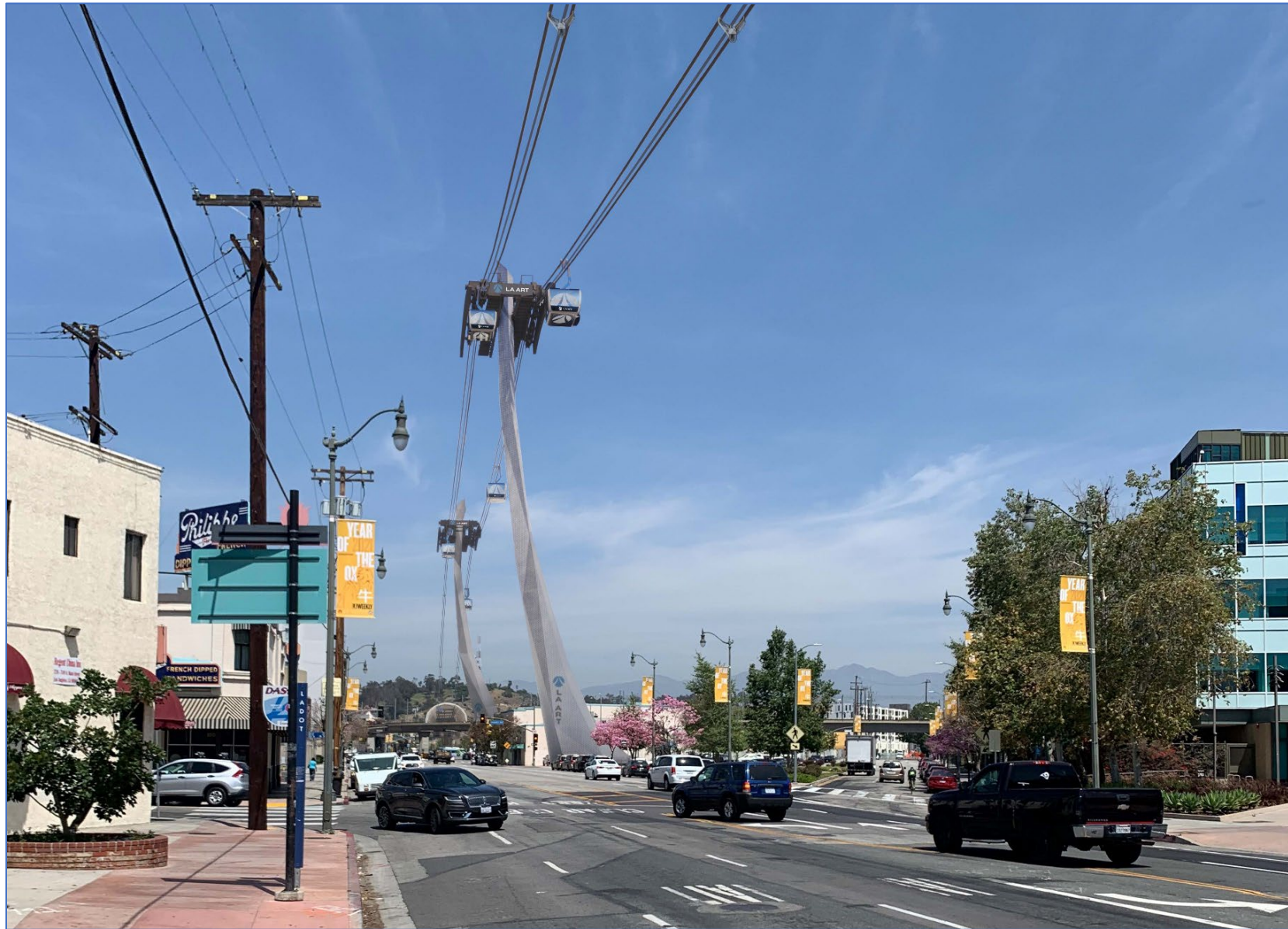
Figure 3-6 2-6: Illustrative Design of a Tower *This illustrative design depicts Alameda Tower in the foreground and Alpine Tower in the middle ground.
