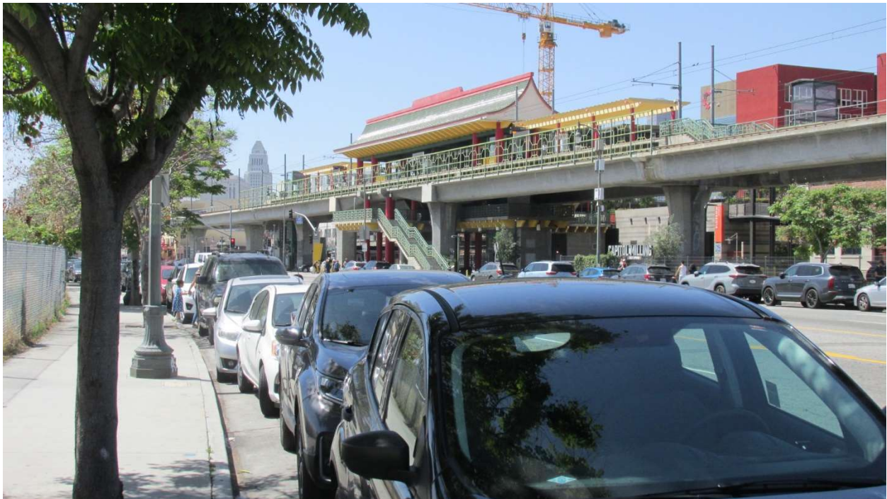
A view of Gold Line Chinatown Station from Spring St.
