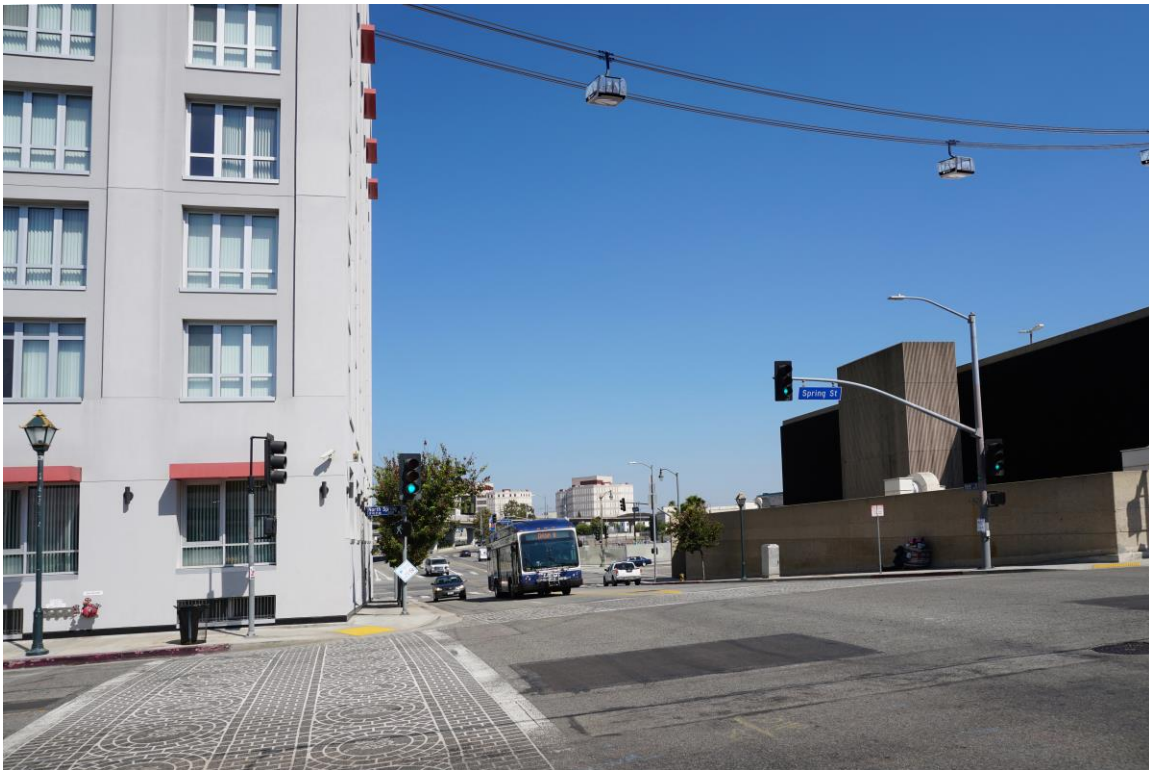
Figure 5-12: Existing and Simulation Views of KOP 11 – Looking East along Alpine Street from Spring Street
