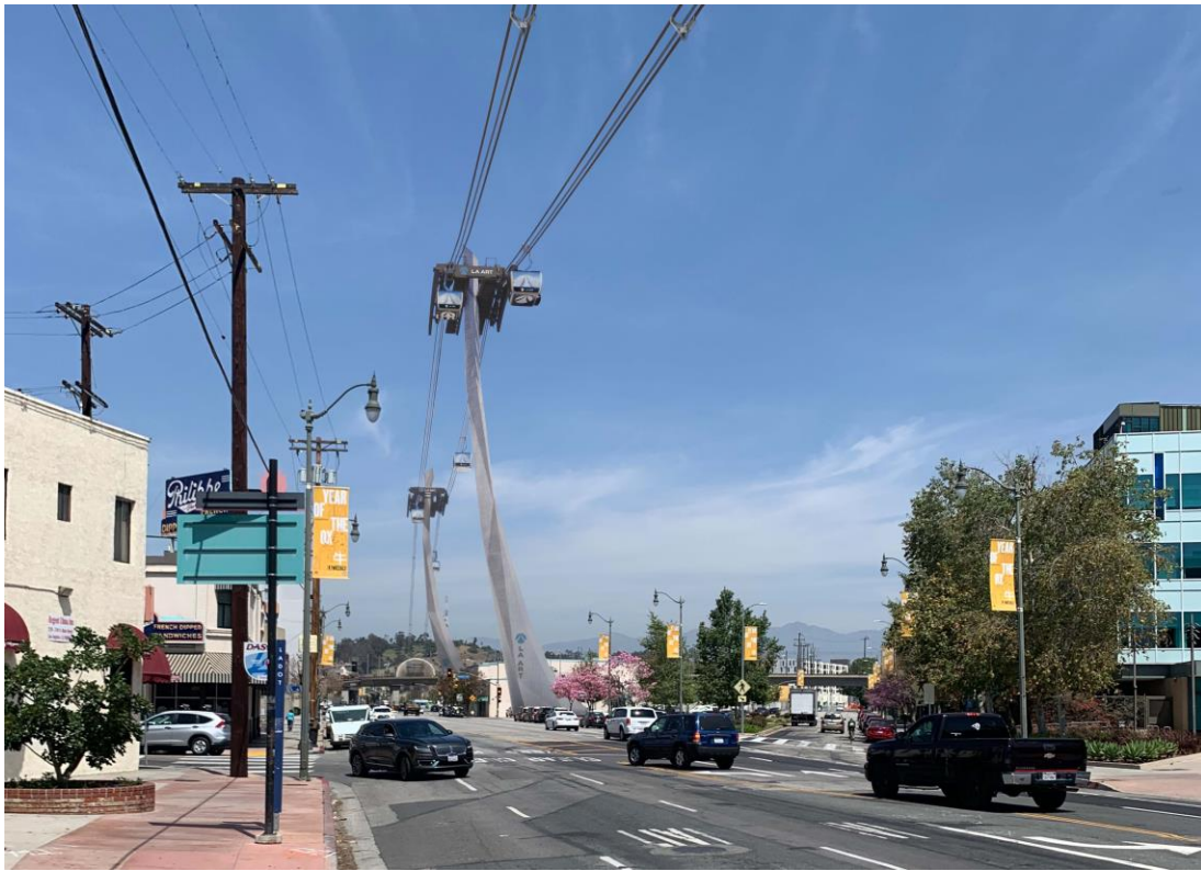
Figure 5-10: Existing and Simulation Views of KOP 9 – Looking North on Alameda Street from Main Street
