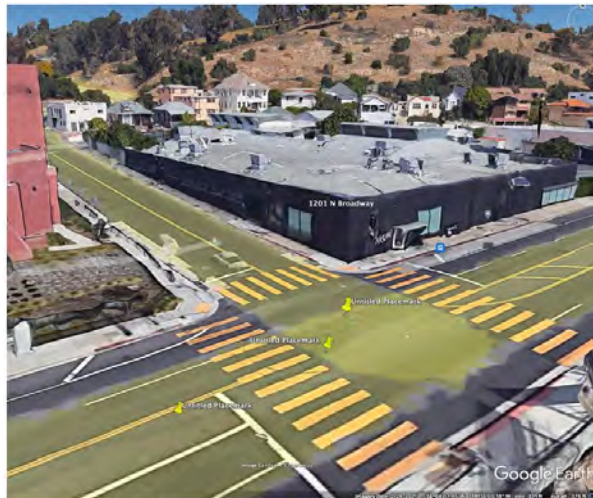
Google Earth View of Broadway Junction Site, view from 45 ft above ground
