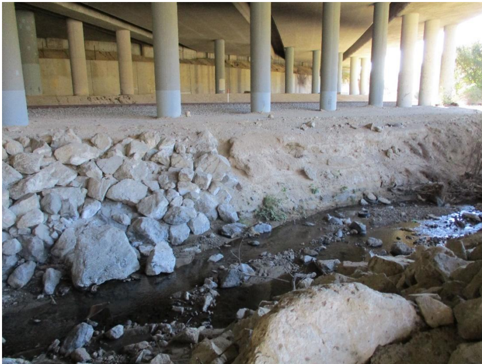
Figure 11: Exposed Pico Formation, sandstone (Tps) beneath the I-5 overpass in the Balboa Double Track Extension area. View southeast.
