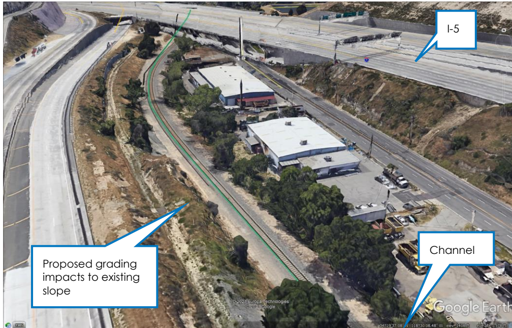
Figure 22: Balboa Double Track Extension site downstream view
