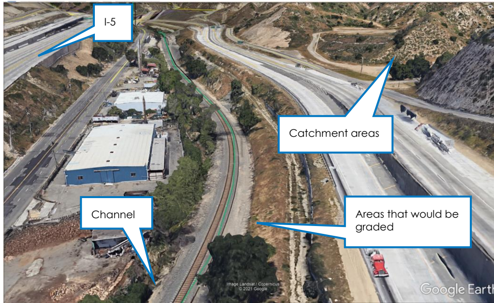
Figure 21: Balboa Double Track Extension site upstream view
