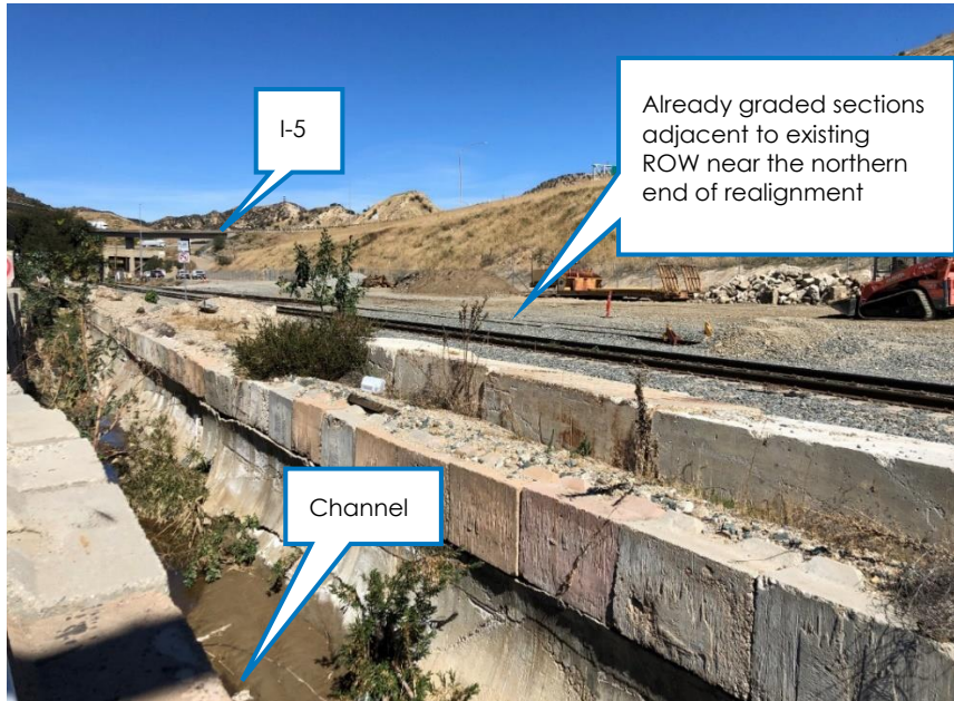
Figure 20: Balboa Double Track Extension site downstream view
