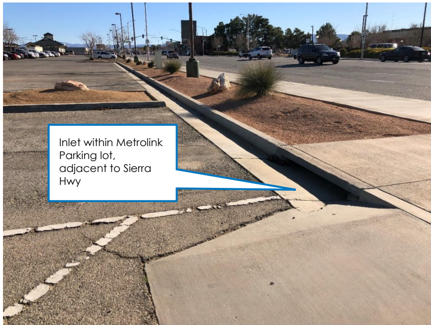
Figure 17: Lancaster Terminal Improvements site - inlet
