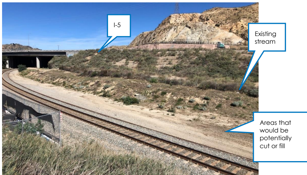
Figure 19: Balboa Double Track Extension site upstream view
