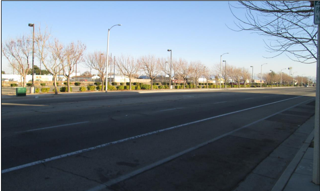
Figure 3.2-8: Key View 7 – Sierra Highway Looking Southeast
