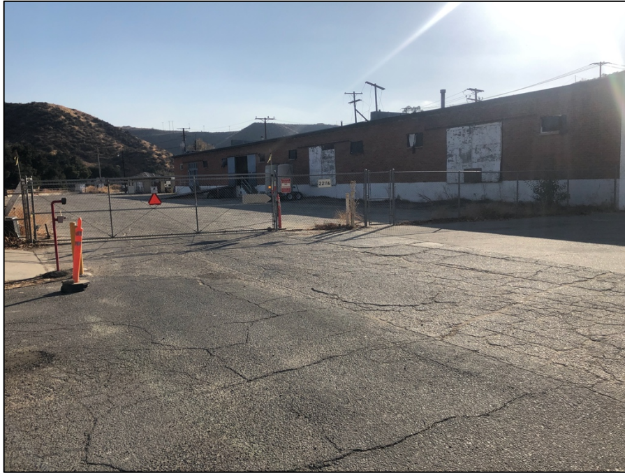
Photograph 5 – Central Portion of the Canyon Siding Extension Project Area. View to the South.
