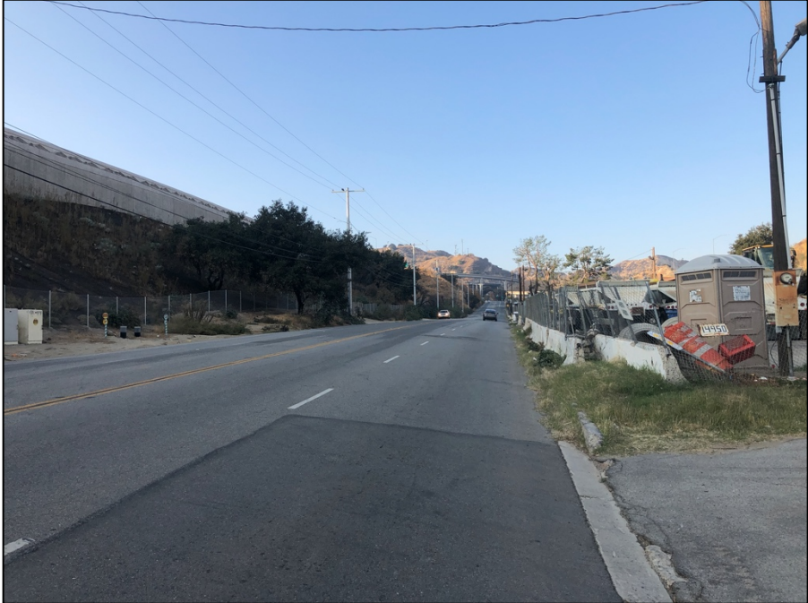
Photograph 8 – Central Portion of the Balboa Boulevard Project Area. View to the Northwest.
