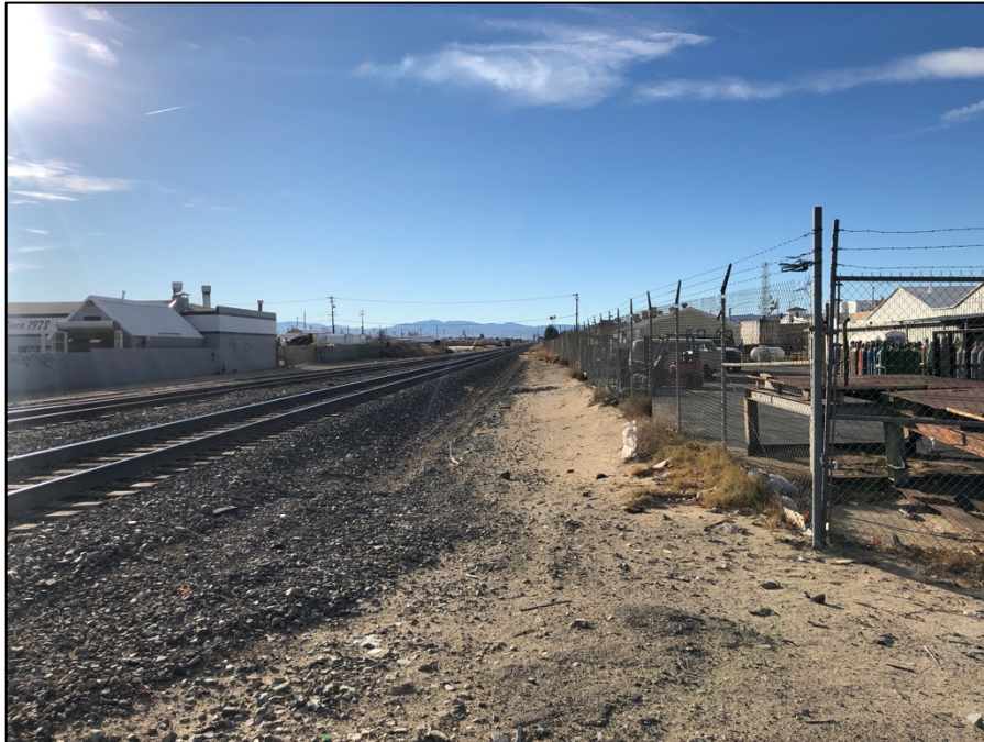
Photograph 1 – Northern Extent of the Lancaster Terminal Project Area at Avenue I. View to the South.
