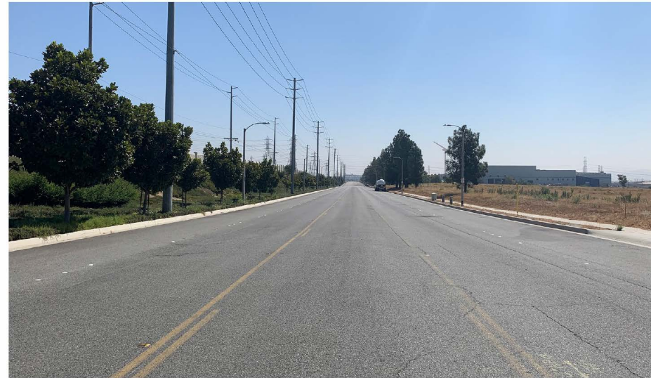
View 2: Looking east along 6th Street with the Project site visible in the right portion of the image
