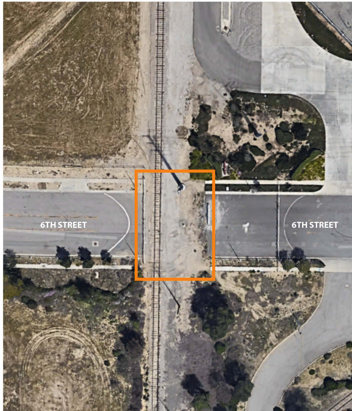
6TH STREET CROSSING - EXISTING CONDITION
