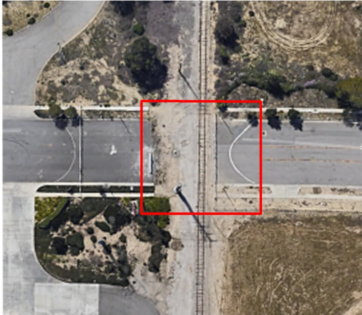
6th Street Crossing - Existing Condition
