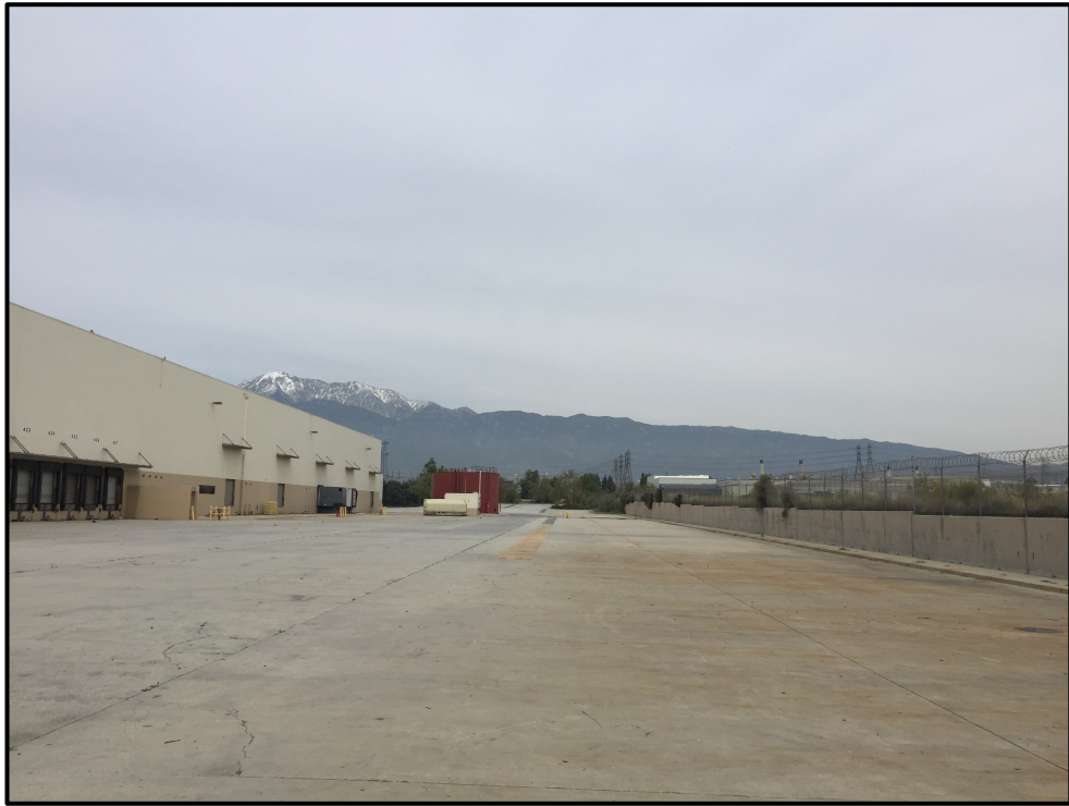
Plate 4.2-2: Overview of the warehouse/distribution facility within the subject property, facing north.
