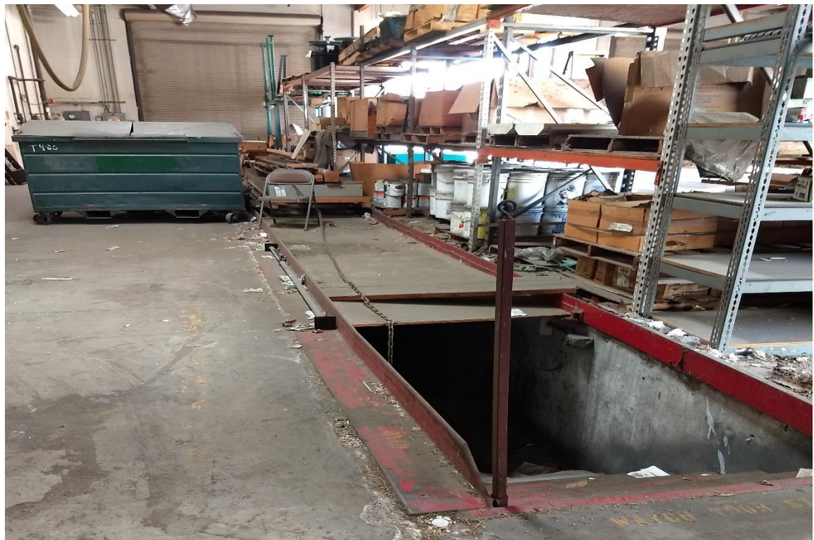
Photograph No. 4: Maintenance Pit located within the Former Truck Maintenance Area.
