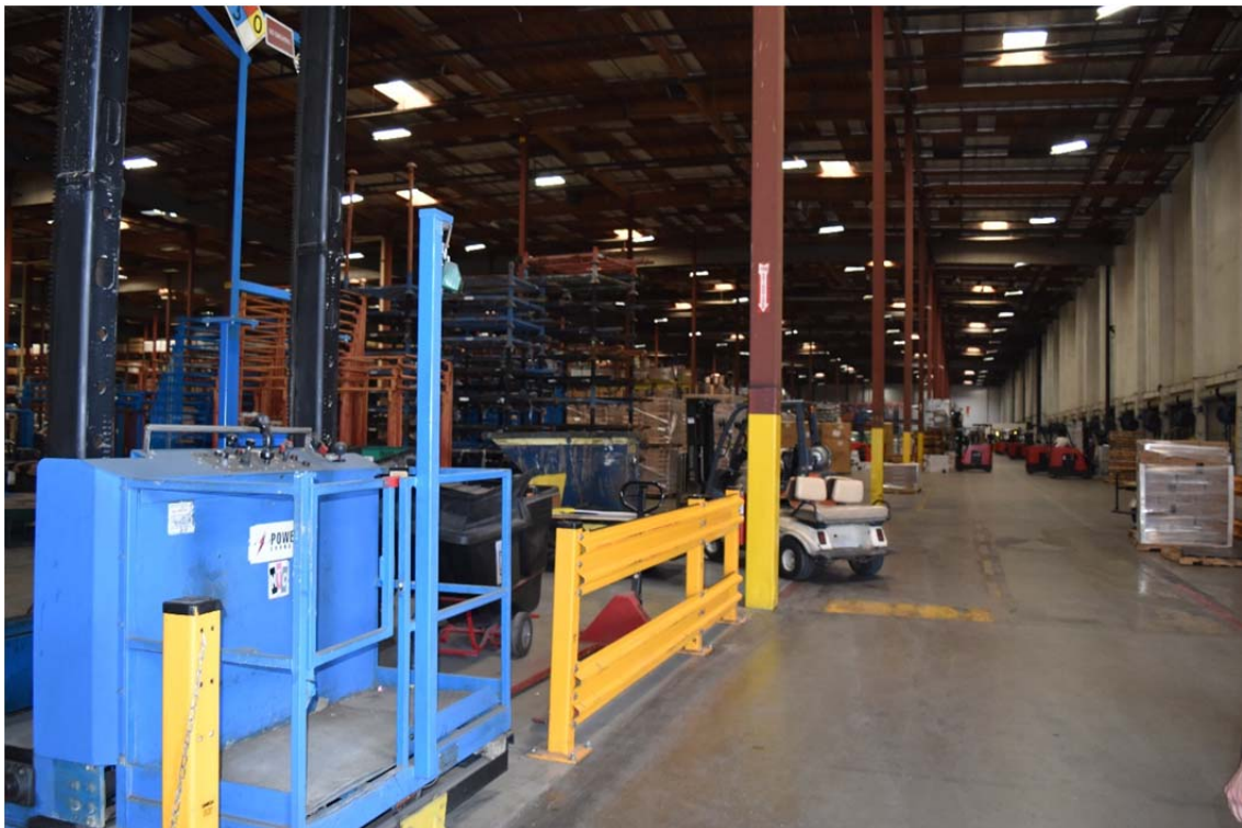
18. Warehousing operations and storage area for batteries to recharge equipment used at the Site located inside the southeastern portion of the structure.
