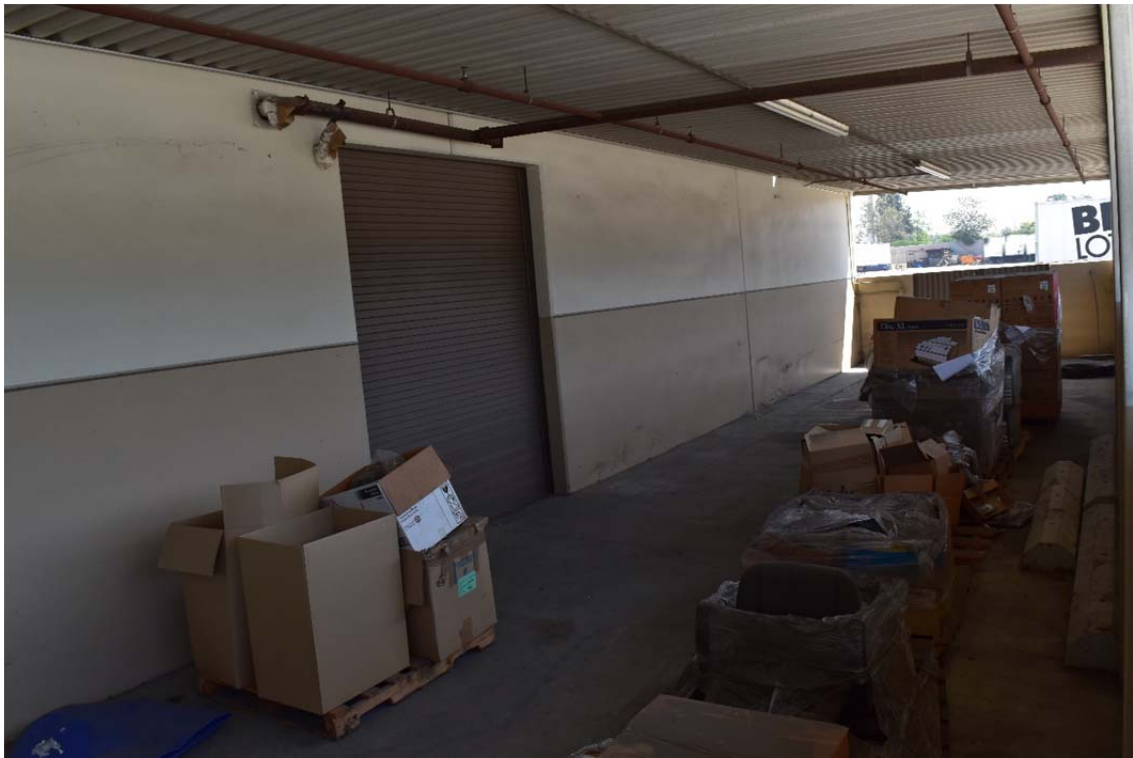
43. Former underground storage tank and storage area outside to the south of the former maintenance structure located in the southwestern portion of the Site.
