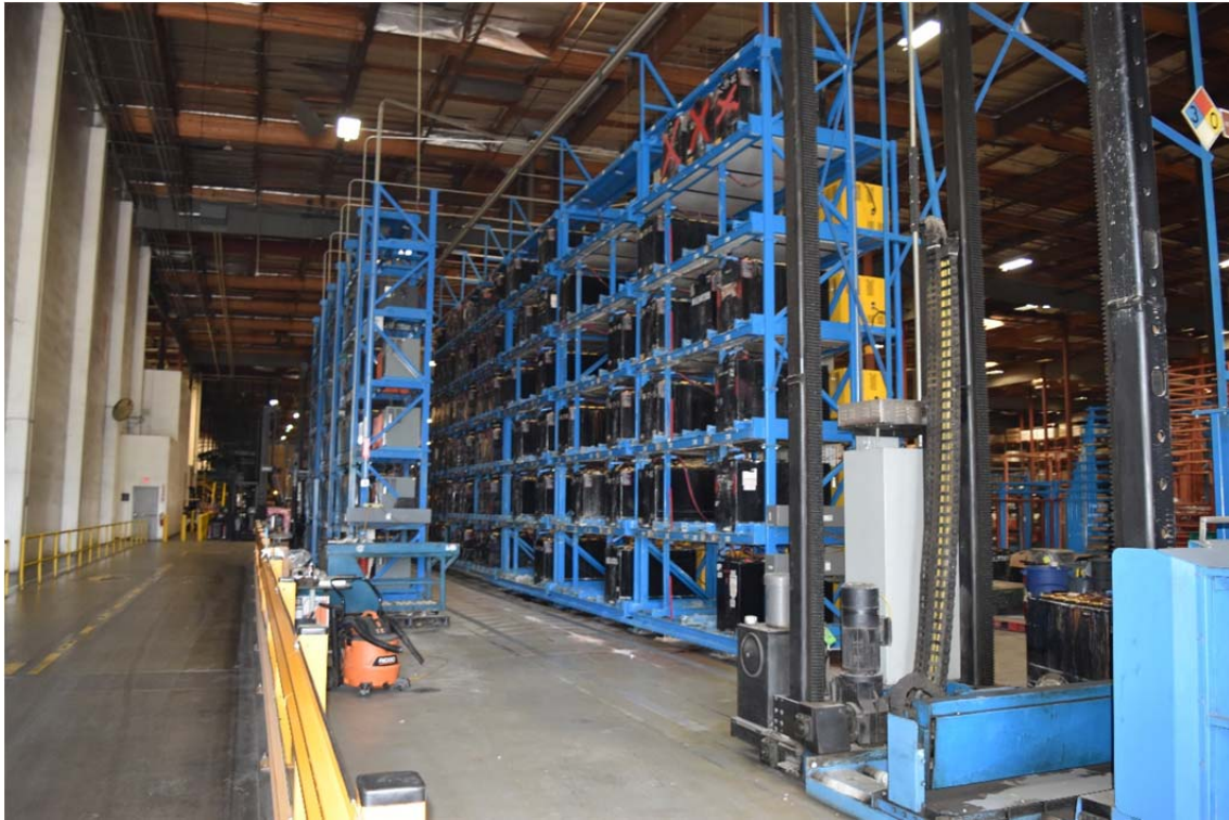
17. Storage area for batteries to recharge equipment used at the Site located inside the southeastern portion of the structure.
