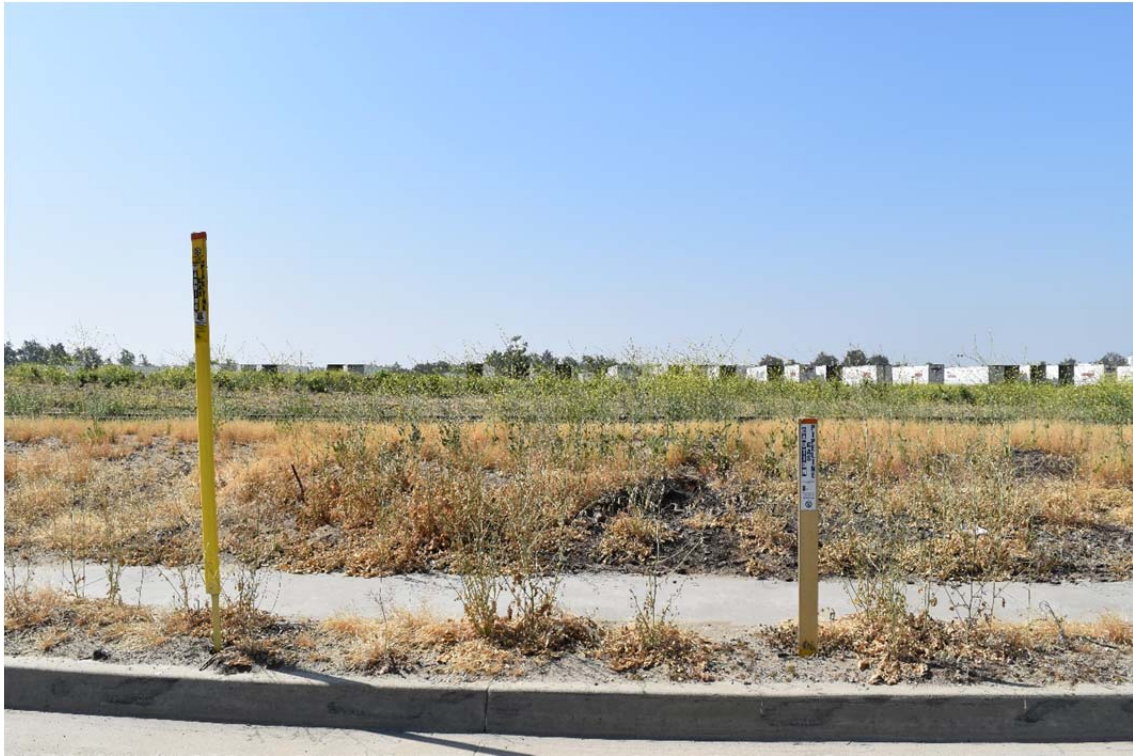
5. High pressure gas line beneath the sidewalk along the northern perimeter of the Site – view facing south.
