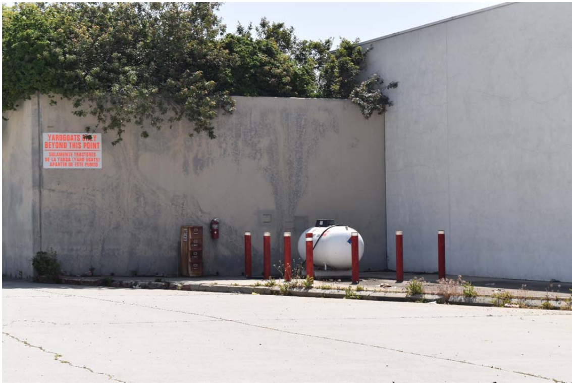
47. Propane tank storage area located to the north of the Big Lots retail store and south of the former automobile maintenance building – view facing southeast.
