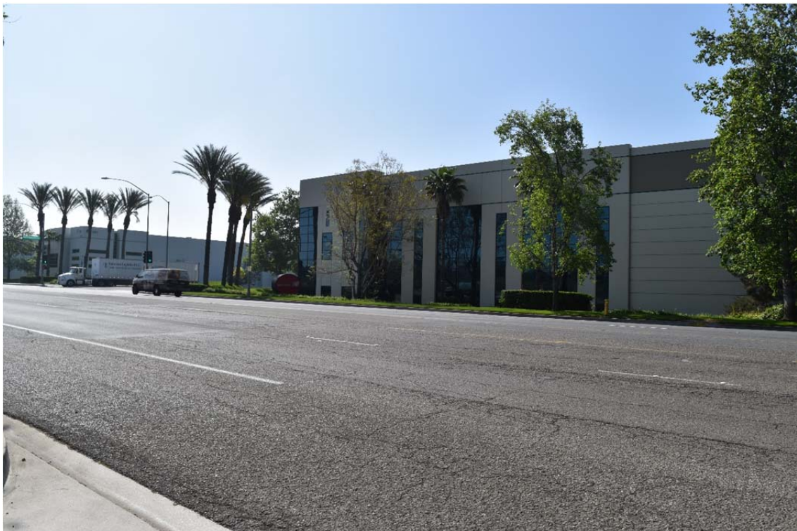
62. Fourth Street followed by warehousing operations to the south of the Site – view facing southeast.
