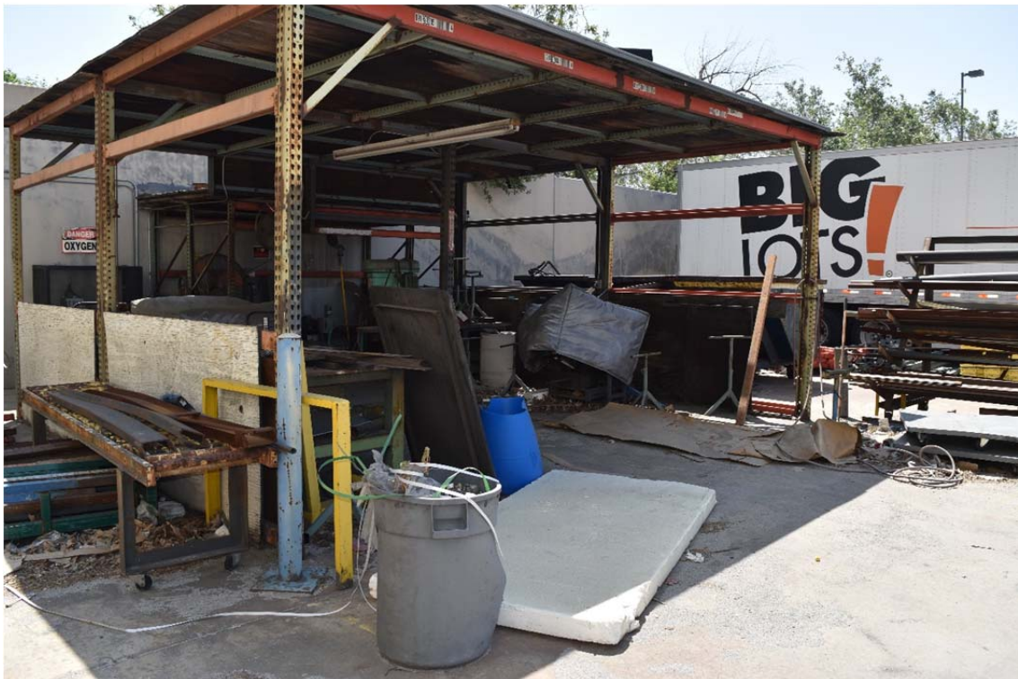
50. Storage area located to the east of the former automobile maintenance area and south of the warehouse structure.
