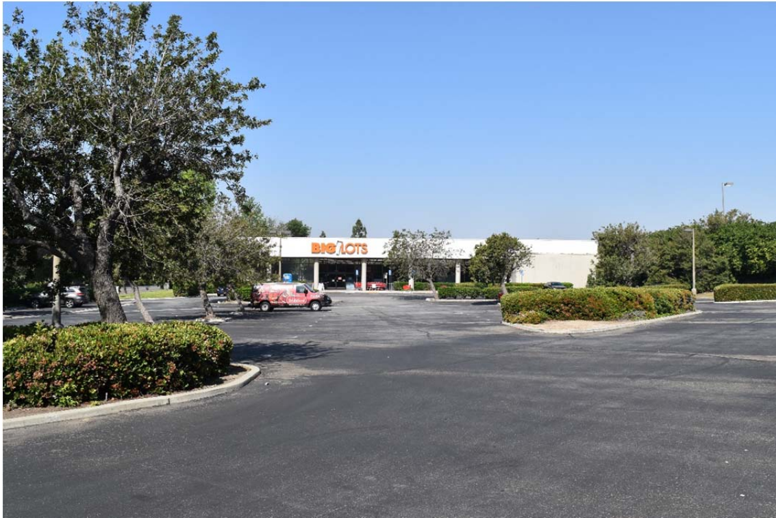
57. Big Lots retail structure and paved surface parking lot on the southwestern portion of the Site – view facing west.
