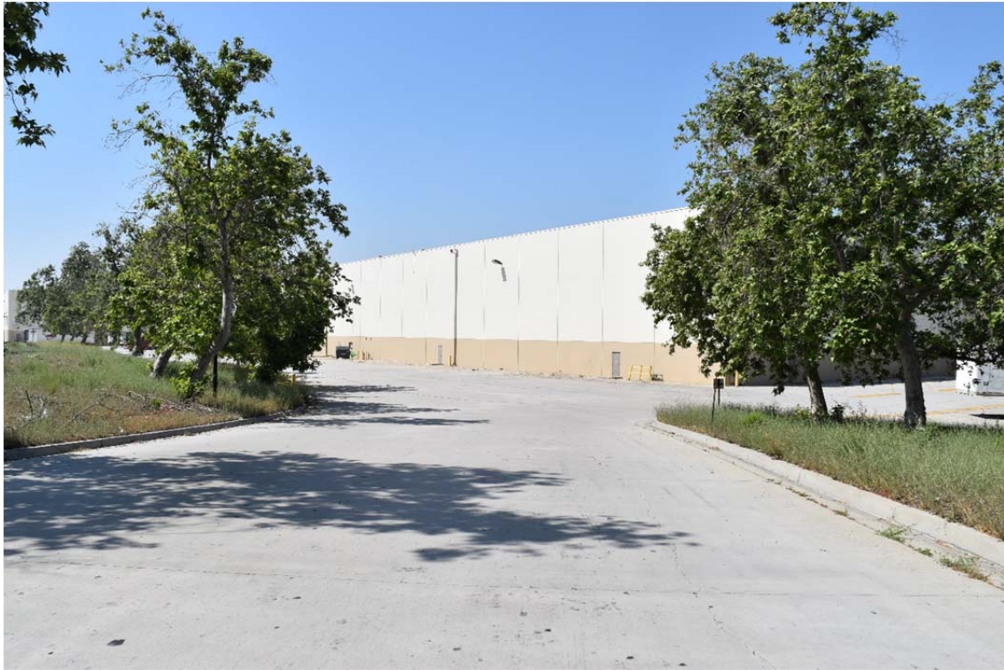
11. Driveway from the parking lots to the warehouse structure in the central portion of the Site – view facing southwest.
