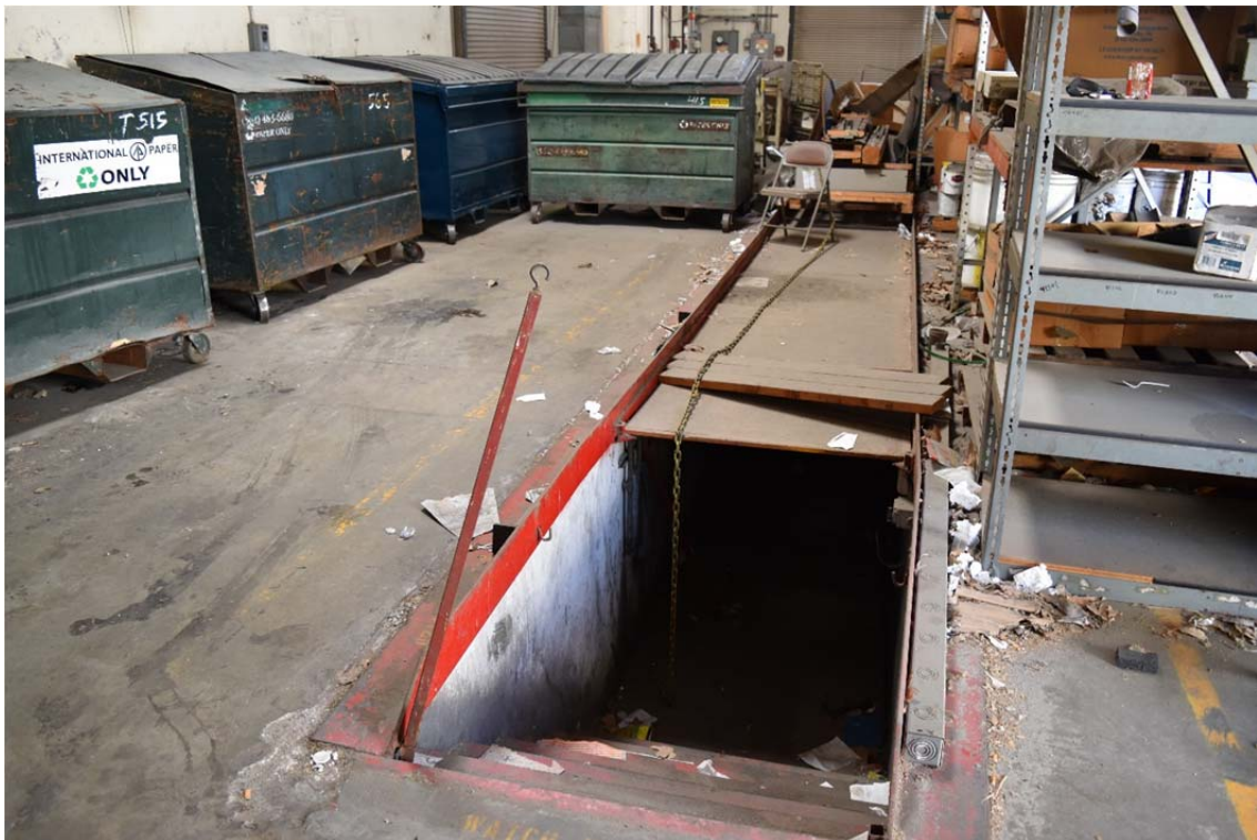
42. Former automobile maintenance vault in the former maintenance building.
