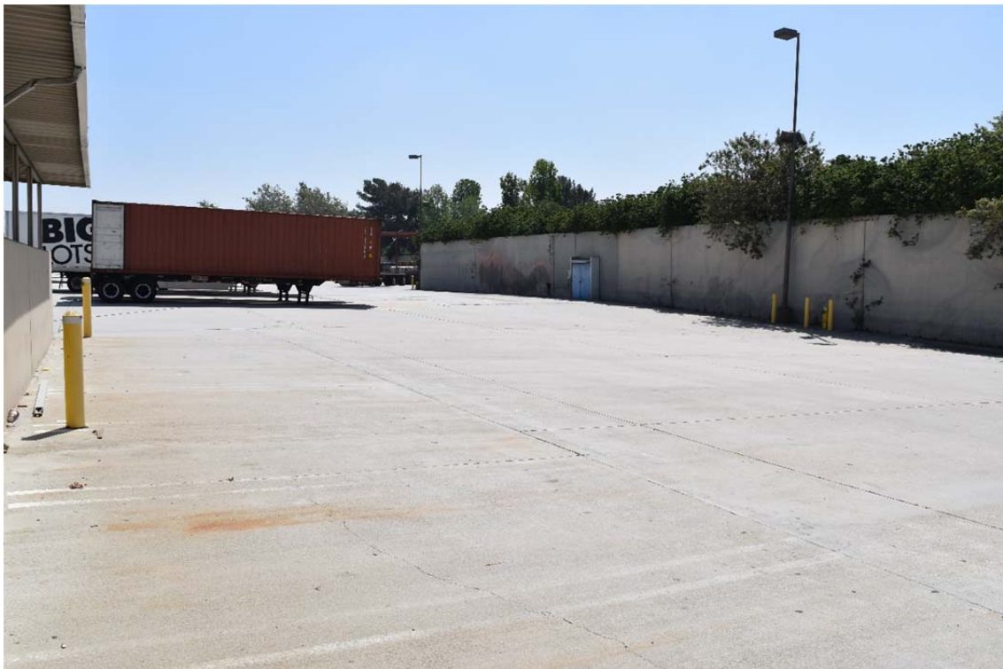
44. Former underground storage tank area outside to the south of the former maintenance structure located in the southwestern portion of the Site.
