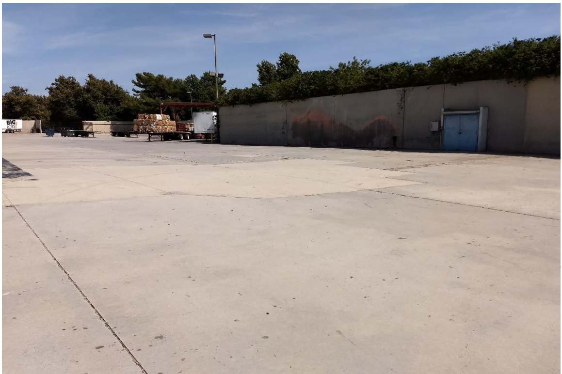
Photograph No. 6: Location of former fuel underground storage tanks (USTs), looking southeast.
