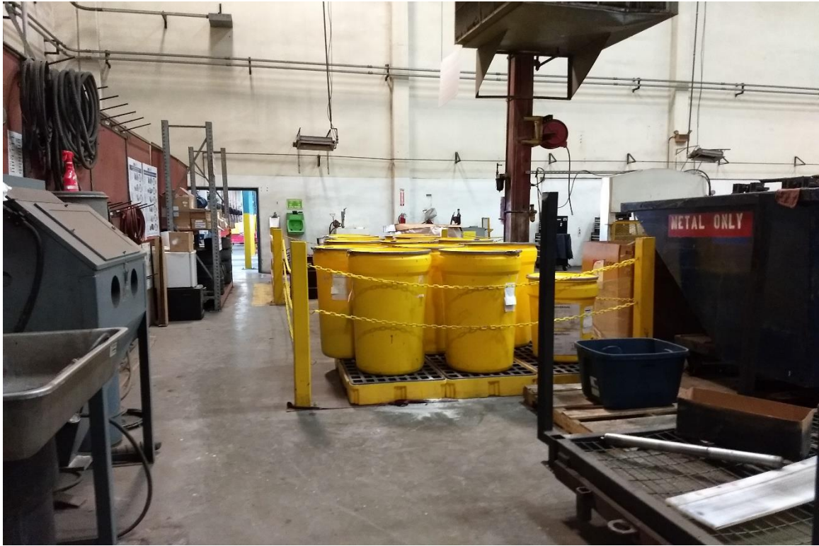
Photograph No. 13: Hazardous Waste Storage Area in the Forklift Maintenance Area.
