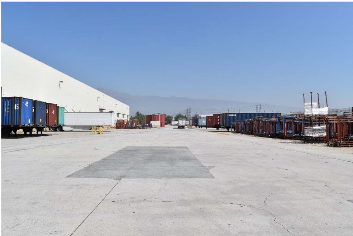
12. Shipping, receiving, transport, and warehousing operations at the structure in the central portion of the Site.
