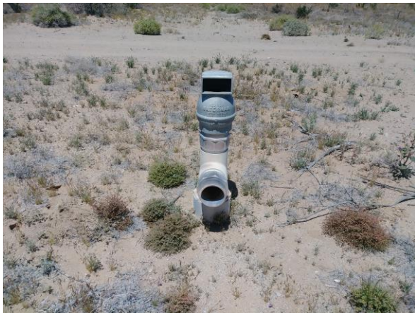
Photo #15 Irrigation piping air-release valve located along the western boundary of the northern tract.
