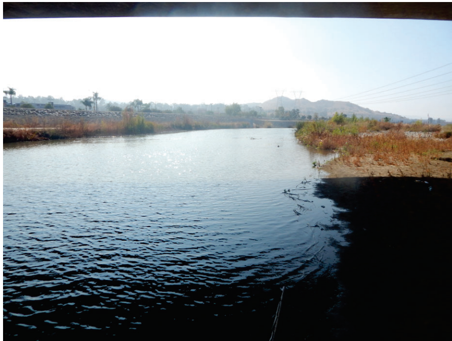
View of the Santa Ana River looking west from beneath the Yorba Linda Boulevard bridge. November 7, 2019.
