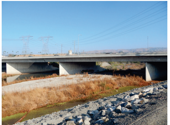
View of waters and wetland areas looking north toward the downstream side of the Yorba Linda Boulevard bridge. November 7, 2019.
