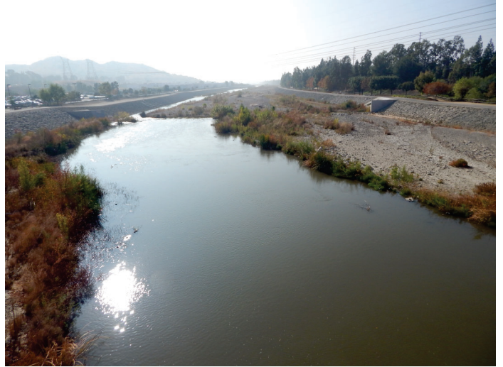
View of the Santa Ana River looking west from the Yorba Linda Boulevard bridge. November 7, 2019.
