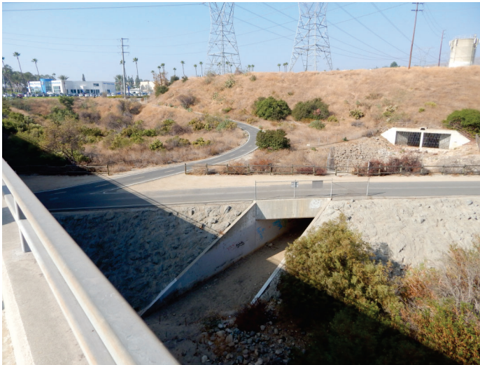
View of the tributary looking north from the Yorba Linda Boulevard bridge. November 7, 2019.
