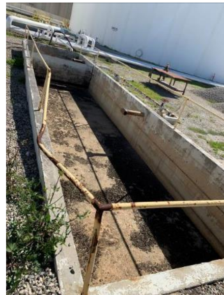
Figure 2-5. Oil/Water Concrete Separator Sump (to be demolished)
