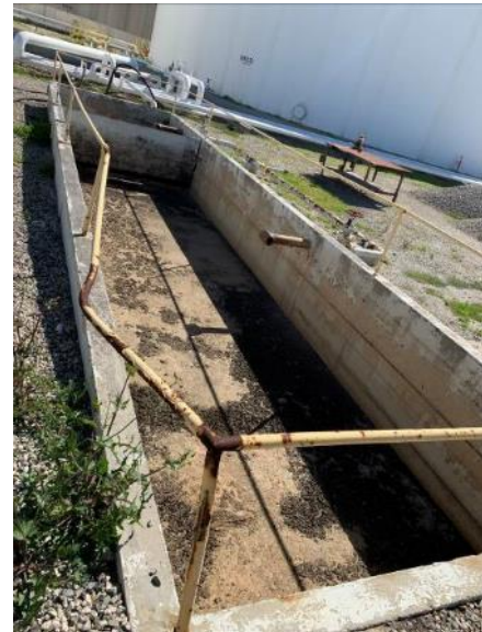
Figure 2-5. Oil/Water Concrete Separator Sump (to be demolished)
