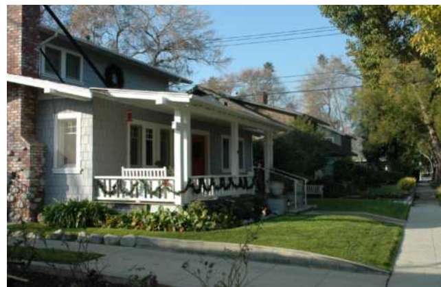
A Projecting Porch on the front creates a space for seating and a platform for decor.
