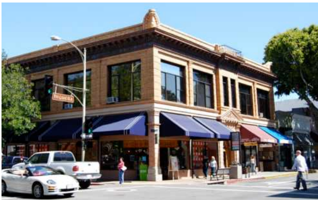
Two-story Main Street building with tall ground floors.
