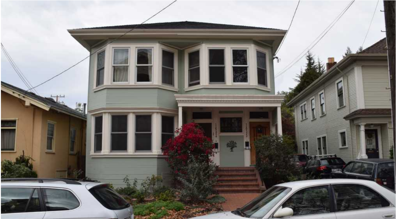
Two-story Duplex with engaged porch.
