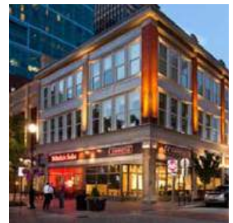
Figure 3.30 Adaptive Reuse Renovation and adaptive use of historic buildings is sustainable, and preserves a sense of history.
