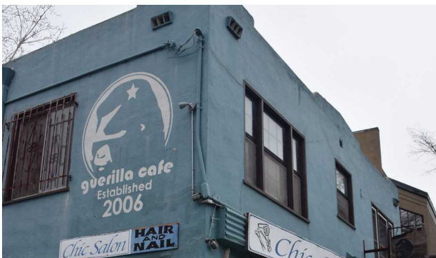
Example of Wall Mural Sign at a second story.
