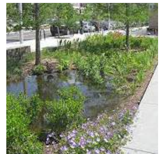
Figure 3.23 Rain Gardens Rain gardens for treating stormwater runoff integrated into streetscape design.
