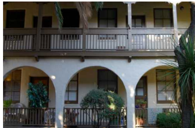
A two-story Gallery fronting a passage.
