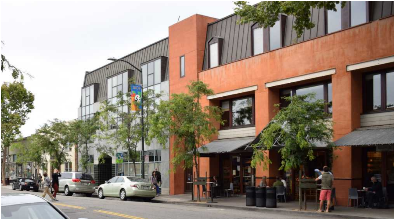
Three-story Main Street building forms a contemporary streetscape with variation.
