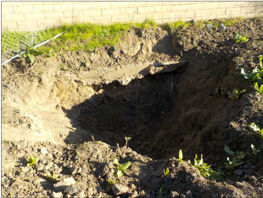
Photo 5. Excavated pit and wall footing, looking east.
