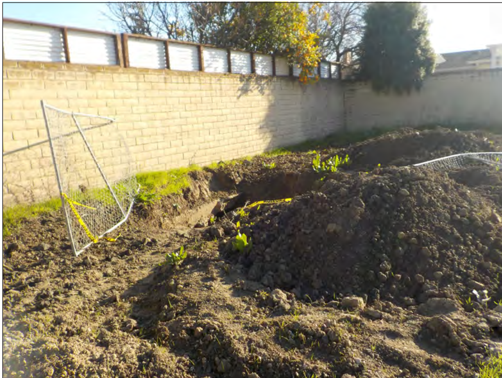
Photo 6. Excavated pit and chain link fence, looking southeast.
