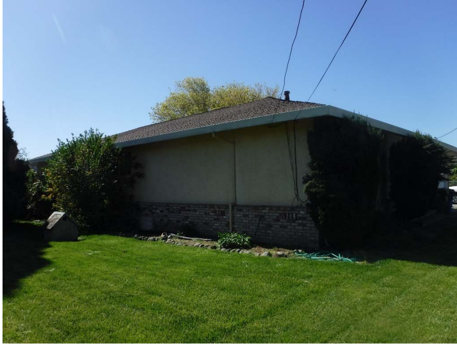
Photo 15: Occupied residence in the northern portion of the Subject Property.
