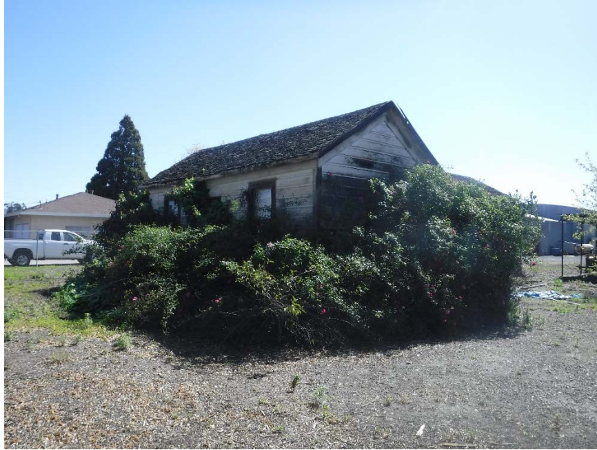
Photo 7: Front of abandoned residence shown in Photo 6.
