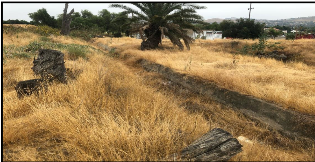
Figure 19. Remnant of Lateral No. 3. View from northeastern corner of property, facing west. Photo, Caius Chickanis.
