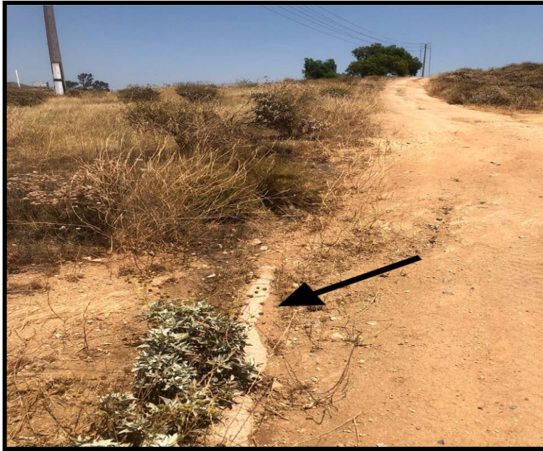
Figure 22. View from northeastern corner of property, facing west. Sections of Lateral No. 3 were buried. Photo, Caius Chickanis.
