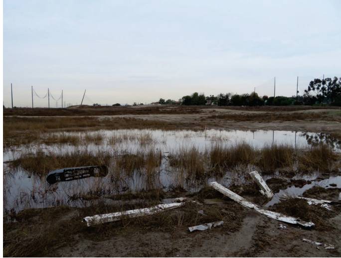
Photo 5: View looking northwest. The site has standing water from a recent storm event.
