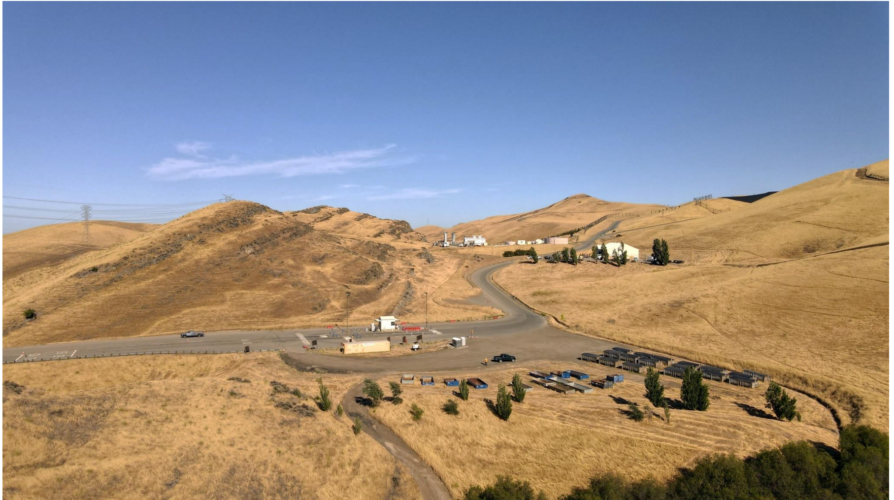
Figure 1-6 Existing bird's-eye aerial view of project site from Vantage Point #4
