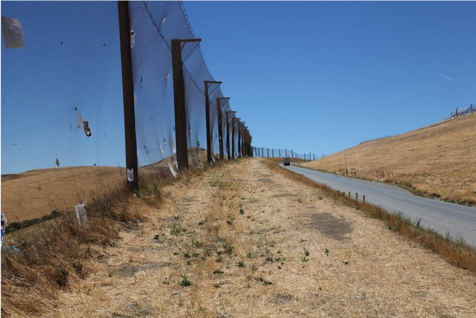
Figure 12 Pipeline Alignment Along Litter Fence Looking East
