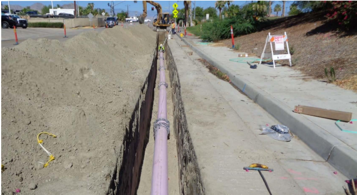
Figure 4 Typical Non-Potable Water Pipeline Trenching Work Site
