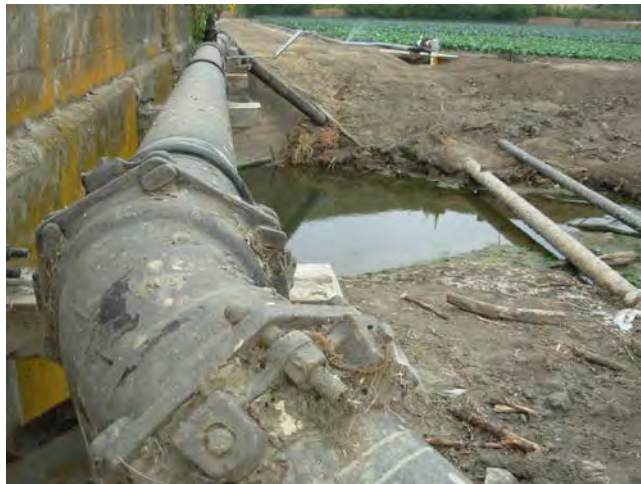
Photo 5 – Iron pipe attached to north side of bridge span
