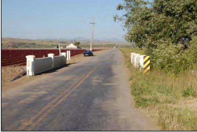
Photo 5. Developed habitat in the BSA includes the existing roadway and bridge.
