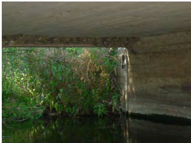
Photo 3 – West abutment and span
