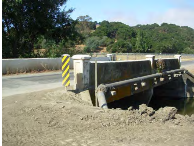
Photo 1 – Anzar Road Bridge (43C-0039) at San Juan Creek, Post Mile 3.86 in San Benito County, California
