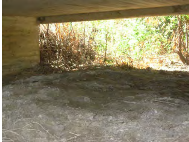
Photo 4 – East abutment and span
