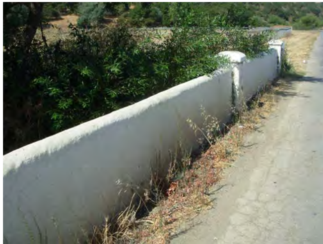
Photo 2 – Bridge deck and barriers
